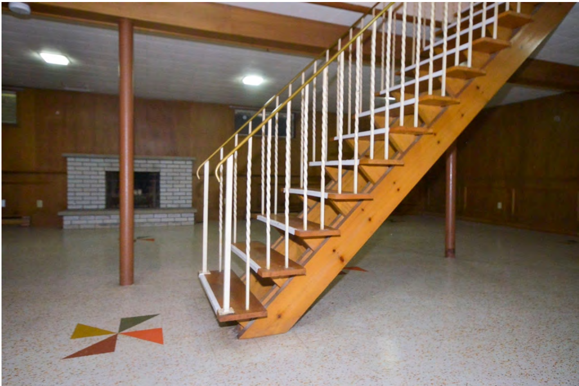
Fig. 48 Floating staircase in basement
