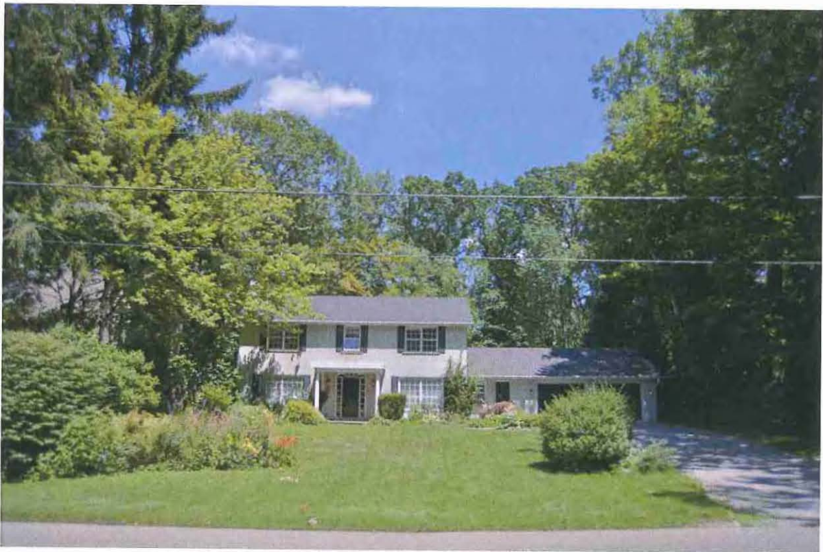
Fig. 1 Front yard and front facade, 1285 Minaki Road
