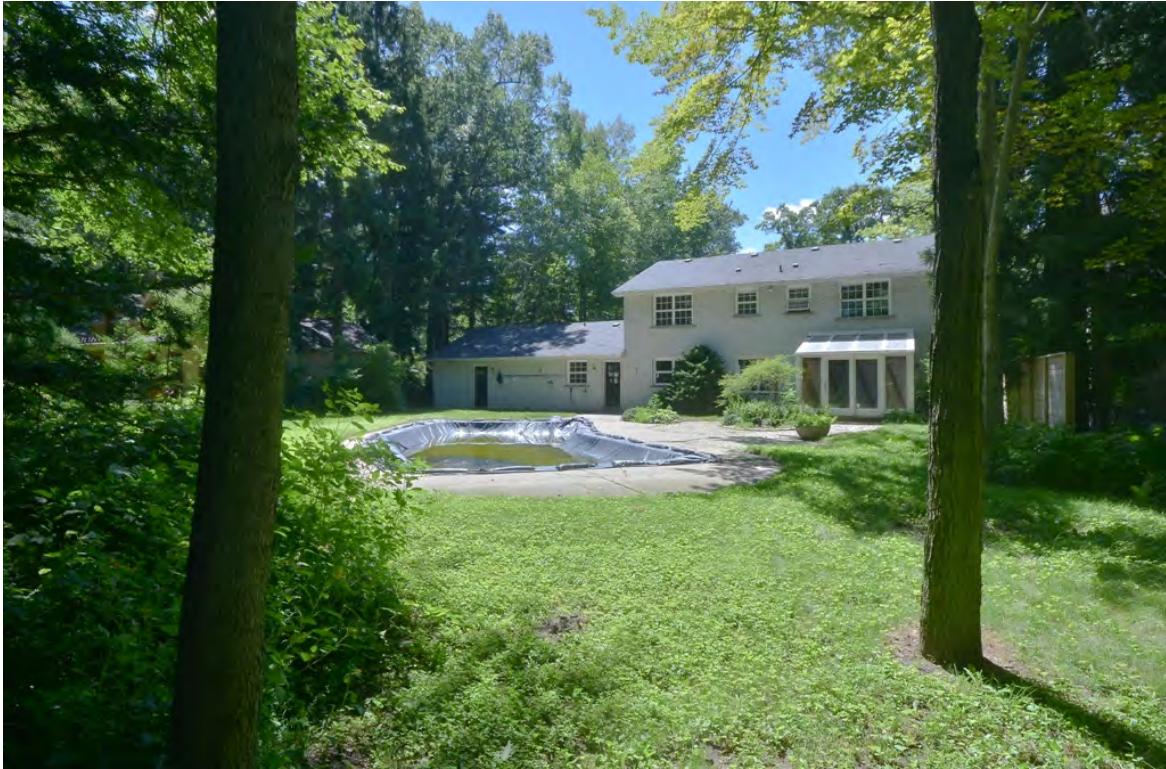
Fig. 6 Backyard as seen from the northeast corner of the lot
