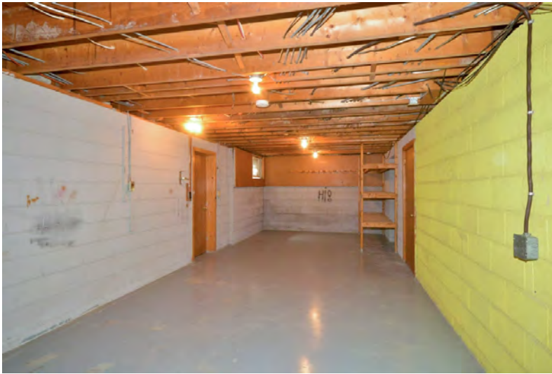
Fig. 49 Unfinished room in basement
