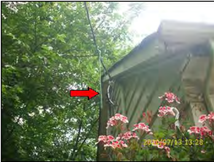
15. Rope attached to service wires.
