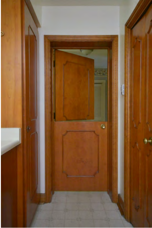
Fig. 42 Dutch door in kitchen
