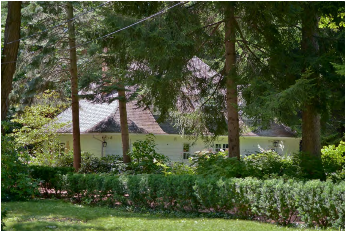
Fig. 11 1290 Minaki Road, on the west side of the street
