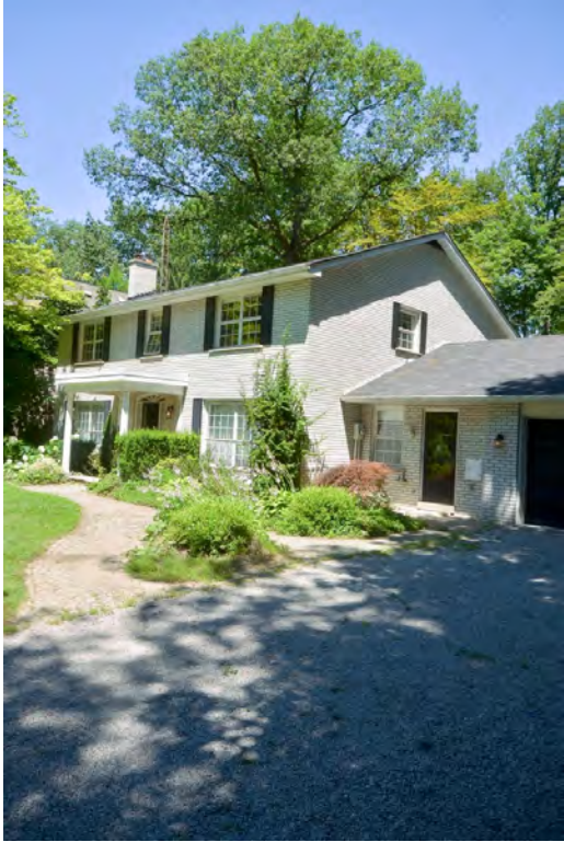
Fig. 24 Corner view, showing front facade and south gable end
