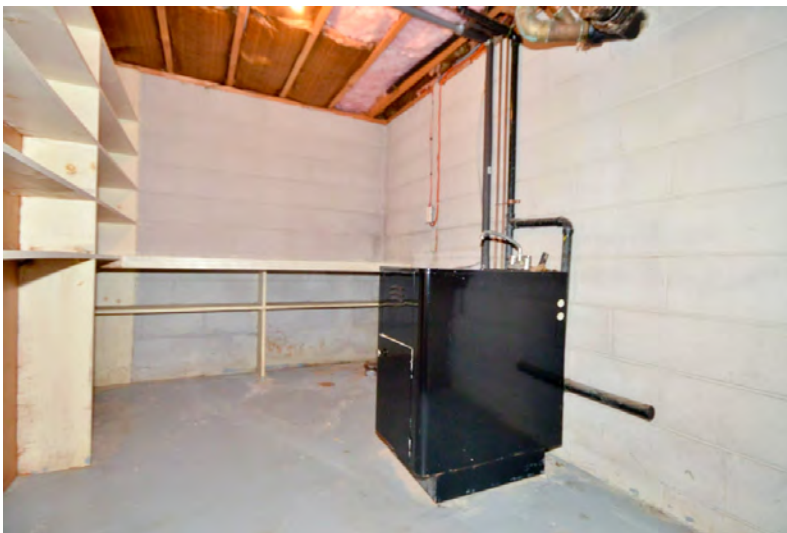
Fig. 50 Laundry room in basement
