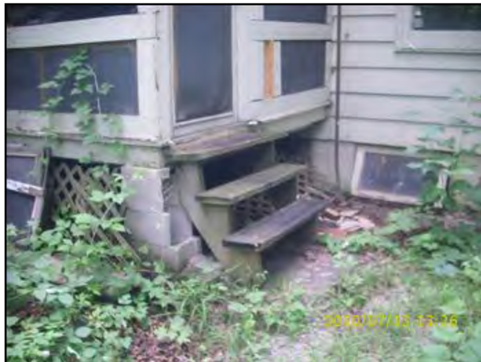
14. Rear porch steps
