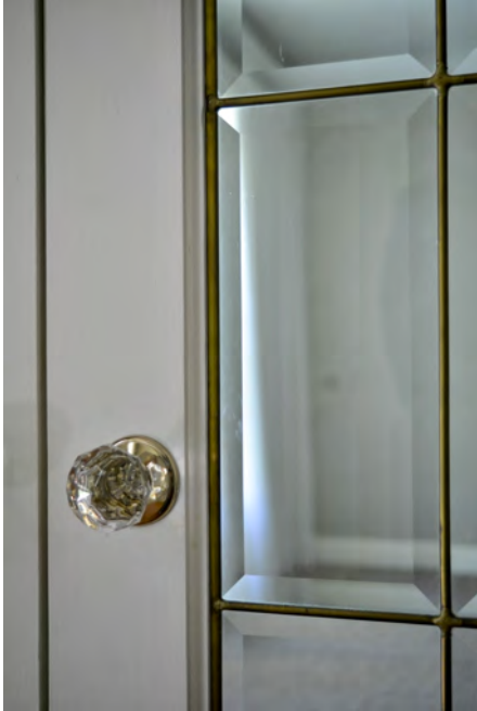
Fig. 32 Detail of glazed door in Fig. 31 (note leaded and bevelled glass and faceted glass door knob)
