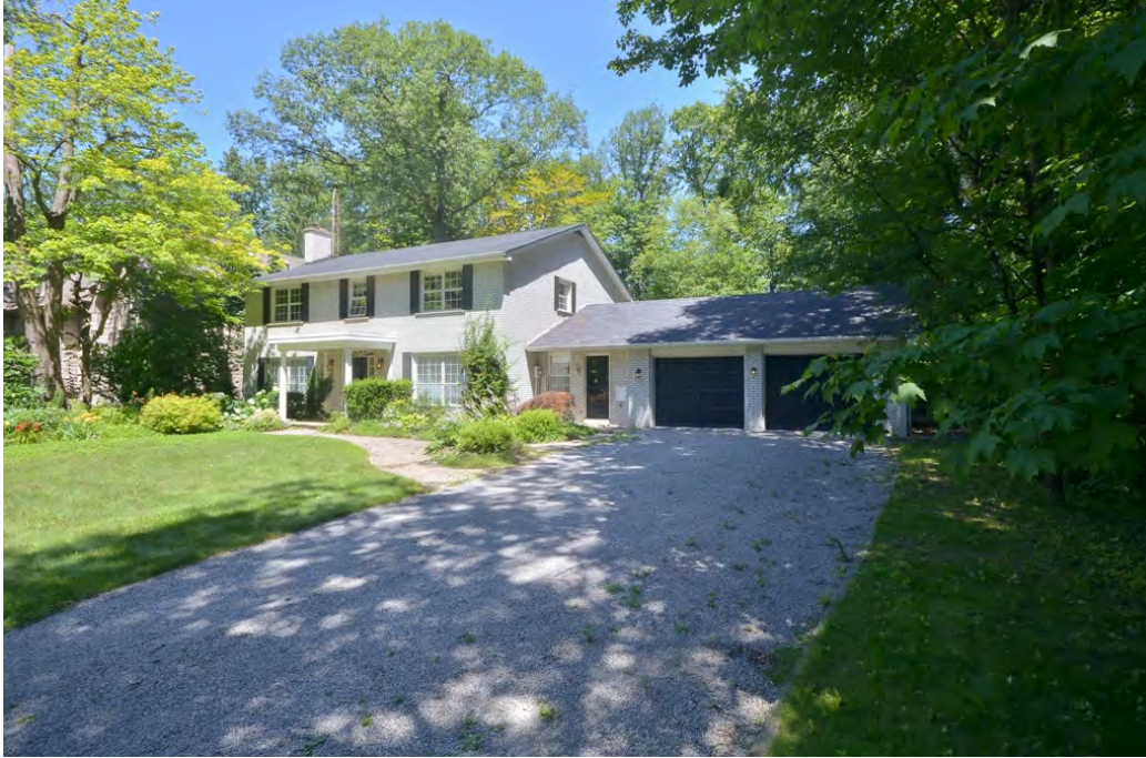
Fig. 4 Front yard, showing gravel driveway
