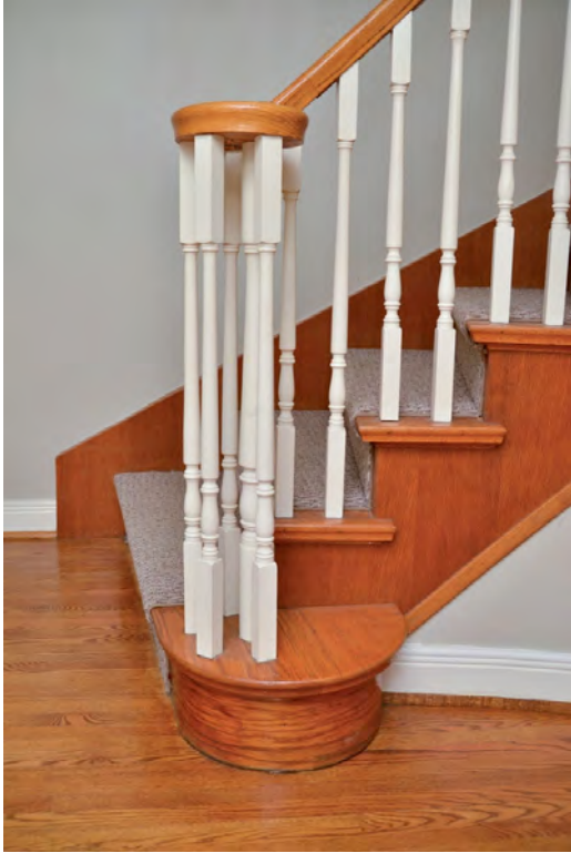
Fig. 30 Staircase newel post and balustrade
