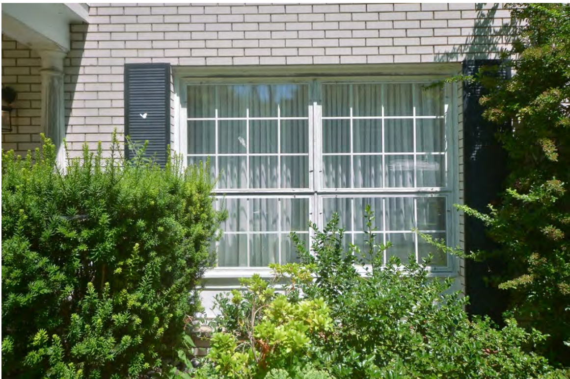
Fig. 21 Ground-floor window in front facade
