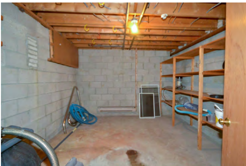
Fig. 51 Storage room in basement
