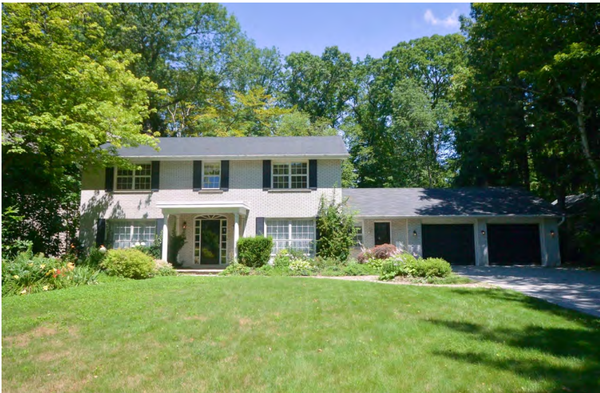
Fig. 19 Front facade (west elevation) of house and garage wing
