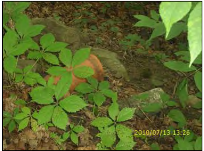
19. Pipes into ravine
