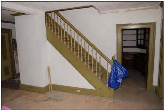
STAIRCASE (BLEED-THROUGH OF KNOTS ON STRINGER AND PROPORTIONS OF STAIR AND RAIL SUGGEST RECENT CONSTRUCTION)
