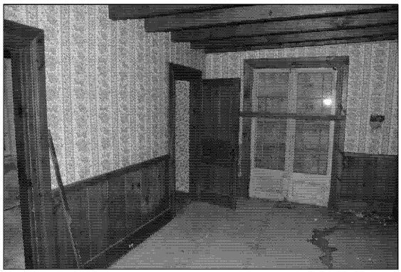
DINING ROOM IN EXISTING PRESUMED EARLIEST PART OF BUILDING (WALLS ARE DRYWALL FINISH, ALL TRIMS ARE NEW, EXPOSED JOISTS AT CEILING ARE NON-FUNCTIONAL, DOORS AT CENTER-REAR MAY BE ORIGINAL OR RE-CLAIMED)
