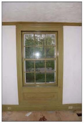
LIVING ROOM WINDOW (NOTE LACK OF SASH STOPS OR HARDWARE – SASH JUST RESTS IN PLACE)
