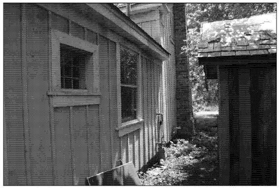
PARTIAL WEST ELEVATION (NOTE NON-STANDARD FRAME FOR CASEMENT WINDOW AT LEFT, NON-ORIGINAL CHIMNEY, ACCESSORY BUILDING AT RIGHT)
