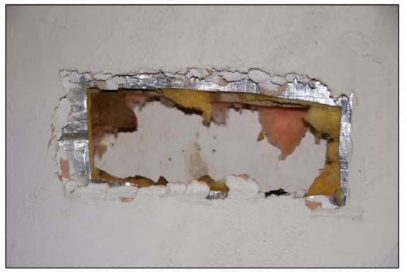
WALL ASSEMBLY IN MAIN FLOOR BEDROOM (NOTE MODERN INSULATION, DRYWALL, ORIGINAL PLASTER BENEATH)
