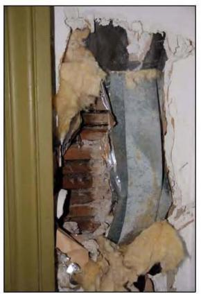
WALL ASSEMBLY NEAR FRONT DOOR (NOTE MODERN INSULATION, DRYWALL ON ORIGINAL BOARD-ON-BOARD FRAMING)
