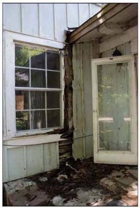
ROTTED SIDING FINISH (PREVIOUS HORIZONTAL SIDING VISIBLE BENEATH)
