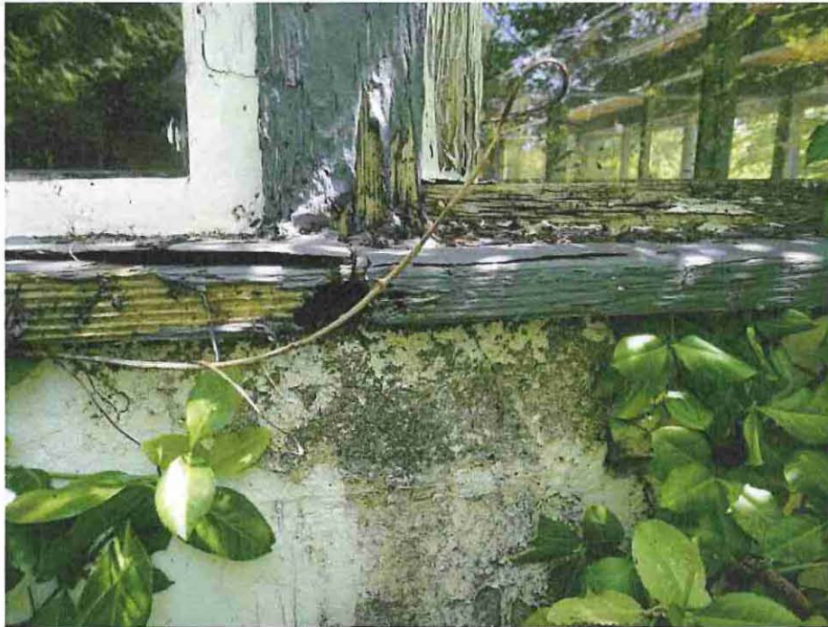
Photograph 5: Deteriorated and damaged wood window frames at Bldg. 1.
