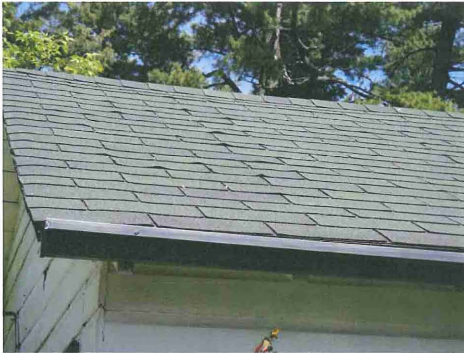
Photograph 15: Sloped gable roof with asphalt shingles over Bldg. 2.
