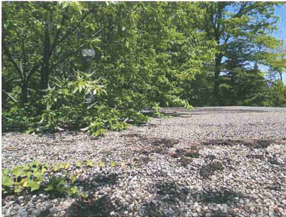
Photograph 3: Recently replaced conventional built-up roofing assembly over Bldg. 1.
