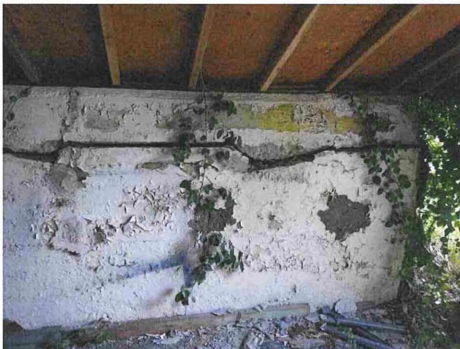
Photograph 29: Cracked and displaced concrete foundation wall in Bldg. 3.
