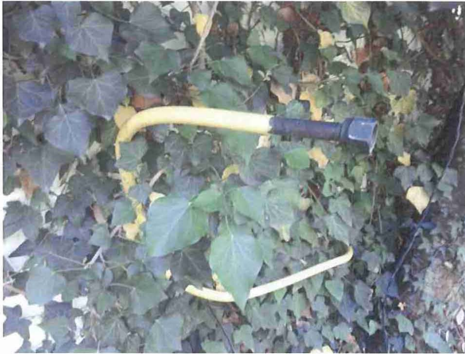
Photograph 11: Gas Line from Bldg. 1 furnace, previously was connected to a standalone propane tank.
