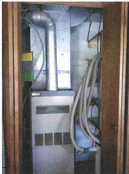
Photograph 10: Lennox gas/propane furnace located in Bldg. 1.
