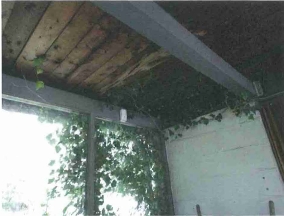
Photograph 7: Vegetation growing into the interior and along the stained wood strip decking of Bldg. 1.
