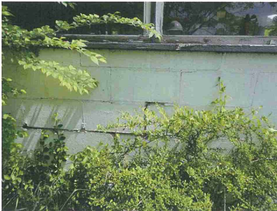
Photograph 4: Stepped crack through the concrete block retaining wall on the southwest elevation of Bldg. 1.
