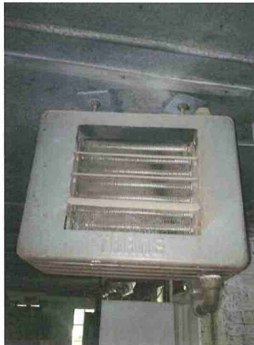
Photograph 24: Typical hydronic unit heater in Bldg. 2.
