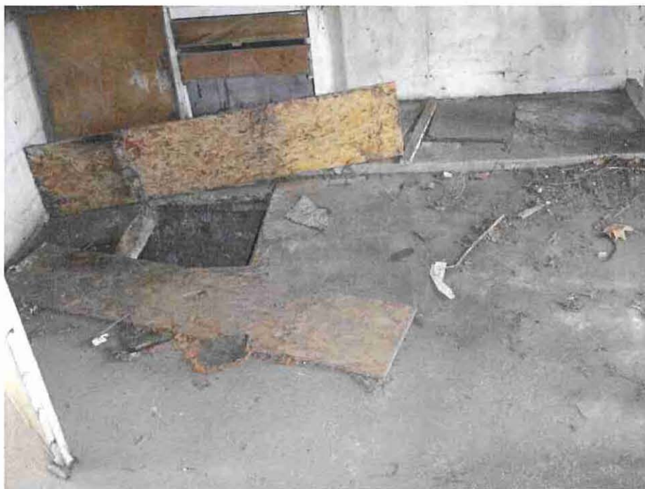
Photograph 17: Opening to the underground cistern at the east end of Bldg. 2.
