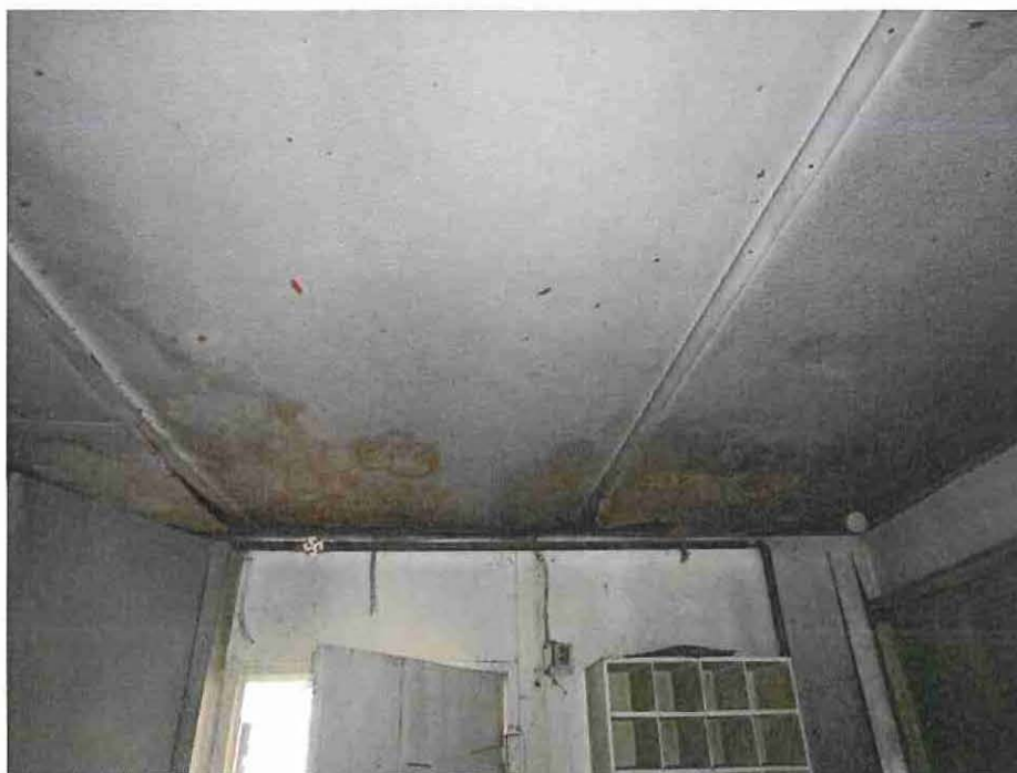
Photograph 18: Deteriorated and damaged ceiling panels over the entrance to the Greenhouses in Bldg. 2.
