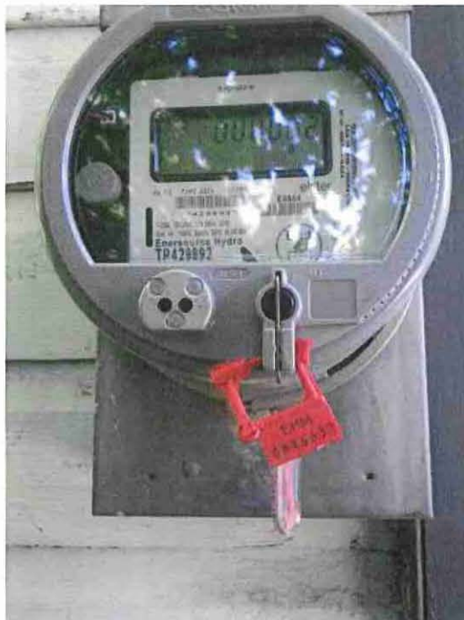
Photograph 26: Power meter mounted to the west elevation of Bldg. 2 that serves the entire complex.
