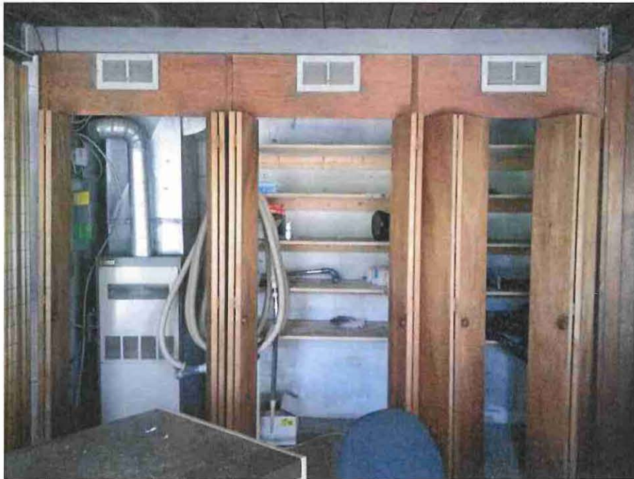
Photograph 9: Air distribution ductwork plus furnace at Bldg. 1.
