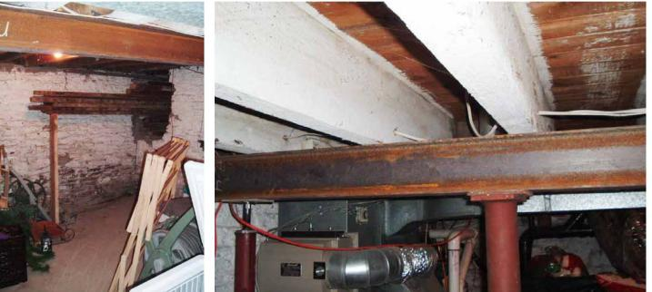
The photo below shows the wood floors of the original house supported by timber joists. Steel beams and jacks were added at a later date to reinforce the structure.
