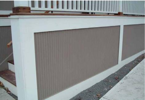
The porch at Pond Street containts more architectural features than any other location on the building. A line of small wood dentils runs along the top of the entablature and a simplified spandrel mimicking spindle work hangs below.
