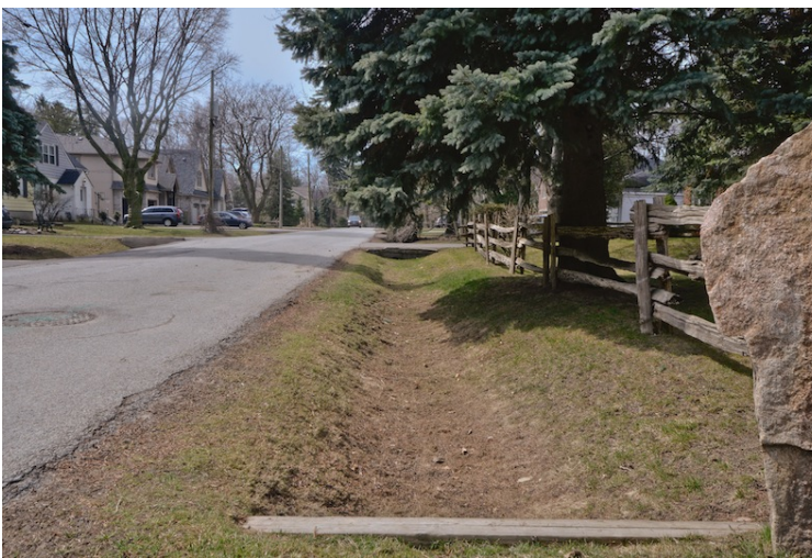
Fig. 6 Open ditch and culverts in front of 63 Veronica Drive
