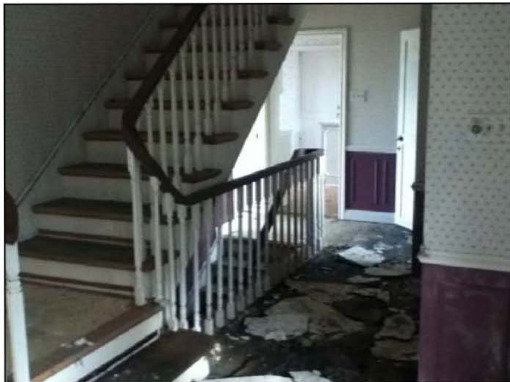
2-STOREY HOME – HALL – NOTE DAMAGE FROM WATER LEAKAGE
