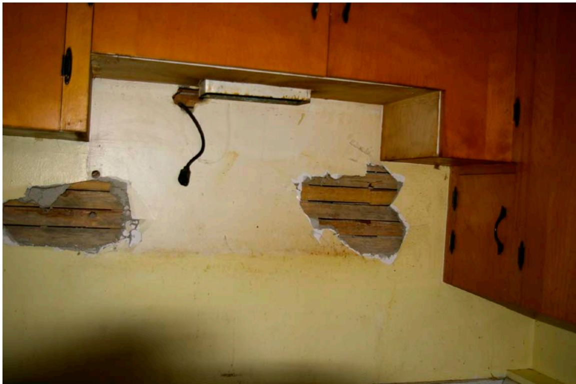
Photo 56 Broken plaster on the wall facing the window, where a refrigerator and stove were removed, shows the original wood lath and plaster construction.
