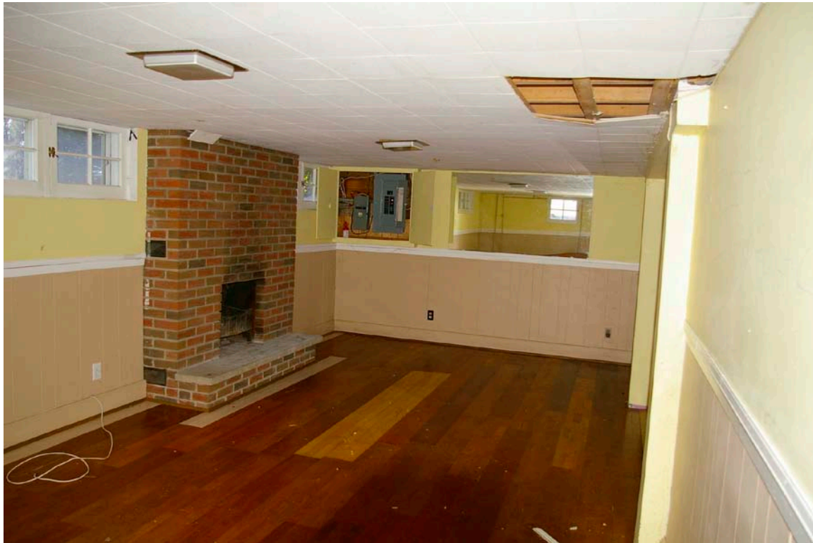
Photo 58 Basement looking towards the front wall, with a fireplace below the one in the living room on the east side of the house. Finished recreation room with laminate flooring (buckling in places due to water damage) and fireplace surround dating from the 1950s or 1960s.
