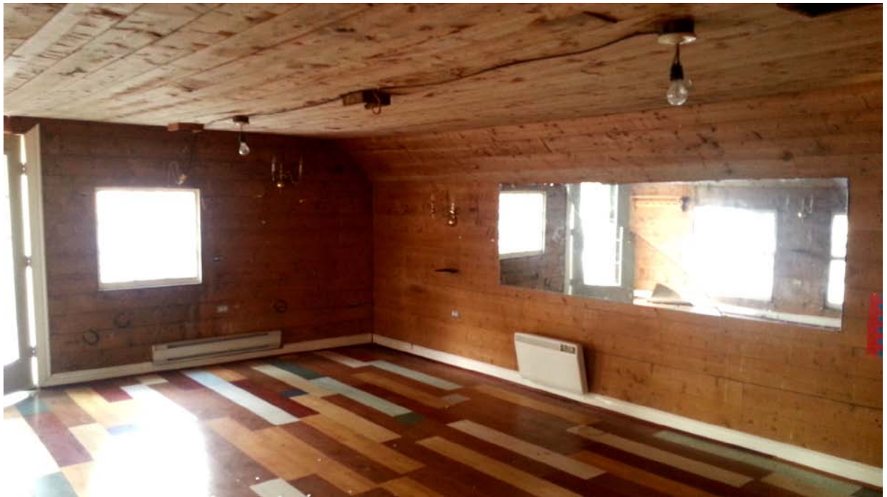
Photo 40 Interior of accessory building, with entrance doorway facing west on the far left and mirror on the rear wall. Wood plank ceiling with walls finished with horizontal wood boards and the concrete slab with laminate flooring.
