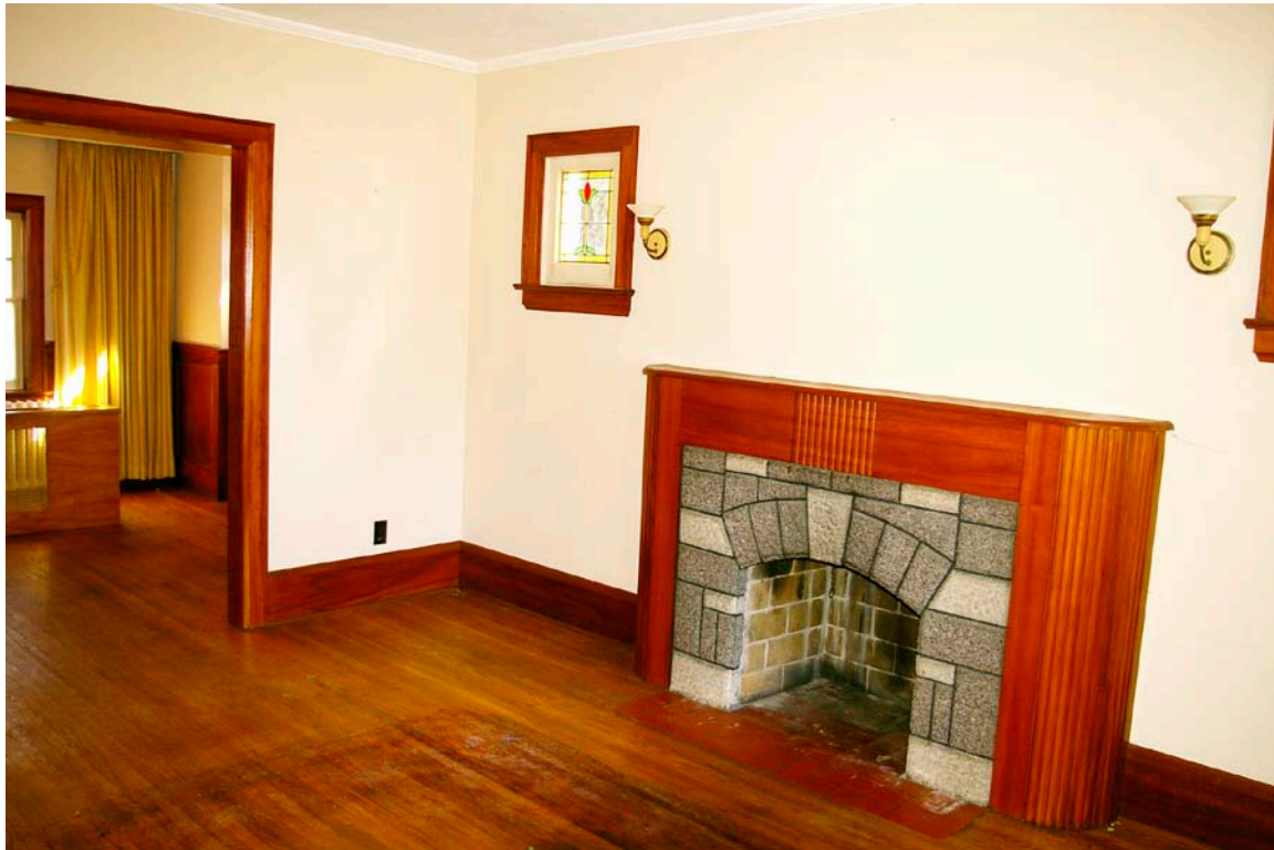
Photo 47 Living room looking through a doorway to the original dining room at the rear. Concrete block fireplace with a stone veneer facing and an Art Deco style mantelpiece, which is not original (MDF board construction and estimated to be 20-30 years old by the project architect, Andrew Reeves).
