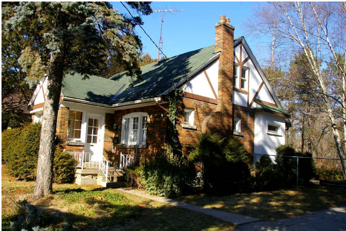
Photo 28 View of existing dwelling looking north-west, showing the concrete entrance stoop (not original) and doorway to the sun porch. The chimney serves the fireplace in the living room.
