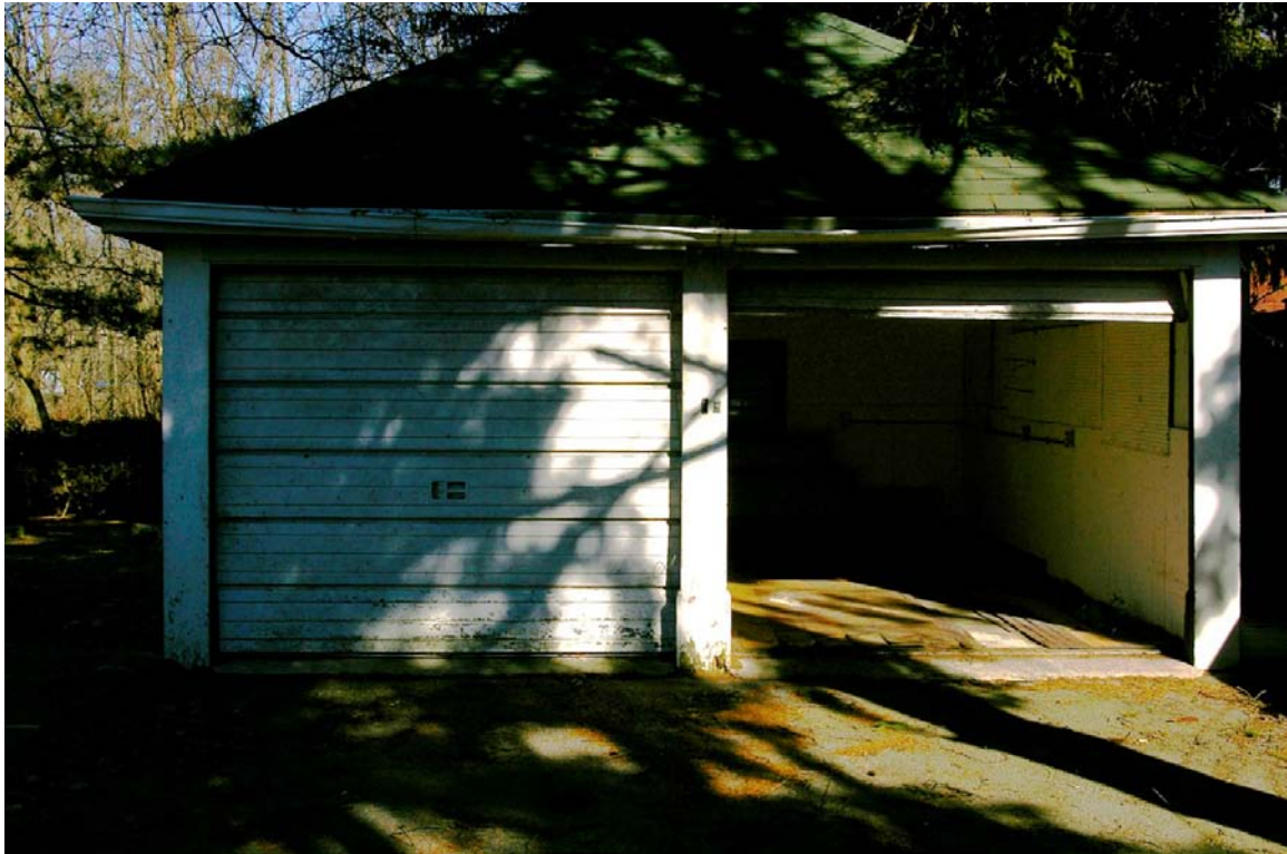
Photo 37 Freestanding two-car garage with two overhead rolling metal doors: frame structure on a concrete slab with a hipped roof and shiplap siding (condition: poor).
