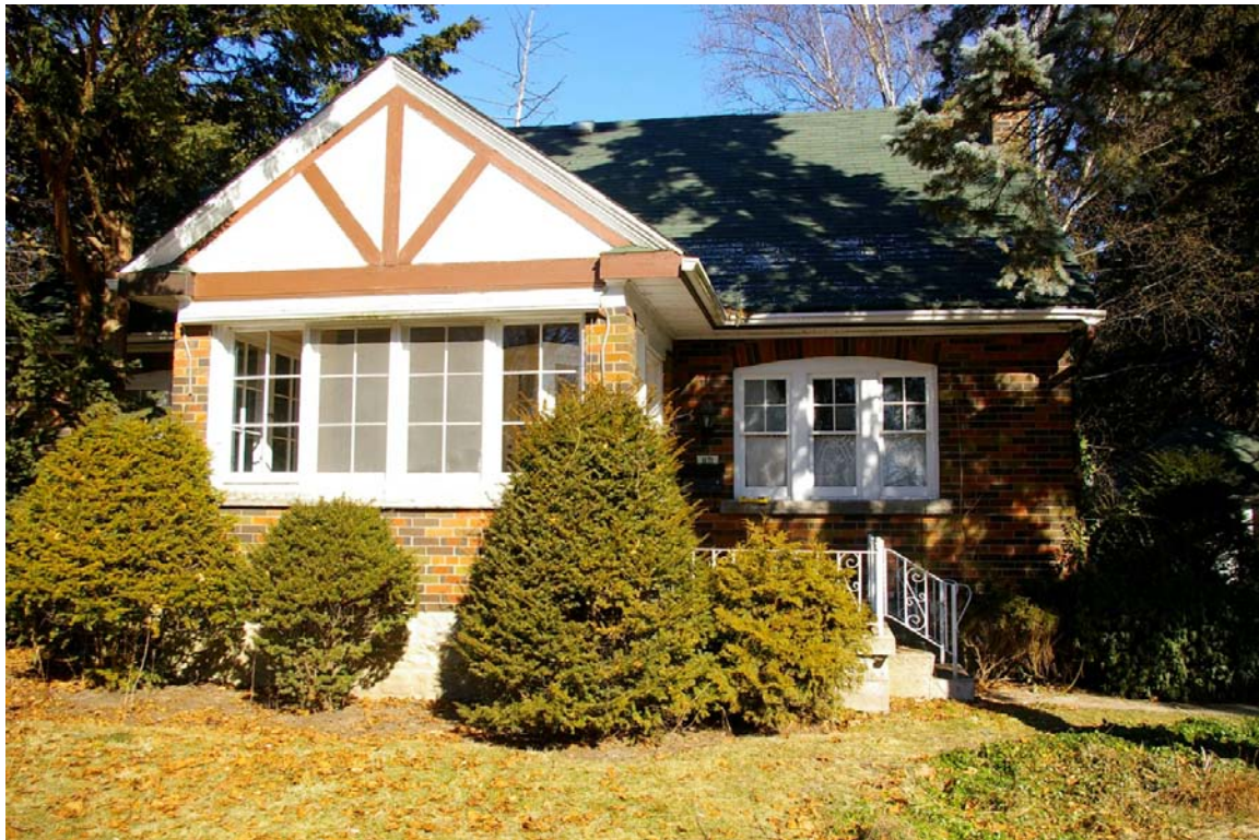
Photo 27 Front façade showing the entrance sun porch and the living room window to the right. The detailing of the roof gable with its stucco finish, half timbering and moulded soffits echoes that of the main end gables, shown in photos below of the east and west gables.
