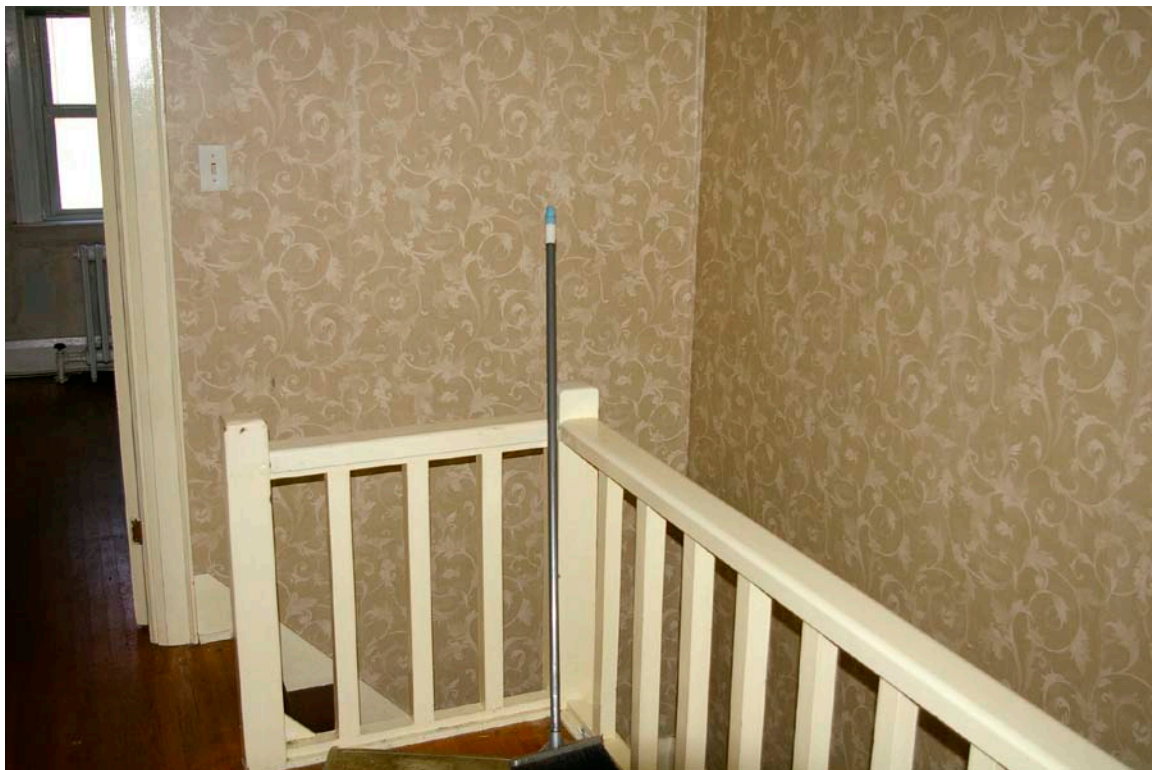
Photo 69 Upper hallway and stairs down to the main floor, with a simple wood balustrade (square balusters and newel posts). Doorway to the west bedroom on the left. Also shows the hardwood flooring in both bedrooms and the hallway.
