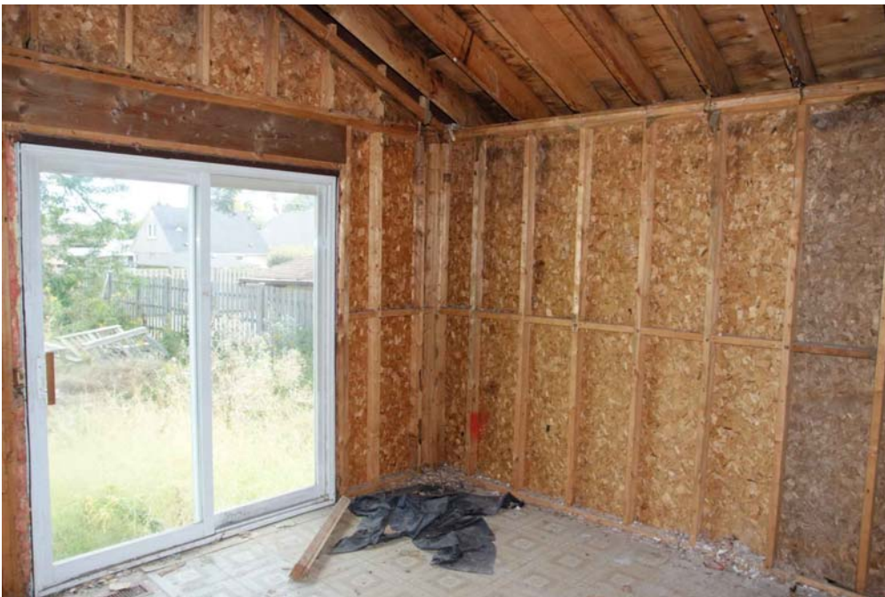
Typical interior framing at addition (note OSB wall sheathing, plywood roof sheathing)
