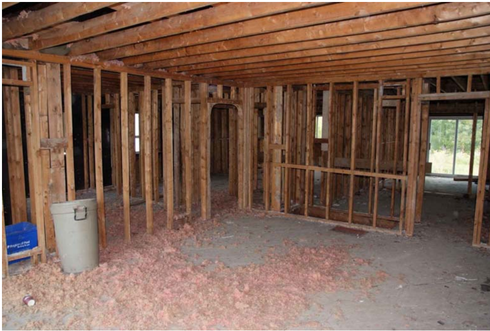
Typical interior framing original part of building
