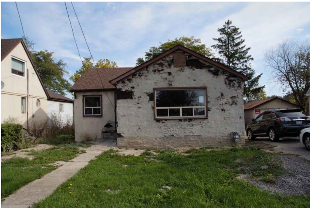
Front elevation (October 2012) showing garage and exterior finishes removed (note permit for partial demolition in front window)
