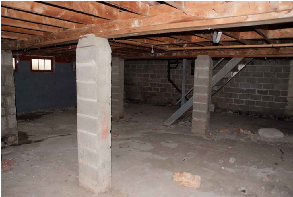
Typical basement concrete block construction
