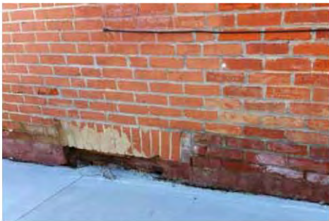
Detail of covered window on North wall at grade.
