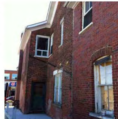
North wall shows evidence of an exterior addition.
