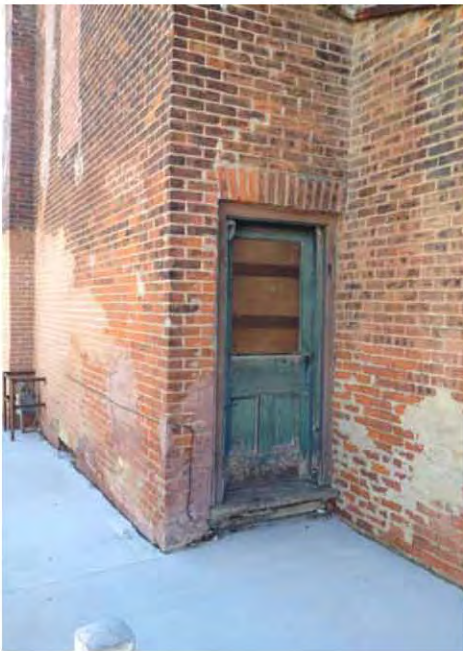
Deterioration of exit door and sill.
