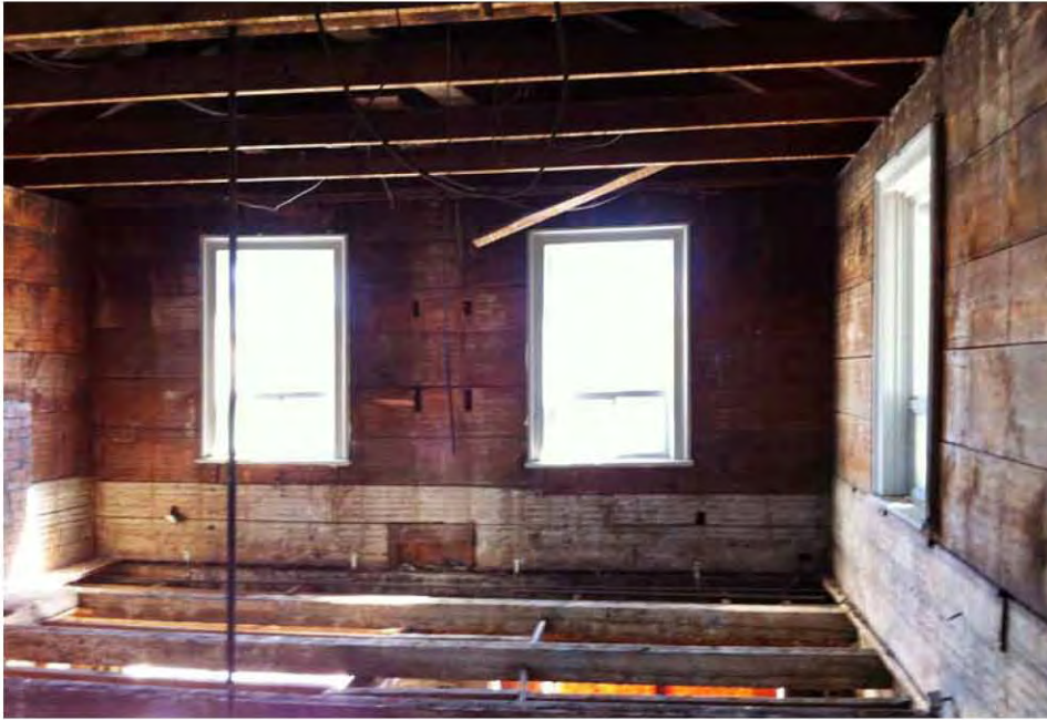
Second floor above store showing original wide planking and hand hewn floor joists..
