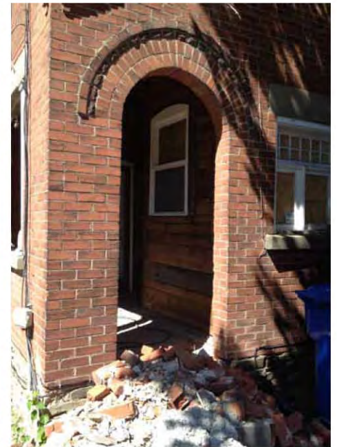
Radiating brick arch in portico.
