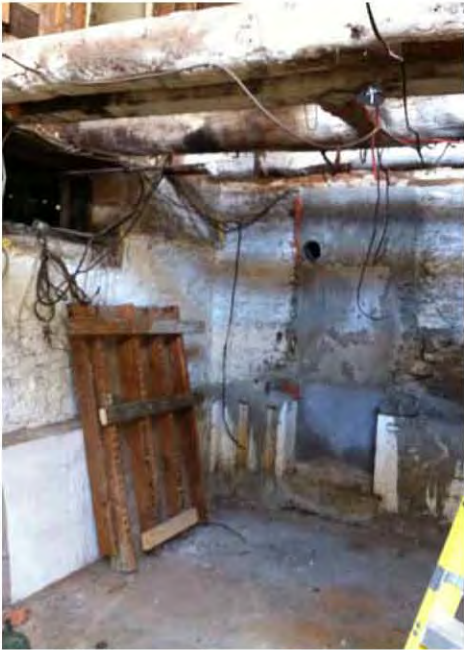
Detail of basement north wall with evidence of prior door.
