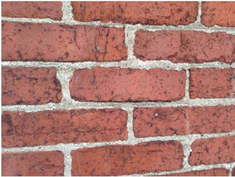
Photo 9: Bricks at the west addition appears to be a more modern extruded brick with black iron flecks. The brick is in sound condition, but the chipped/irregular edges will make cleaning the brick for salvage difficult.
