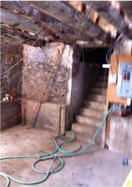
Bench footings used to lower basement floor.
