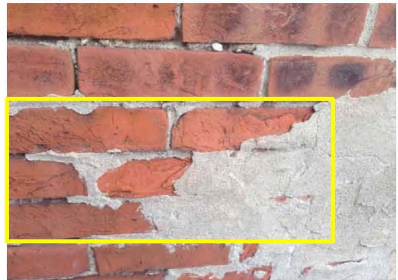
Photo 6: Original Brick – Bricks in the top 2 courses of this photo appear to be in sound condition and could be left in place or salvaged for re-use at the building. Bricks with eroded/sandblasted surfaces (yellow box) could be re-used if the concealed inner faces are in sound condition. We do not expect the parged bricks (lower right corner of photo) could be cleaned for re-use.
