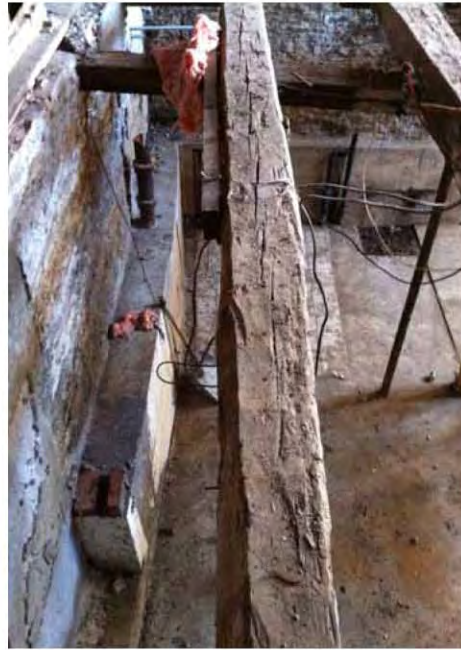
Detail of condition of hand hewn floor joist.
