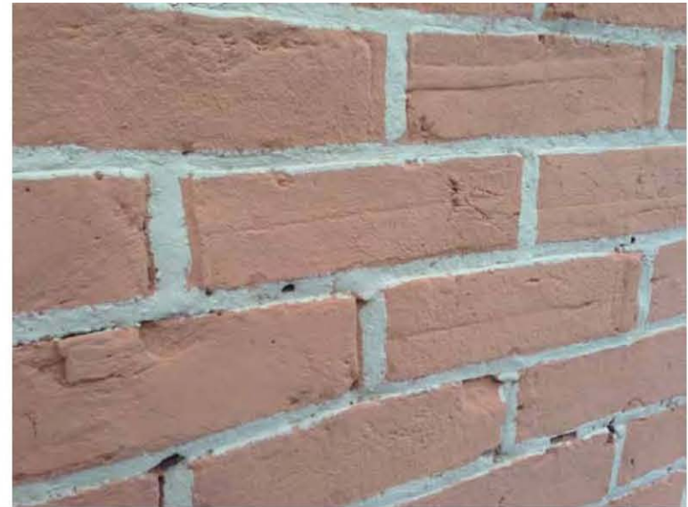
Photo 4: Painted brick and mortar joints. We expect the brick was painted to either "protect" deteriorated surfaces or to match the original brick. If the inner, unpainted surface of these bricks are in sound condition and match the original brick, they could be turned and re-used. If they are deteriorated and/or do not match, they should be replaced with salvaged brick.
