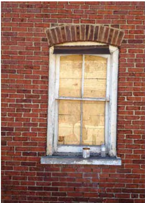
Deterioration of window frame & sill.
