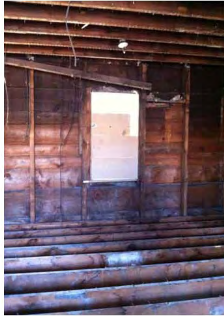
Evidence of fire damage to side wall.
