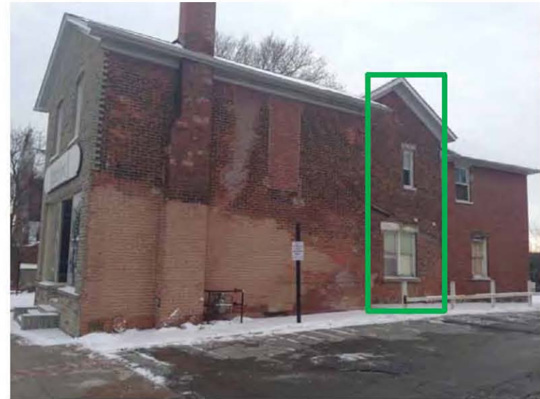
Photo 2: North façade, east end (left side of photo): The older brick from the “middle third” of the north façade (green box; this is the area west of the building “jog”) will be removed. Salvageable brick taken from this area will be used to restore the east façade and the east half of the north wall.
