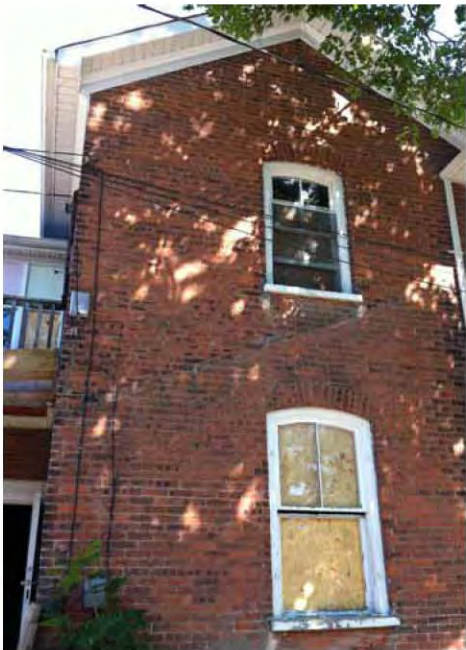
Middle portion of south wall showing the "boarding" up of a damaged window.
