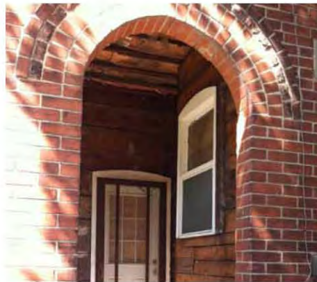
Front entrance to Portico. Original brick veneer has already been removed.
