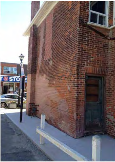
Shows brick deterioration and previous alterations.
