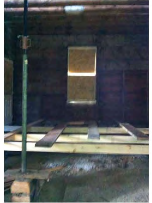
Temporary support column used to hold up the rear of building.
