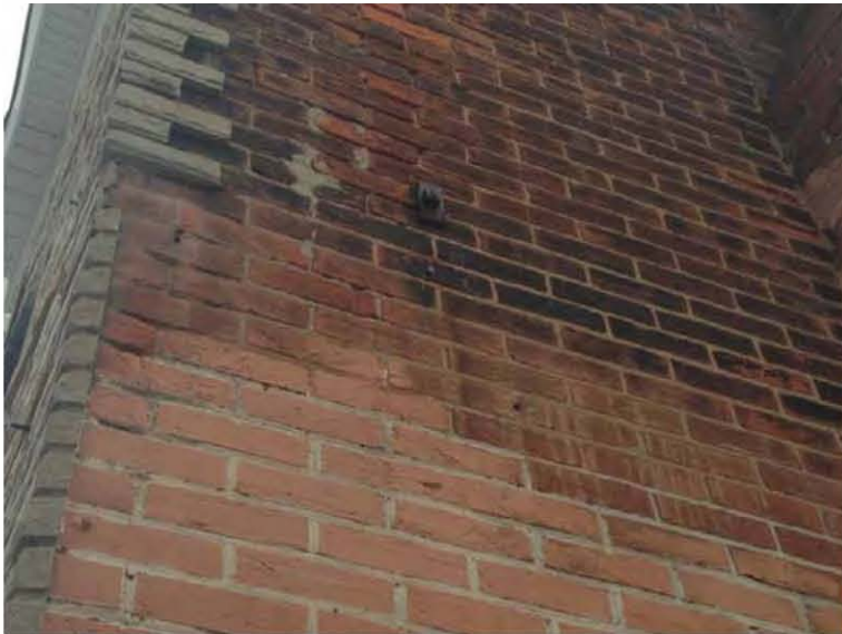
Photo 3: Many of the bricks at the 1 st storey, northeast corner have been painted ("pink" bricks at the bottom of photo; see also Photo 4). Brick faces at the 2 nd storey are eroded, likely from leaky eavestroughs. If the concealed inner faces of the eroded bricks are in good condition, the bricks could be turned to expose the sound surface and re-used. If all surfaces are eroded/deteriorated, the bricks should be replaced.
