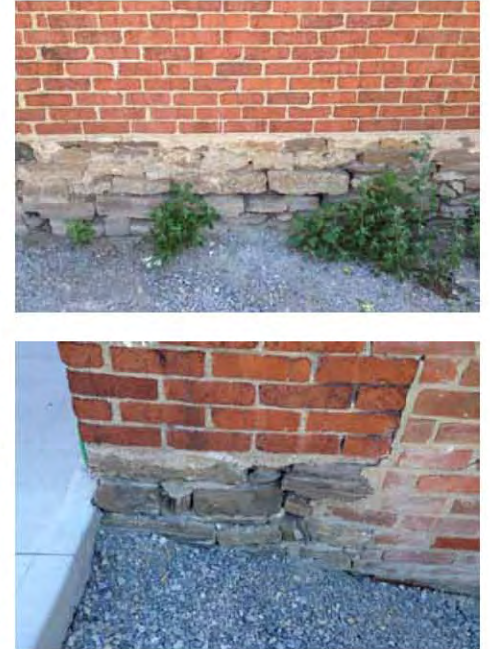
River stone foundation requiring repair.
