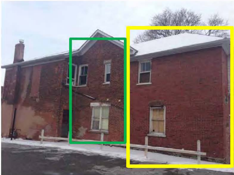
Photo 7: The western third of the north wall (yellow box) is a newer addition that is clad with more modern extruded bricks. A previous fire affected the structure in these areas. We understand that the addition will be removed so that a new addition can be constructed. The older brick from the “middle third” of the north façade (green box) will be removed and salvaged for re-use on the east façade and the east half of the north wall.
