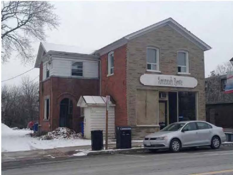
Photo 1: The east façade (facing Queen Street) is over-clad with “angel stone” veneer, and the south façade is clad with brick and siding. We understand that the “angel stone” will be removed to expose the original brick.
