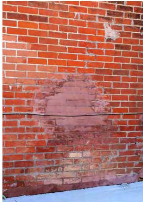
Numerous brick repairs and patching.
