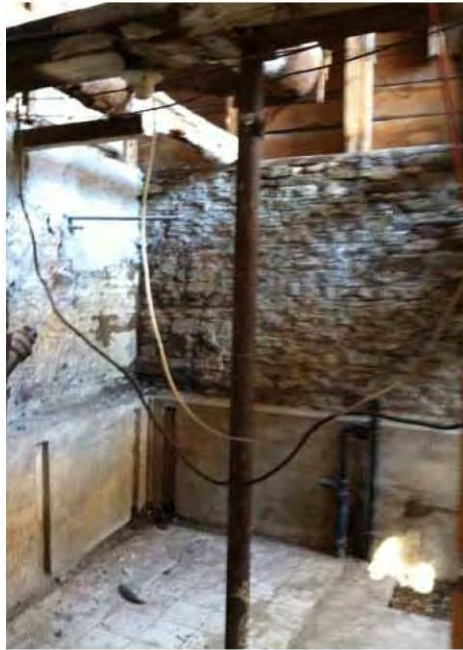
Detail of extent of river stone foundation under original building.
