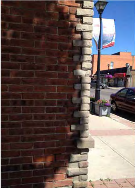
Coining detail at South Wall applied over brick.
