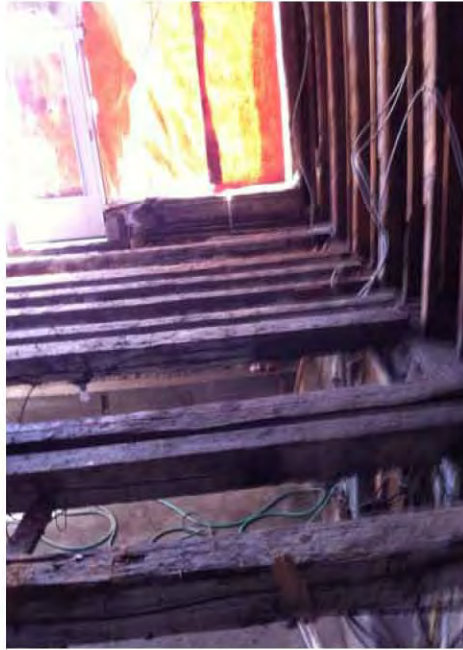
Detail of condition of hand hewn floor joist in original building.
