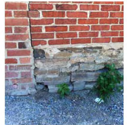
Detail view of the original river stone foundation requiring repointing. Note crack in masonry between additions.
