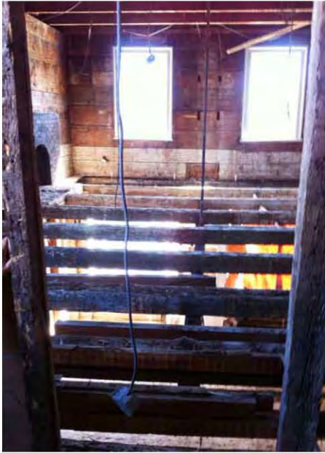
Second floor showing hand hewn floor joists.
