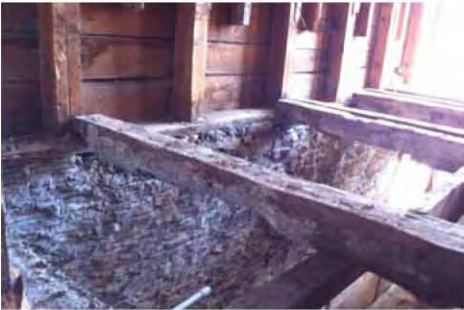
River stone foundation with hewn floor joists..
