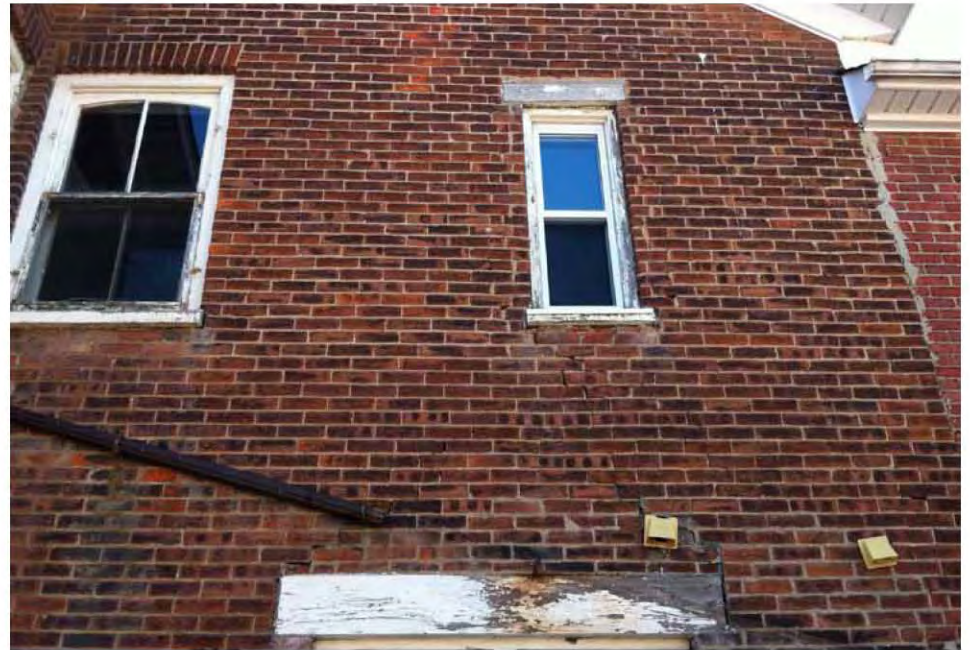
View of existing wood windows that require replacing. Note that the lintels above the windows are not consistent. The window to the right is likely a later addition.
