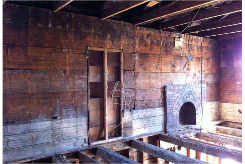
Second Floor detail showing fireplace, evidence of prior door and wide plank interior siding.
