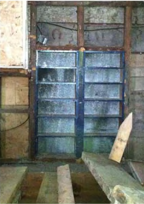
Evidence of possible opening in basement wall.
