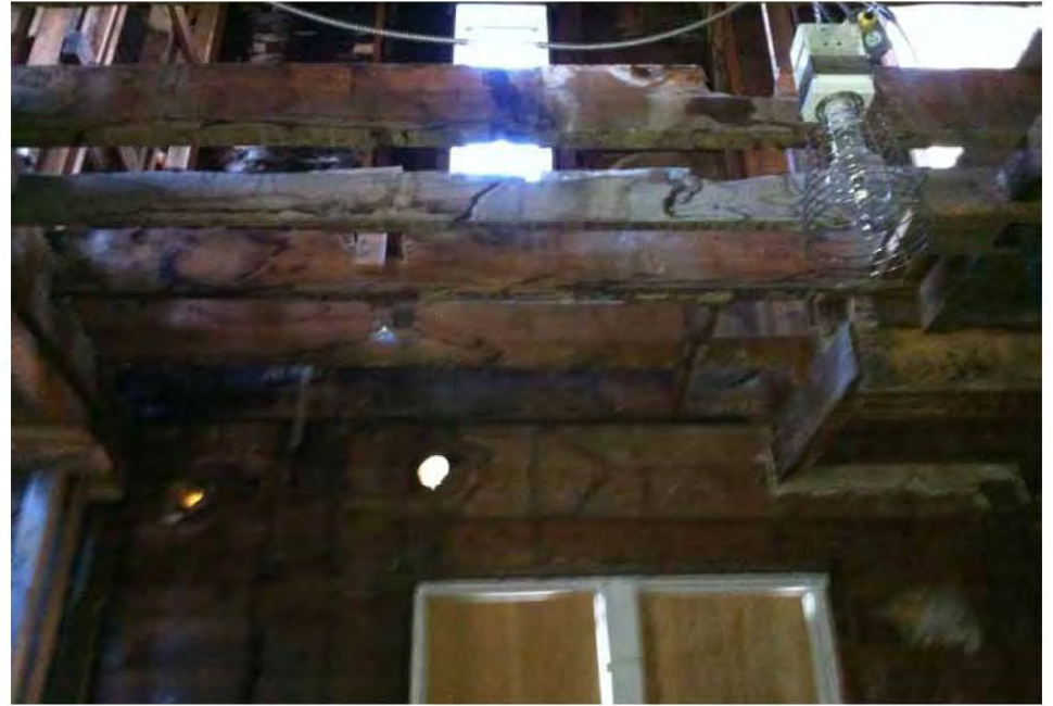
Evidence of fire damage "charring" to second floor joists.
