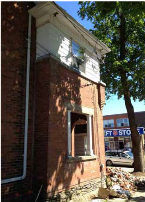
View of the only existing downspout located on south side of building.
