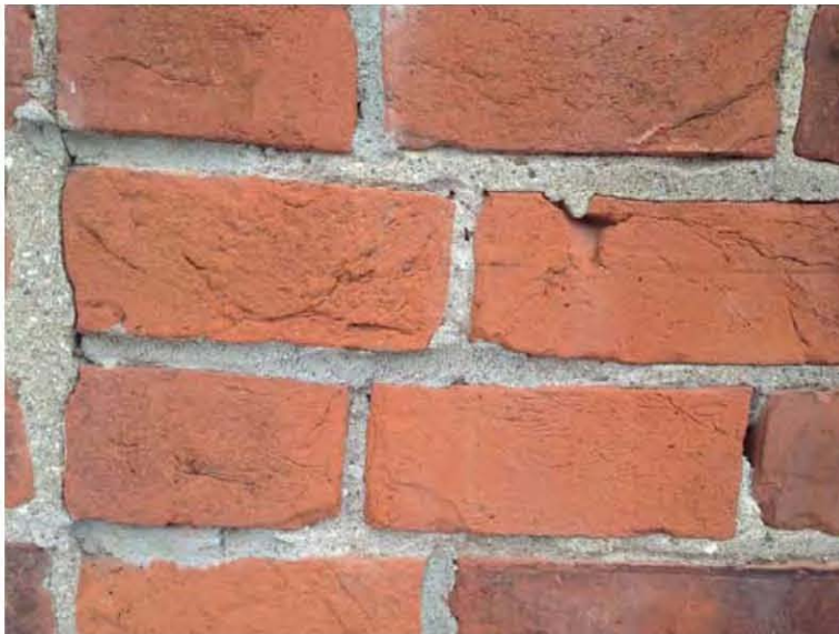
Photo 5: Original Brick - It appears that some brick areas may have been sandblasted in the past, as the hard “fire skin” of the brick is missing. The brick surface has subsequently eroded, exposing the “veins” of the inner brick body. This brick will be prone to continued deterioration if left exposed. However, if the concealed faces are in good condition, the bricks could be turned and re-used.
