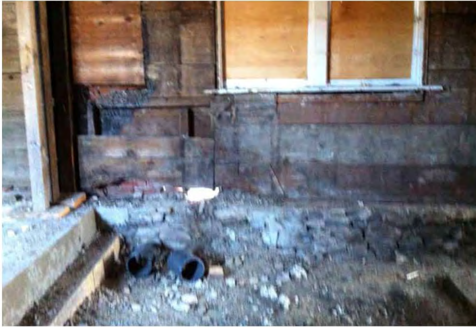
View of middle ground floor showing fire damage at left corner.
