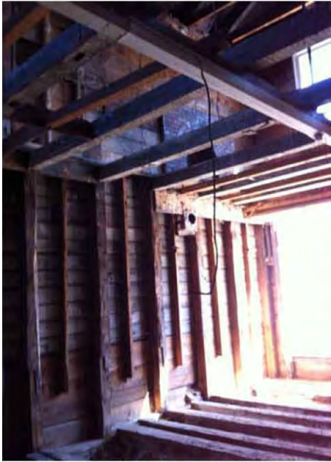
View of main floor from mid-section showing hand hewn logs as joists.
