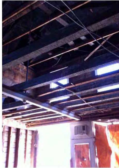
Detail of floor joists.
