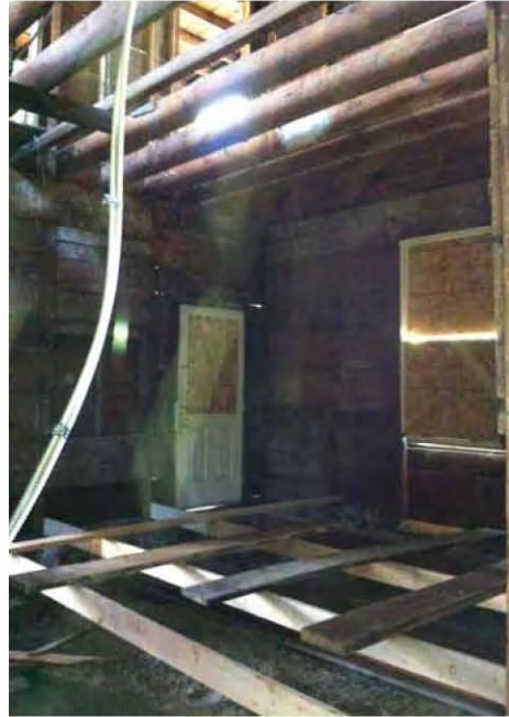
Rear view showing interior "milled" floor joists.
