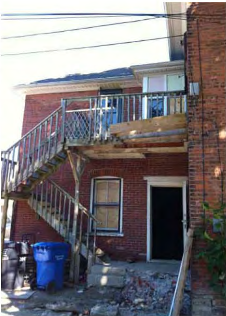
Wooden fire escape to second floor.
