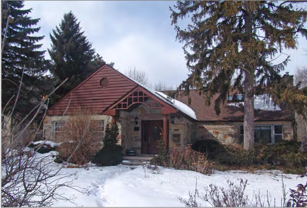
Above: East (front) facade showing wood clapboard gable and vent; open entrance portico with lattice work in gable and turned posts; bay window on right
