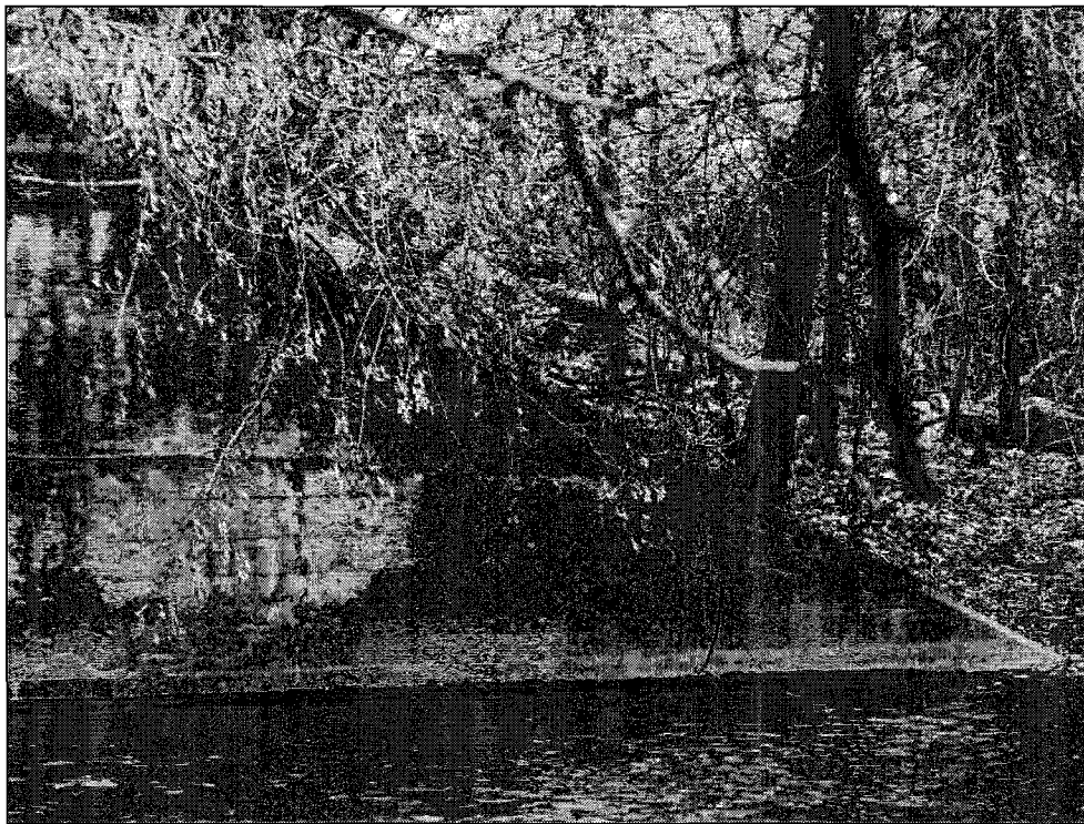
Photo P6– Typical Condition of East Abutment (good condition – stained cracking, isolated spalls and light scaling)
