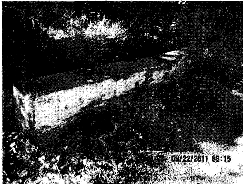
A2: Top of Existing Culvert Abutment
