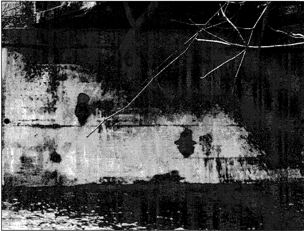
Photo P9– Typical Condition of West Abutment (good condition – localized spalling)
