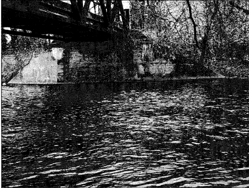
Photo P3— Typical Condition of East Abutment (good condition – stained cracking, isolated spalls and light scaling)
