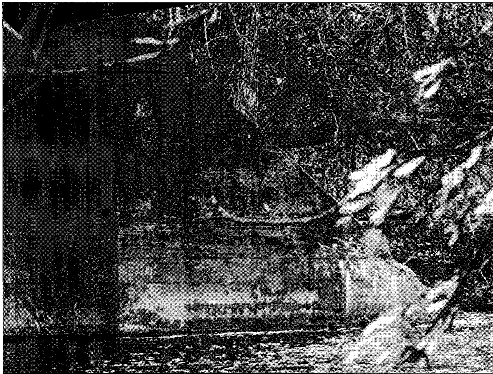
Photo P10– Typical Condition of West Abutment (good condition – localized spalling)
