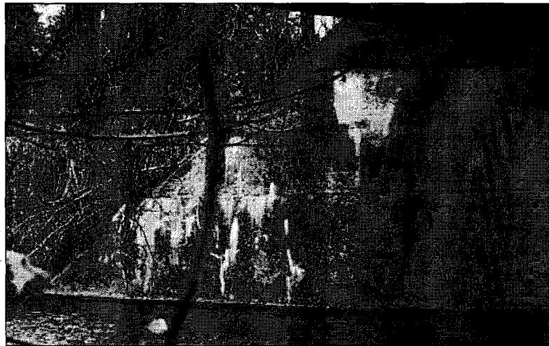
Figure 4: Typical Condition - stained cracking, isolated spalls and light scaling
