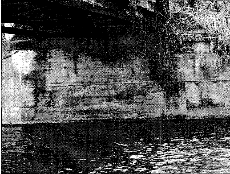
Photo P5– Typical Condition of East Abutment (good condition – stained cracking, isolated spalls and light scaling)
