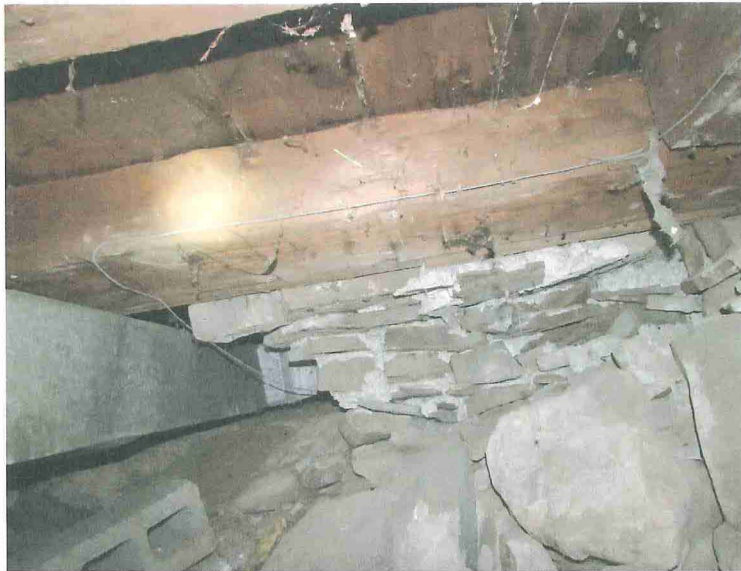
1880s foundation beyond 1840s timber sill plate
