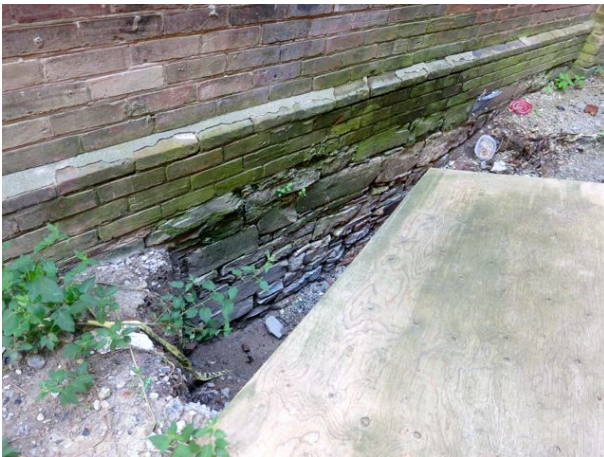
Figure 6: Original rubble stone foundation and a brick apron approx. 6 courses high with a beveled cap. The rubble stone foundation will be repaired.
