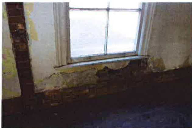
PHOTO #13: Local Brick Damage Around Secnd Floor Window
