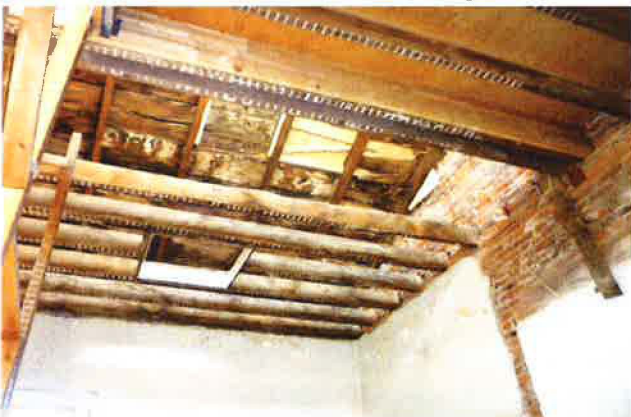
PHOTO #17: Roof Structure, Damaged Deck
