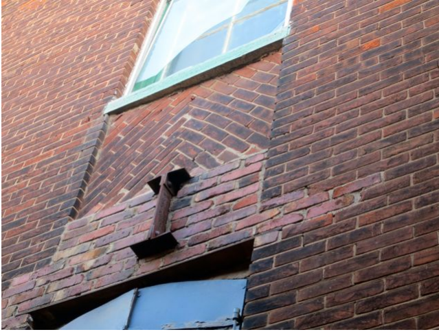
Figure 3: Modern steel I-beam set in the exterior masonry wall. These will not be removed.
