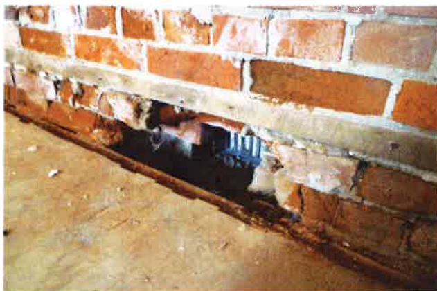
PHOTO #7: Foundation Damage From Previous Renovation
