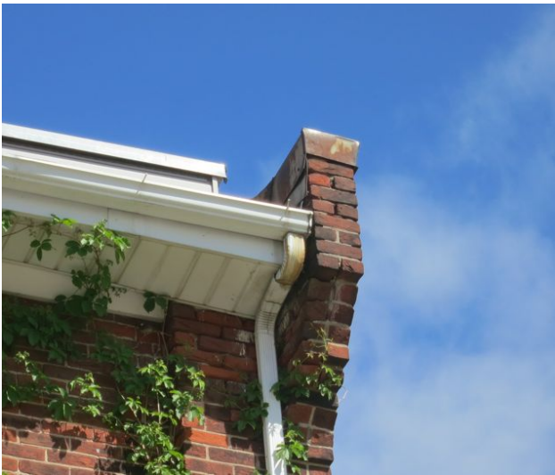
Figure 9: Original brick corbels at corners of the roofline will be repaired.
