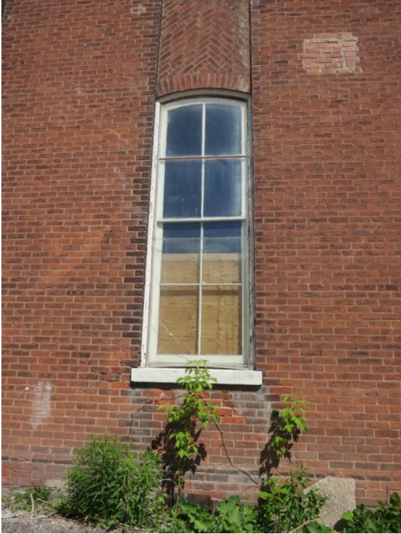
Figure 12: Large four over four wood sash window on the side elevation. These windows appear in the earliest photo of this building c. 1920. These windows will be removed and replaced with new units that will be similar in style and configuration.
