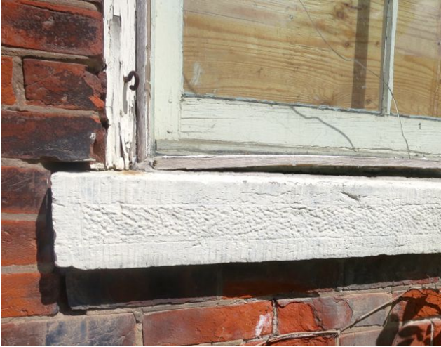
Figure 7: Original cut stone sills with a hammered finish will be retained.
