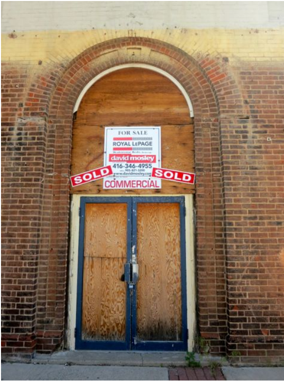
Figure 14: Original front doors have been replaced with an inappropriate metal and plate glass unit. This will be replaced with a wood frame door more in keeping with the character of the building, based on early photographs.
