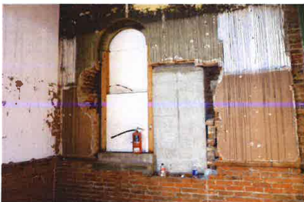
PHOTO #15: Front Window Previous Renovation Damage
