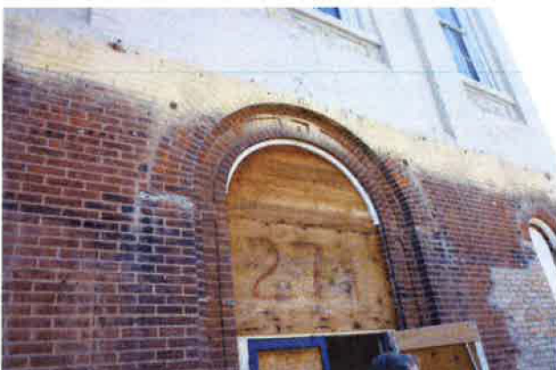
PHOTO #5: Front Door Showing Minor Brick Damage
