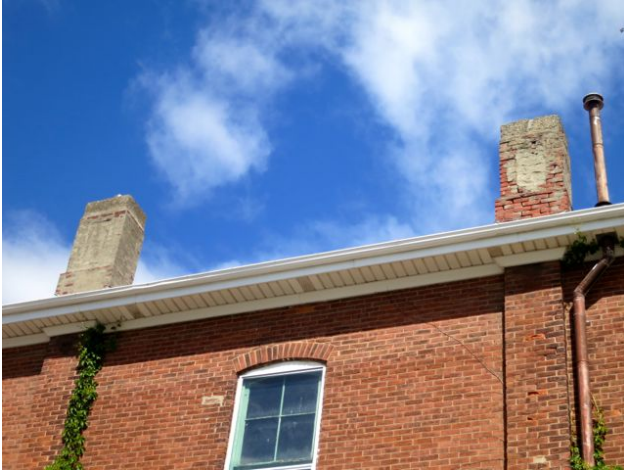
Figure 10: Original brick chimneys have been parged with a cementitious material. This will be inspected and repaired or removed.
