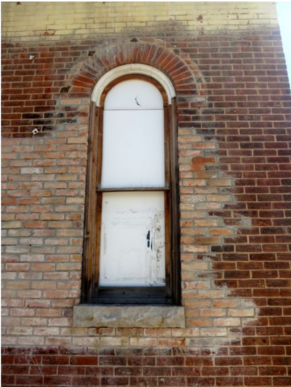
Figure 13: Replacement window on the main facade is in poor condition. Note also the inappropriate modern brick infill and the modern stone sill. The new storefront will cover this area.
