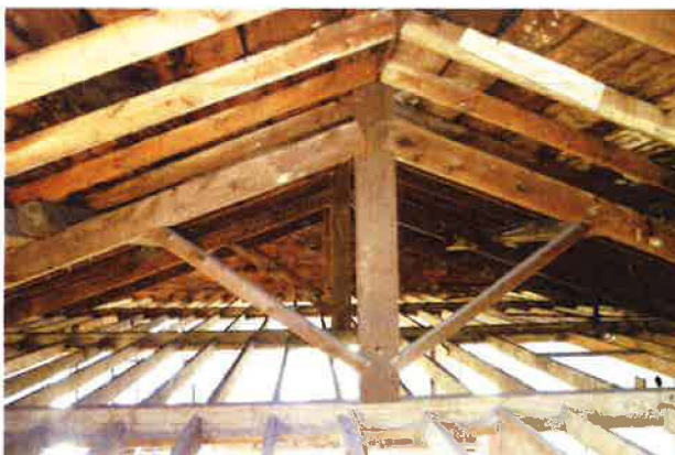
PHOTO #12: Main Roof Truss
