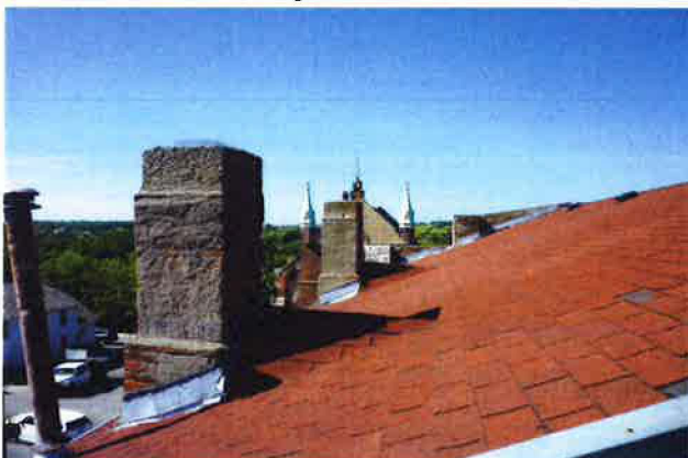
PHOTO #18: Roof Asphalt Shingles
