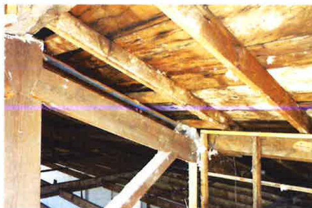
PHOTO #16: Roof Structure, Damaged Joist & Deck
