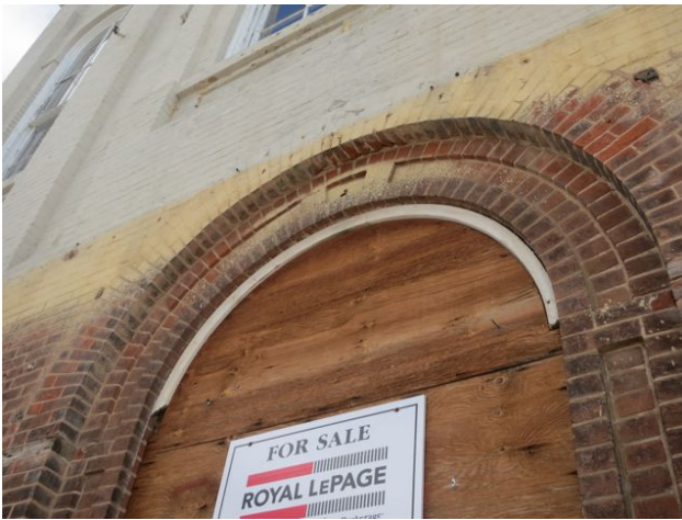
Figure 4: Original brickwork, including the recessed arch around the main entrance, will be retained.
