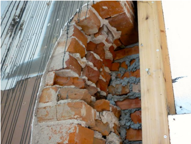
Figure 1: Original exterior masonry consists of 4 layers of locally produced red brick laid in common bond. Original interior plaster is applied directly to the masonry.
