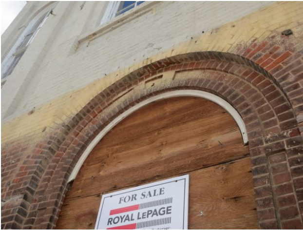
Figure 4: Original brickwork includes a recessed arch around the main entrance. This will be preserved under the new wood storefront.
