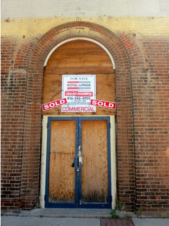
Figure 14: Original front doors have been replaced with an inappropriate metal and plate glass unit. Note also that the ground floor is unpainted but the upper storey is painted. The door is framed by a recessed brick arch. The new storefront will replicate this arch.
