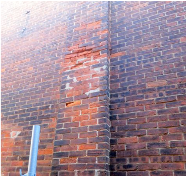
Figure 5: Brick piers on the side elevations that probably housed stove pipes for heating the interior. Damaged brick will be repaired.
