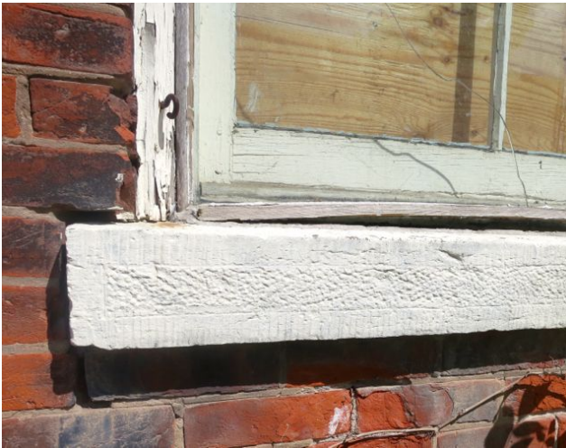
Figure 7: Original cut stone sills with a hammered finish. These will be retained.
