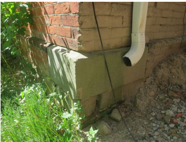
Figure 8: Original cut stone corner block at grade. These will be retained.
