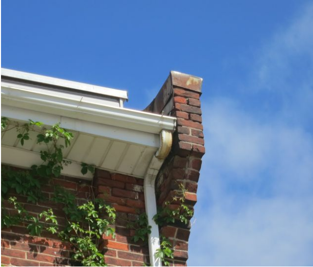
Figure 9: Original brick corbels at corners of the roofline. These will be repaired.
