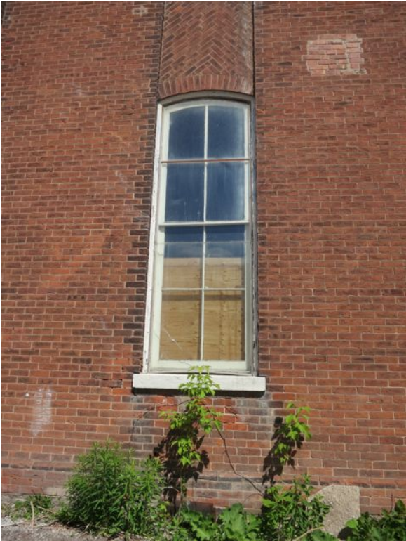
Figure 12: Large two over two wood sash window on the side elevation. These windows appear in the earliest photo of this building c. 1920. These windows will be removed and replaced with new units that will be similar in style and configuration.
