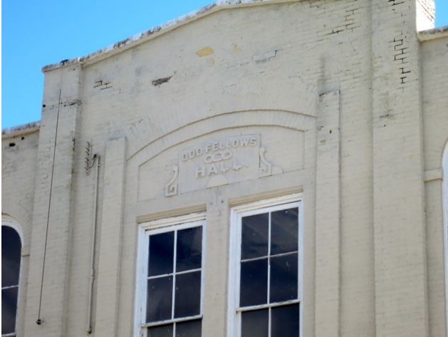
Figure 11: Original Odd Fellows' plaque on the main façade. The plaque will be painted in a contrasting colour to make it more visible from the ground. The brick will be scraped, primed and re-painted with a breathable paint in an appropriate colour.
