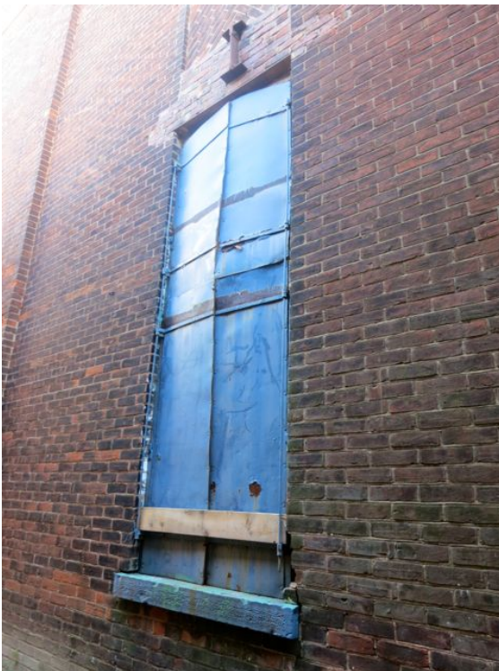
Figure 15: Several original windows on the ground floor have been replaced by modern metal doors for loading docks at the rear. These will be removed and replaced with new windows or doors that are similar in style and configuration to the original 4 over 4 wood sash windows.
