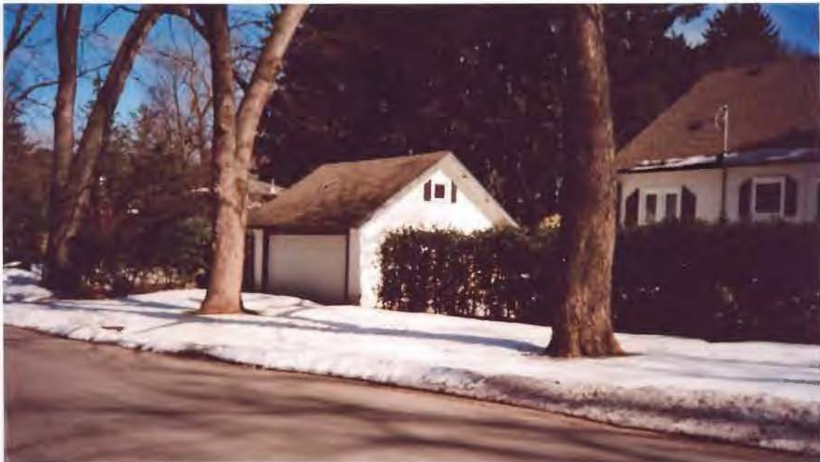
North West View
