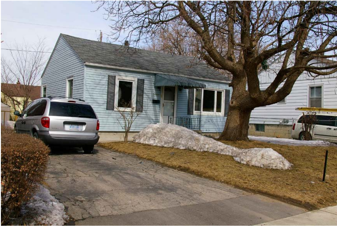
Photo 16: Front and west facades looking almost directly north.
