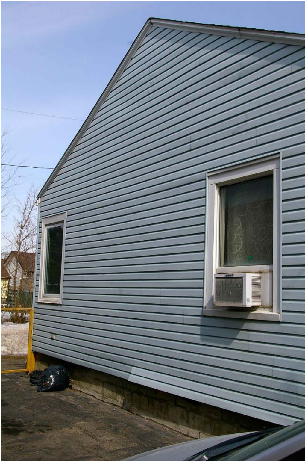
Photo 19: West facade on the driveway side looking north.
