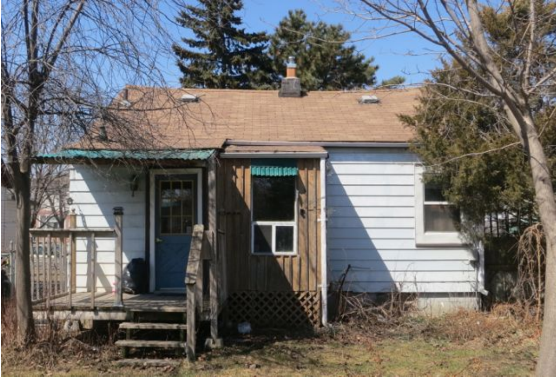
Figure 5: 3032 Churchill Avenue, rear elevation
