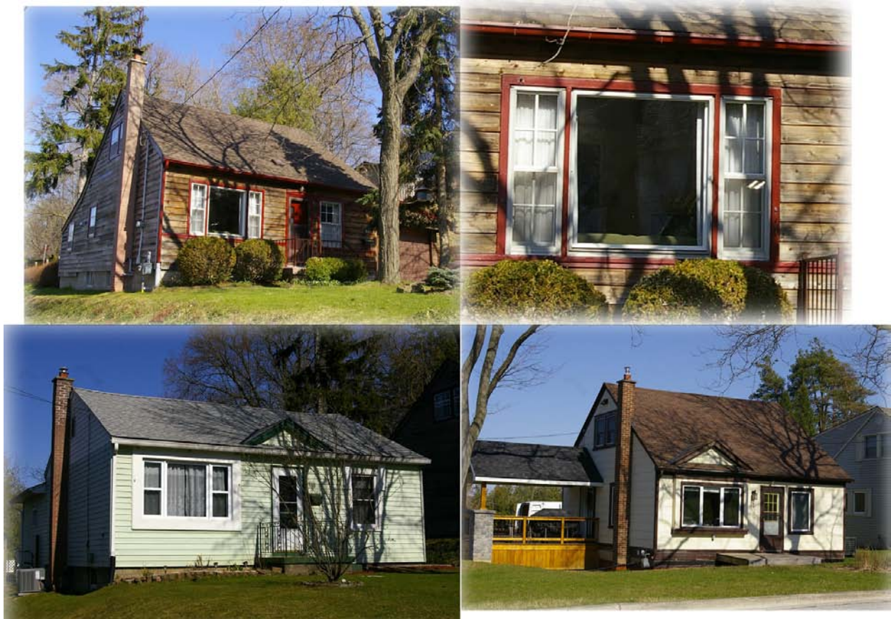
Figure 15: Collage of photos of wartime dwellings relocated to an enclave in Dundas in 1954 and set on full concrete block basements, where furnaces were installed and exterior brick chimneys added. They illustrate a common 1950s modification of dwellings based on a 24' X 28' plan: the enlargement of the frame of the living room window to accommodate a fixed centre pane with two narrow vertical sash windows on either side. (Top) 101 Head Street: a 1½ storey dwelling with an added garage, all sided with clapboard, and a detail of its original living room window with a near square centre pane and two narrow four-over-four sash windows. (Below) 99 Head Street: a 1-storey, vinyl clad dwelling with a similarly enlarged window (which appears to be a replacement for an earlier one but with the same configuration) and 91 Head Street: a 1½ storey dwelling, notable for the survival of its original asbestos shingle siding. Both dwellings have decorative roof gables; the one at #91 was clearly added at the same time as the projecting bay with a picture window.
