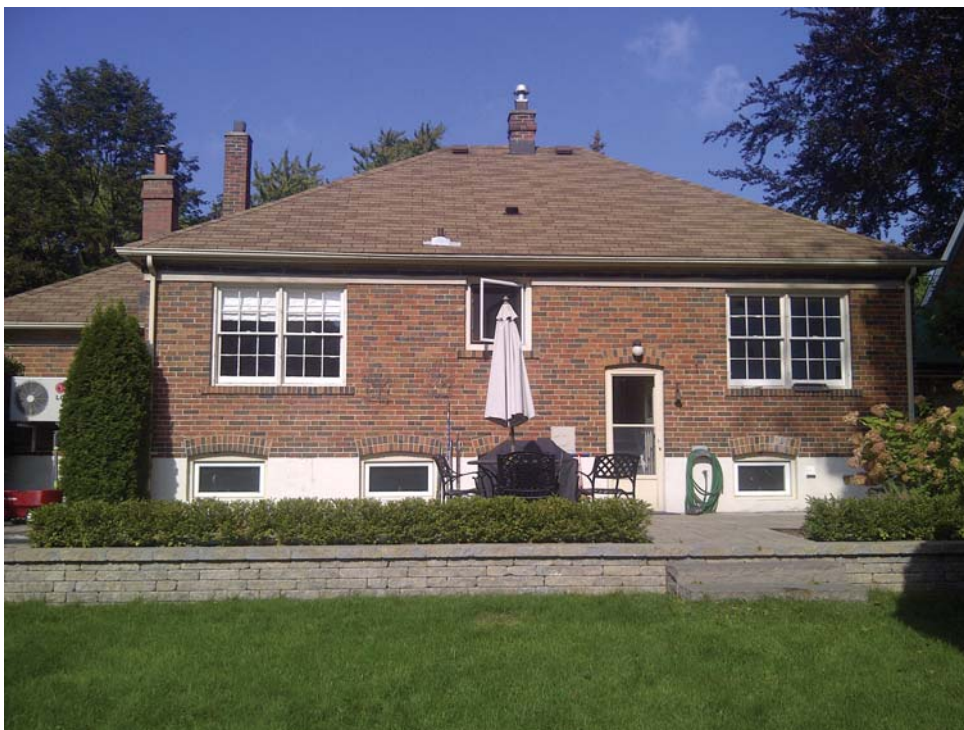
Figure (11): View of rear facade (south elevation).
