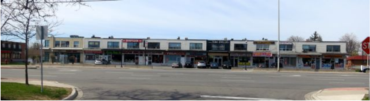
Figure 38: View to Airport Road from Churchill Avenue
