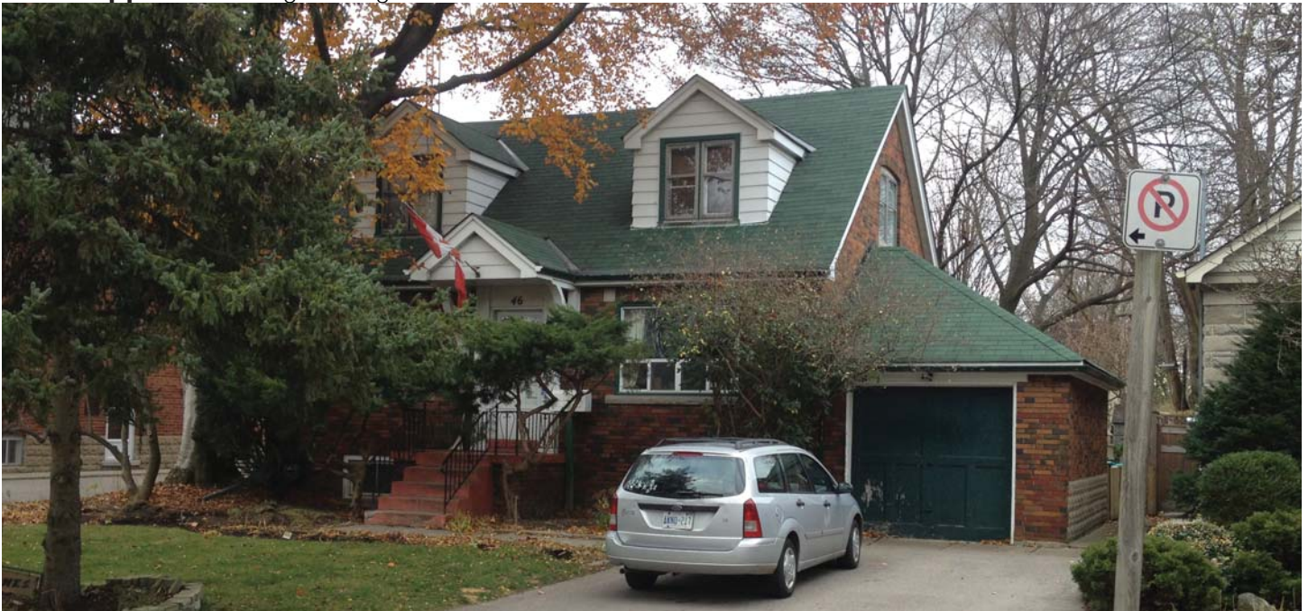
Dwelling immediately east of subject property: 46 Inglewood Drive.
