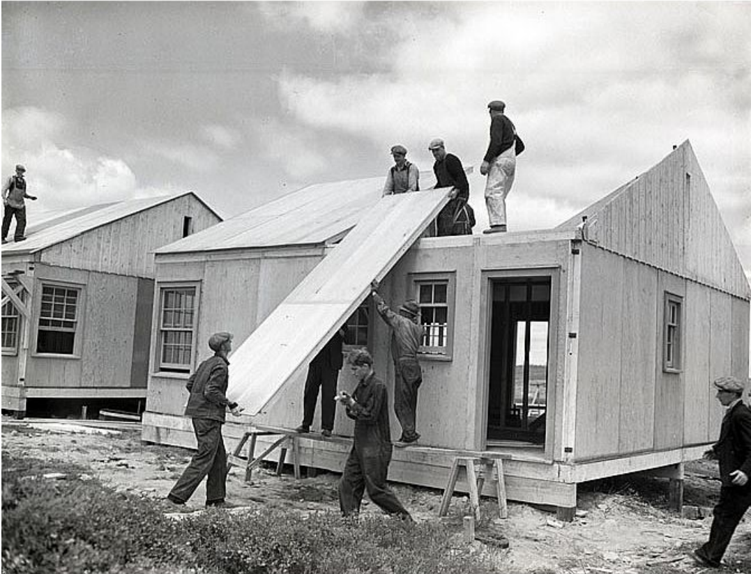
Figure 24: War-time workers' housing being assembled from pre-fabricated components
