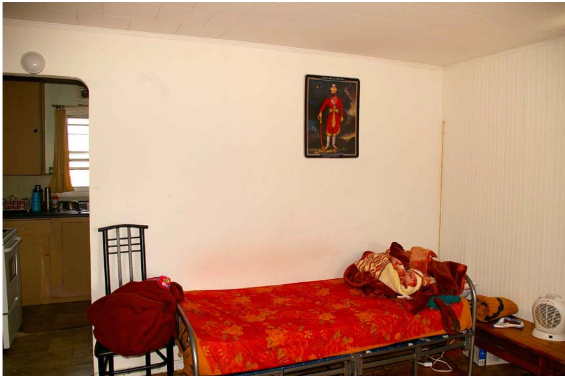
Photo 29: Rear wall of living room with the archway to the kitchen on the left.
