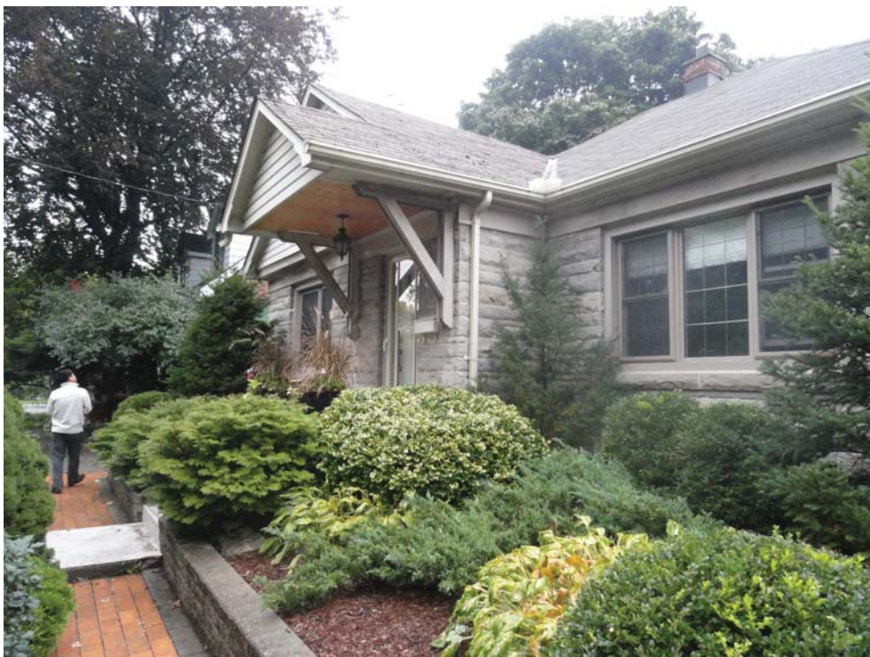
Figure (9): View of entry canopy.
