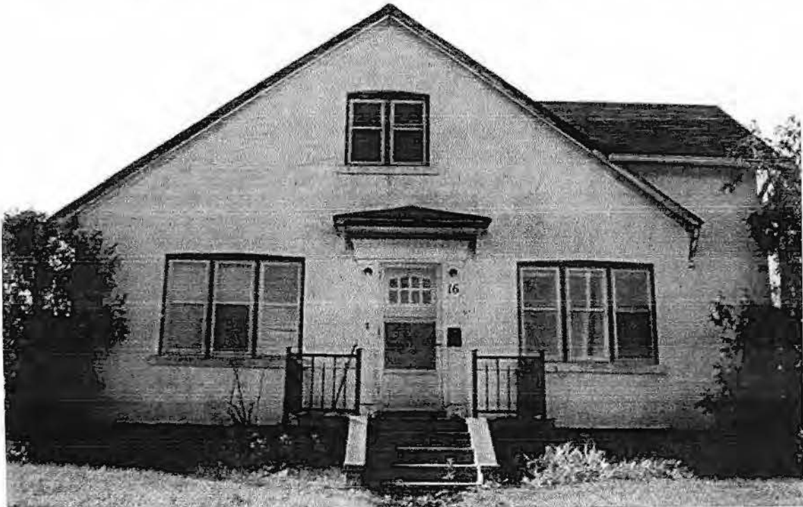
10 Front Street South, Port Credit
