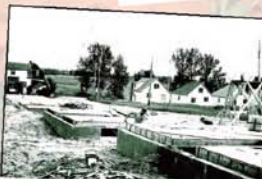
New home construction in the St. Mary's neighbourhood, circa 1946. Kitchener-Waterloo Record Photographers Record Collection, Dana Pinner Library, University of Waterloo.
