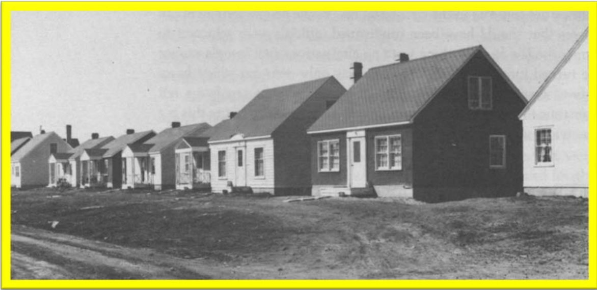
Figure 11: View of part of a streetscape of dwellings built by Wartime Housing Inc. in Edmonton in 1944, shortly after construction. In contrast to most wartime houses in Canada, these dwellings had full basements, a necessity for climatic reasons, with side chimneys suggesting that they were equipped with coal-burning furnaces in their basements.
