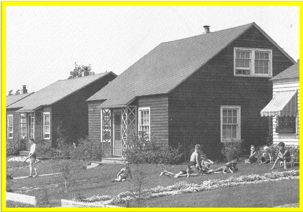
Figure 10: A typical streetscape of wartime housing in Peterborough, photographed shortly after completion in 1943. The houses shown were based on the same plan for a 1 ½ storey house with a steep-pitched, tight-eaved gable roof and projecting canopy over the front entrance with trellis-like supports; six-over-six paned sash windows. These dwellings had clapboard siding and the standard asphalt-shingled roofing. As was the case in many parts of Canada, these wartime dwellings had no basements and were supported on cedar or concrete posts. Heating was provided by a single stove on the main floor vented through a stove pipe (partially visible on the backside of the roofs).
