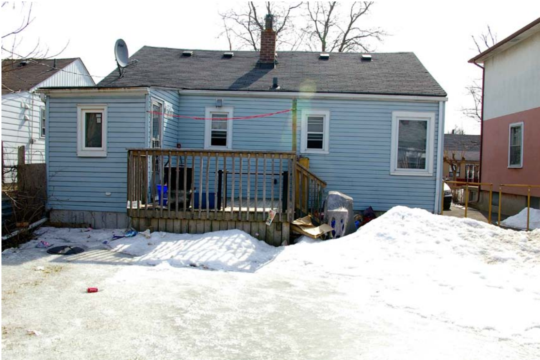
Photo 21: Rear facade looking south-east. Shows the rear addition (laundry room) and windows to the right of the extension (from left to right): kitchen, bathroom and bedroom.
