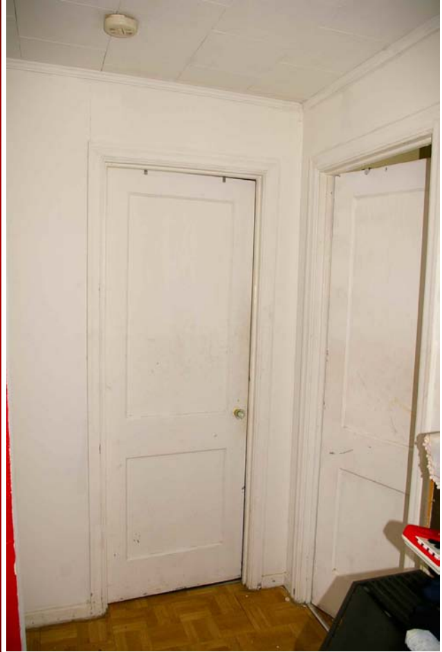
Photo 33: Rear bedroom doorway with bathroom doorway on the right.
