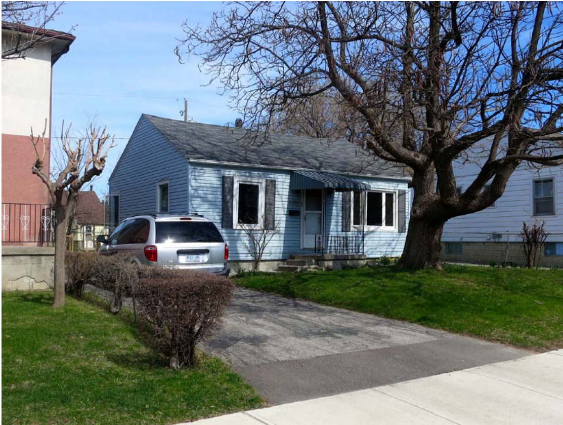
Photo 18: View of the subject property from the same vantage point as Photo 15 but showing fully the concrete stoop and side-facing concrete steps. Photo taken by Megan Hobson on May 5 th at the request of the author of this report.
