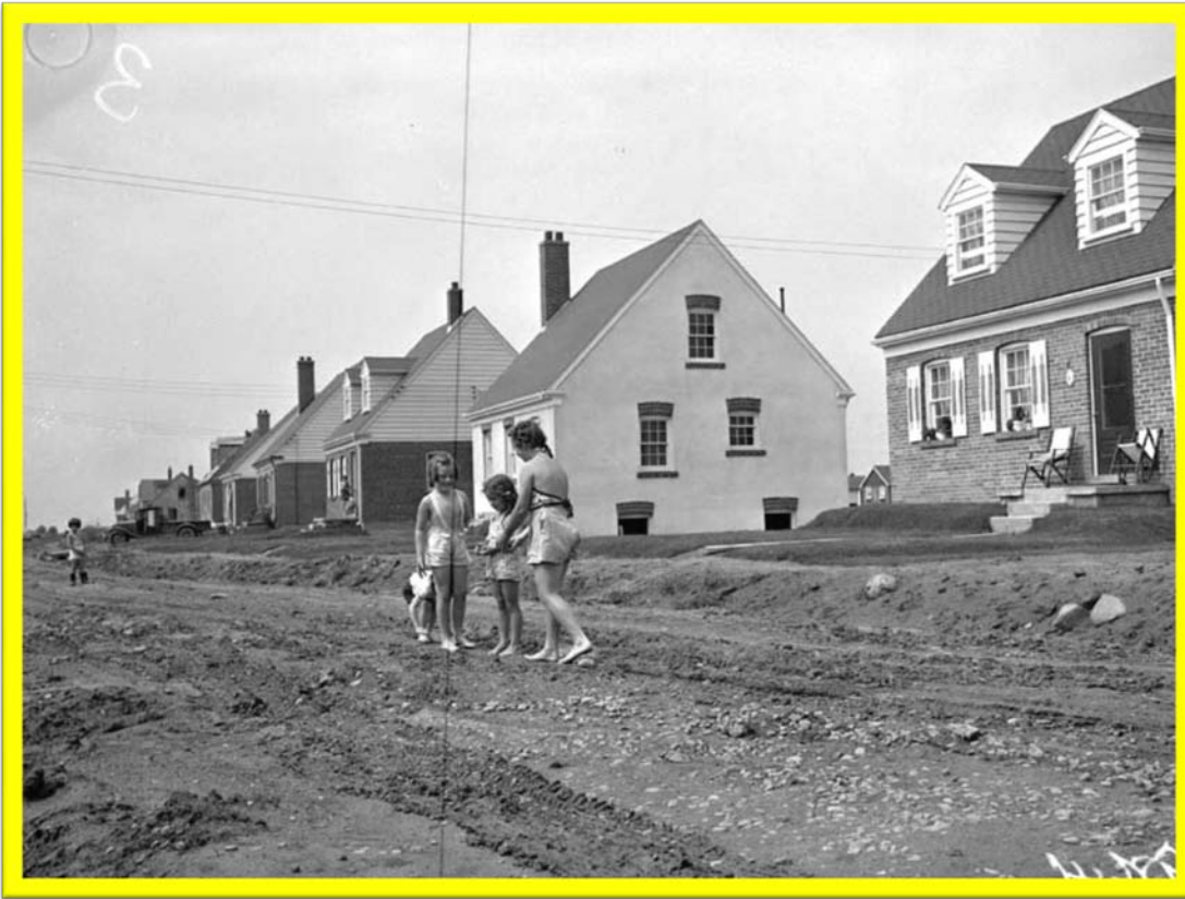
Figure 14: Similar streetscape view of north Toronto’s Winston Park shortly after the houses were built but before completion of the road (with gravel surface) or any sidewalks and front walkways. This post-war subdivision, now located just north of the 401, was clearly built with permanence in mind. It mainly consisted of 1 ½ dwellings, which appear to have been constructed with full basements and heated with coal boilers as indicated by the chimneys. A number of these houses are still standing with the usual alterations and additions made over time. The Winston Park area with its wide roadways and generous setbacks still retains its sense of spaciousness (as observed on Google street view).
