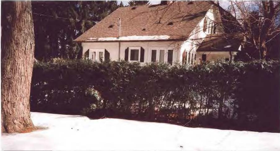
North West View
