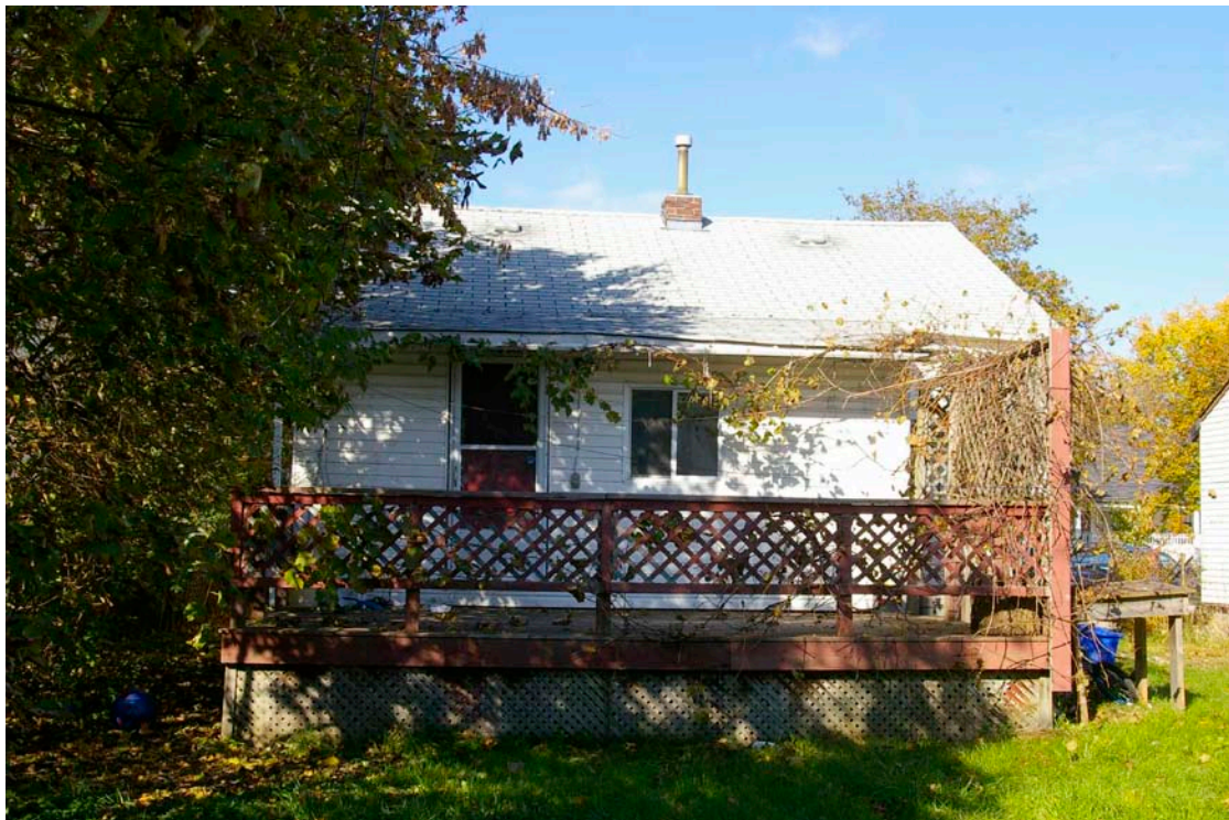
Photo 22: Rear facade showing the shallow addition with a doorway onto a wood deck extending the width of the addition. The chimney for the existing furnace appears to be in the same location as originally constructed for a coal burning stove.
