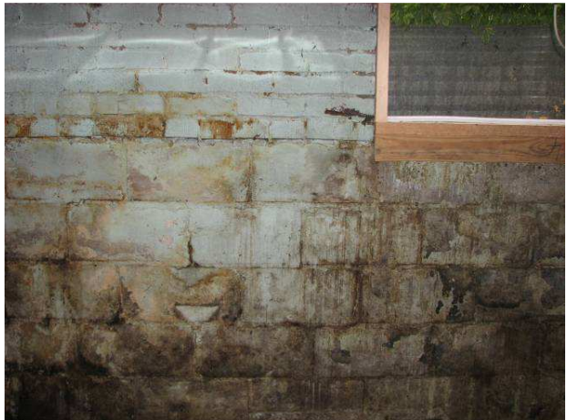
Figure 21. Foundation wall: Block below, brick above.
