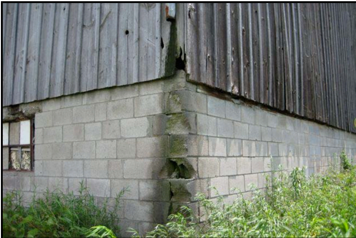
Plate 17: Detail North West Corner of Barn- Deteriorated Foundation & Board
