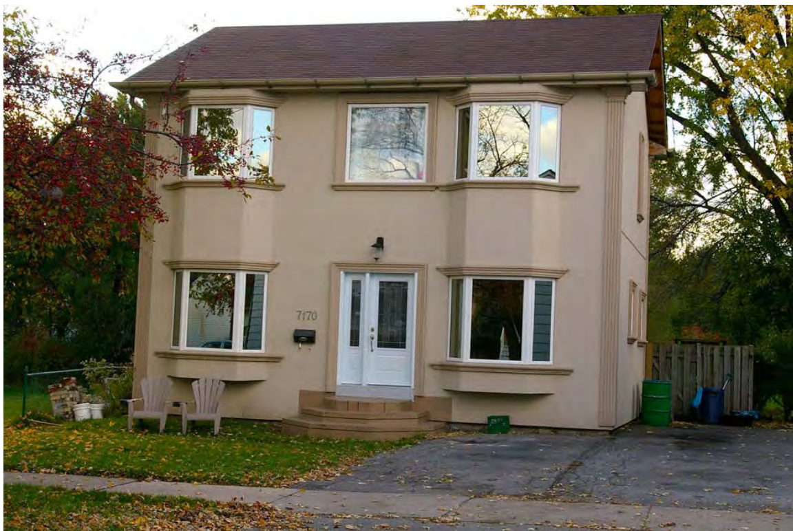
Photo 11: Original bungalow (shown above) at 7170 Lancaster Avenue, altered circa 2011-12 by a second storey addition and a one-storey rear addition (CM> Property Information > Building Permits). Front facade features four bay windows, a front entrance with a glazed door and sidelight and stucco facing with traditional mouldings.
