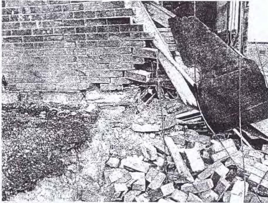
C) Foundation damage.
