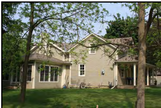
7050 Second Line West, view from the southeast. The indent in the wall between the “V” in the roofline indicates the distinction between the front original portion of the house and the rear addition.
