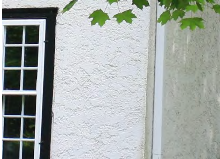
A good example of rough cast stucco.
