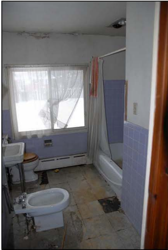
MAIN FLOOR BATHROOM (NOTE WATER DAMAGE)
