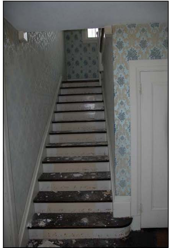
MAIN FLOOR STAIRS (NOTE FALLING PLASTER)
