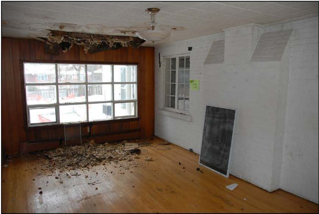
SITTING ROOM (NOTE COLLAPSING CEILING)
