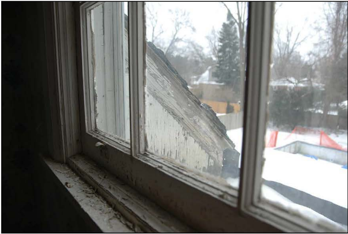
DETERIORATION OF OUTSIDE TRIMWORK
