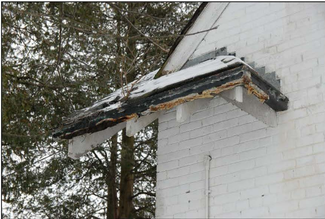
TYPICAL TRIM CONDITIONS (NOTE EXPOSED RAFTER, GENERAL DETERIORATION)
