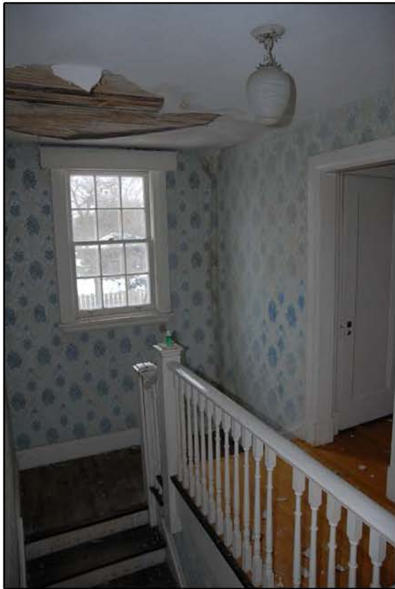
TOP OF STAIRS (NOTE COLLAPSING CEILING)
