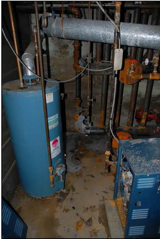
BASEMENT PIPING (NOTE RUST FROM WATER DAMAGE)
