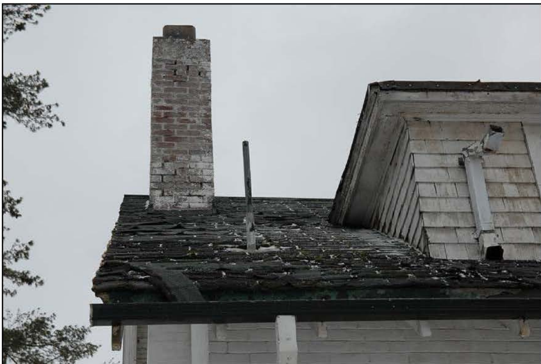
DETERIORATION OF ROOF, CHIMNEY
