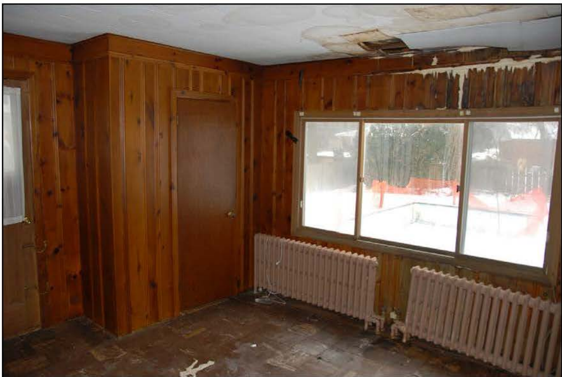
FAMILY ROOM (NOTE COLLAPSING CEILING)
