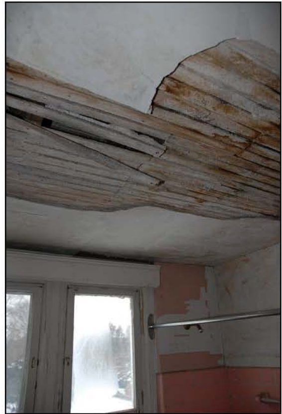
SECOND FLOOR BATHROOM (NOTE COLLAPSING CEILING)
