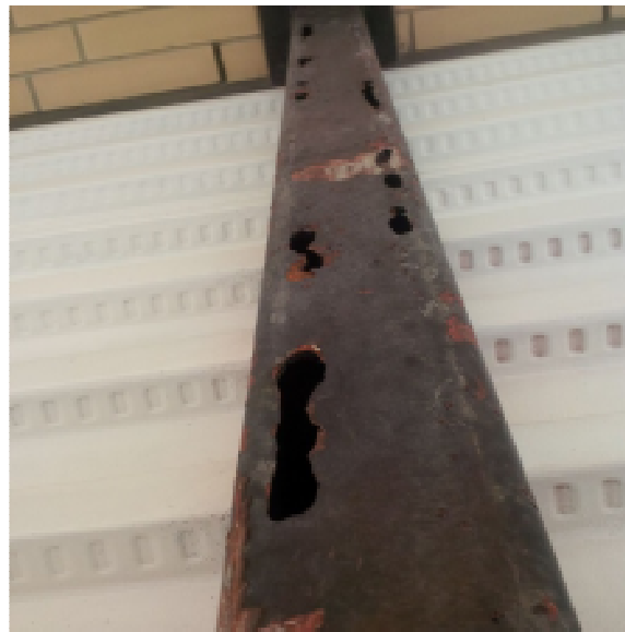
Rusting structural supports at City Hall
