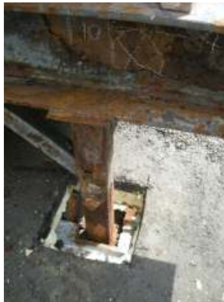
Deteriorating mechanical unit support at Iceland Arena
