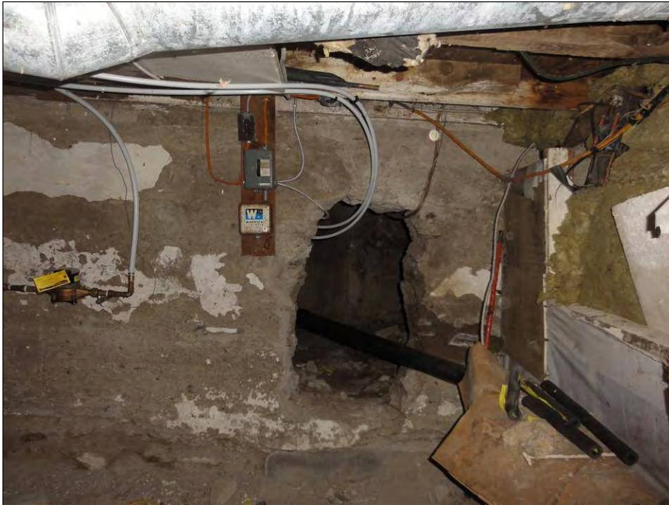
Plate 27: Gap in concrete wall at west end of rear basement, providing access to area underneath the laundry room and bathroom.
