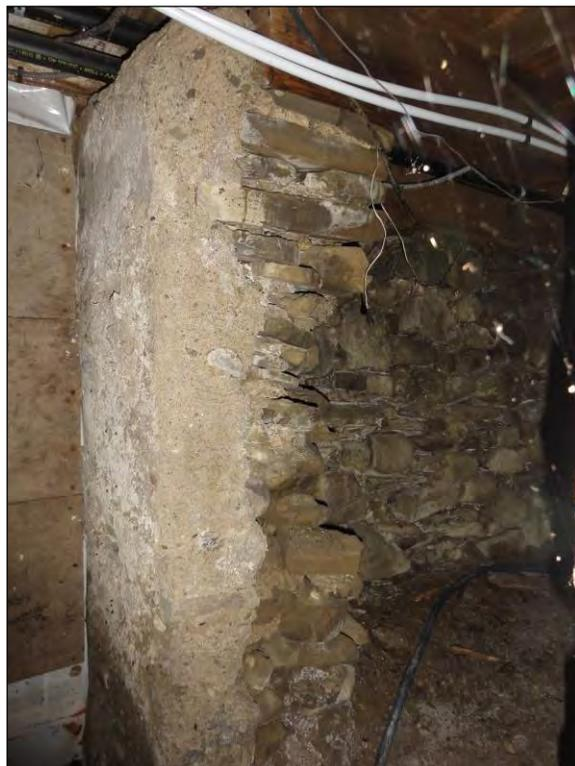
Plate 28: Gap in wall in southeast corner of rear basement, providing access to original cellar underneath the east part of the kitchen. Note the fieldstone material reinforced by concrete.
