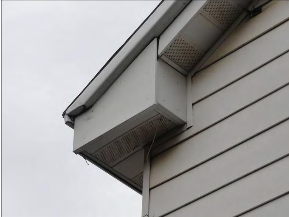
Plate 13: Detail of return eaves, soffit, and siding, showing synthetic materials.
