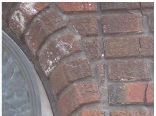
19. Detail cracked brick units on west elevation. (ERA)
