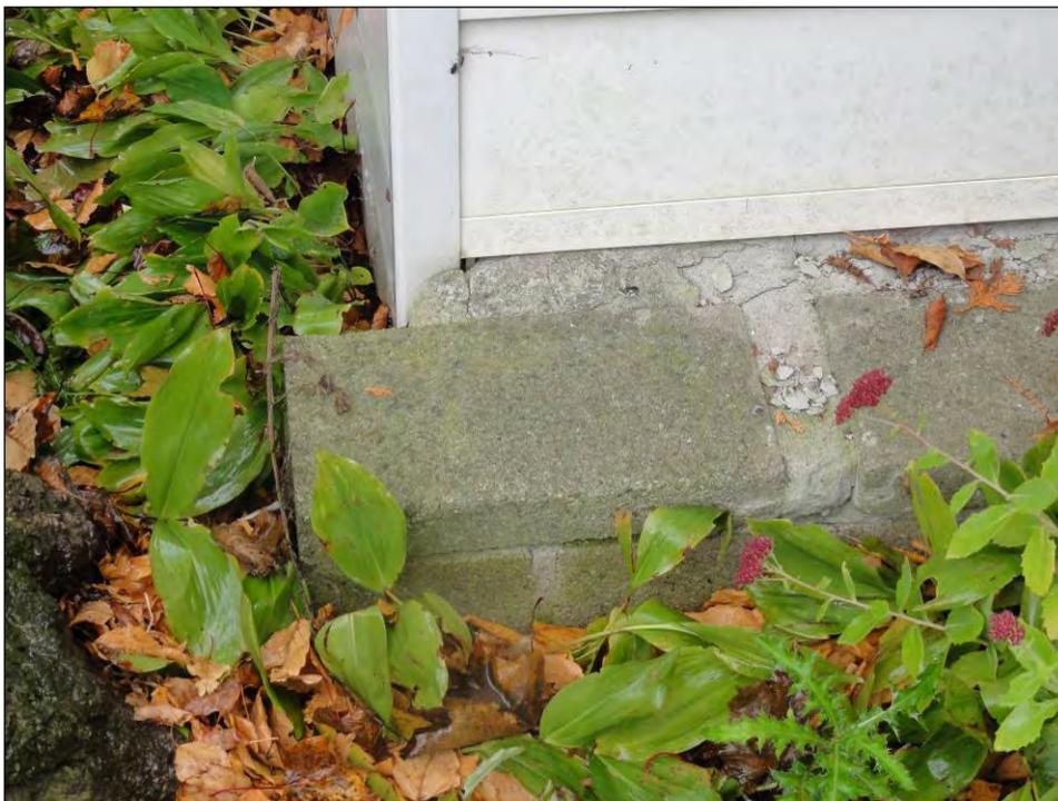
Plate 10: Concrete wall concealing foundations on east elevation at south corner.
