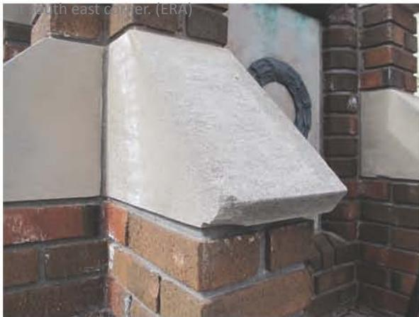
16. Detail chipped sandstone buttress cap. (ERA)
