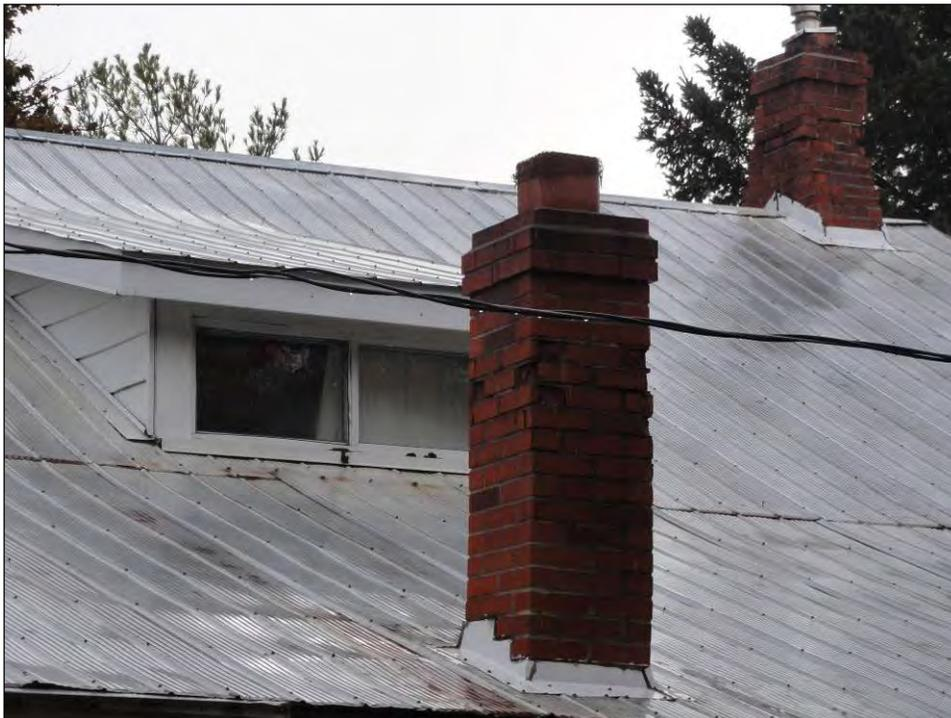
Plate 12: Metal roofing of main house, brick chimney stacks, and rear dormer.
