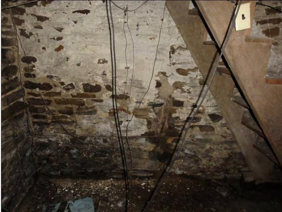
Plate 37: North wall of front basement and view of wooden stairs. Note the tree stump or root in wall.
