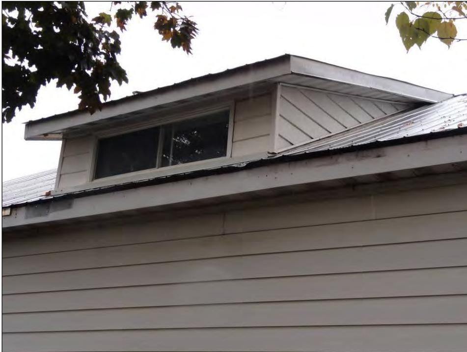
Plate 19: Shed dormer on front elevation.
