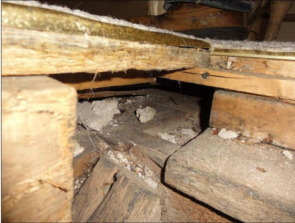
Plate 33: Detail of gap between new floor and original floor underneath.
