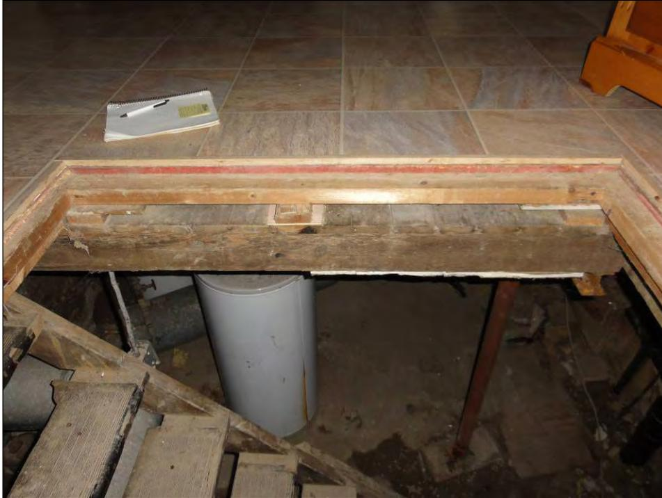
Plate 25: Looking down through trap door in rear addition. Note that the current tiled floor has been laid overtop of the original wooden floors.
