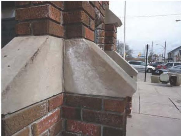
14. Detail efflorescence on sandstone
