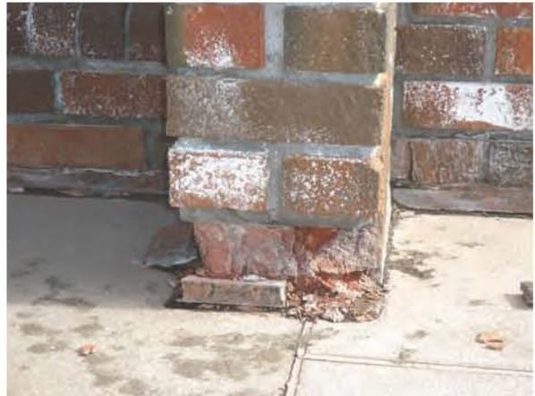
15. Detail spalled brick at base. (ERA)
