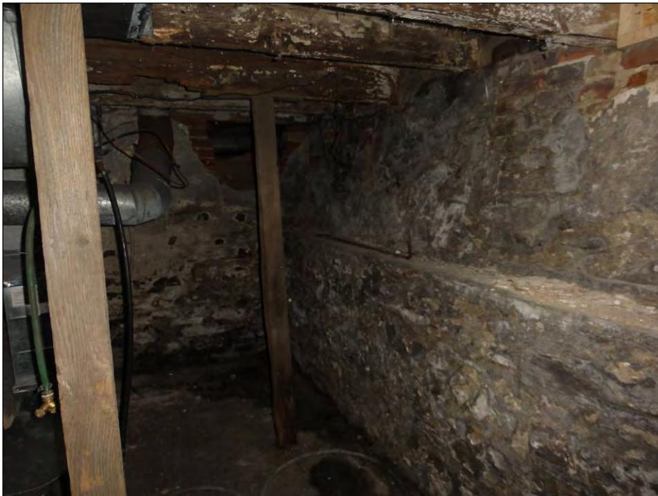
Plate 36: View of south wall, looking east, showing field stone walls and brick repairs.
