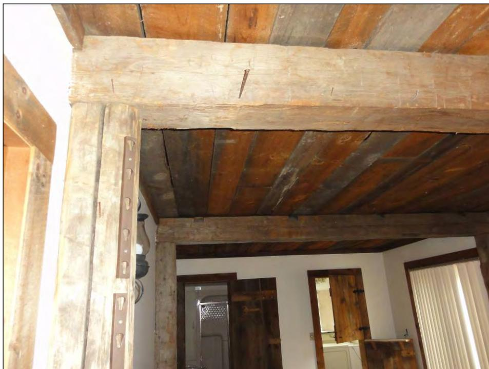
Plate 46: Detail of reclaimed posts, beams and boards used to construct and decorate the family room.
