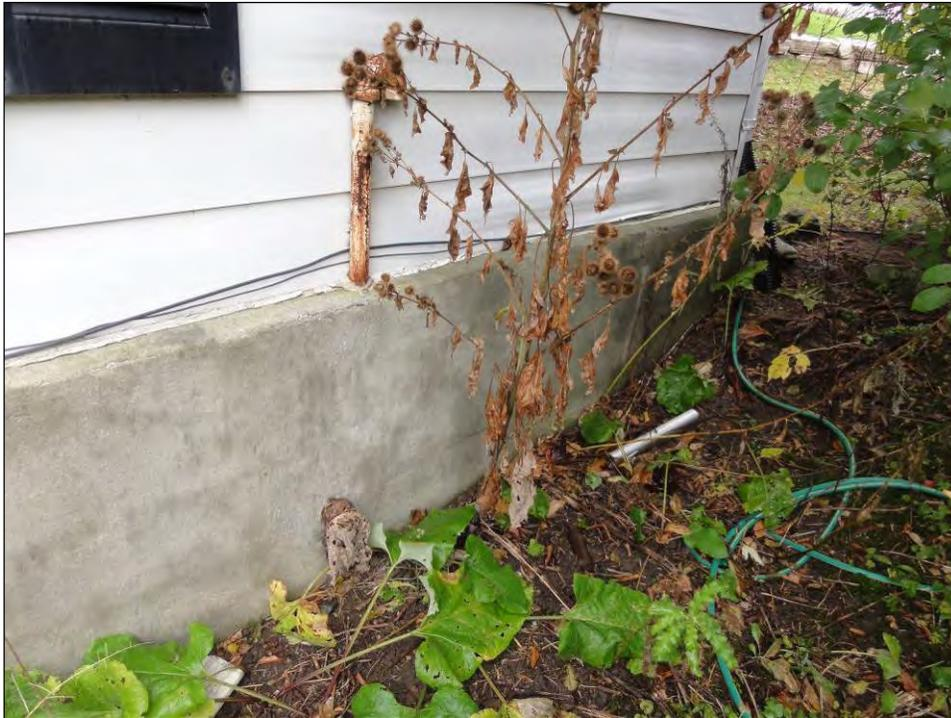
Plate 9: West foundations parged with concrete.
