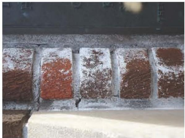
17. Detail, efflorescence on brick, south elevation. (ERA)
