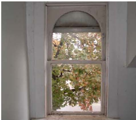
Sash window on second floor has a arched top sash. It is hidden from view on the exterior by an aluminum window.
