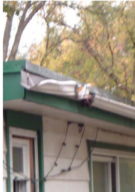
The eavestrough on the one story addition at the back is damaged.
