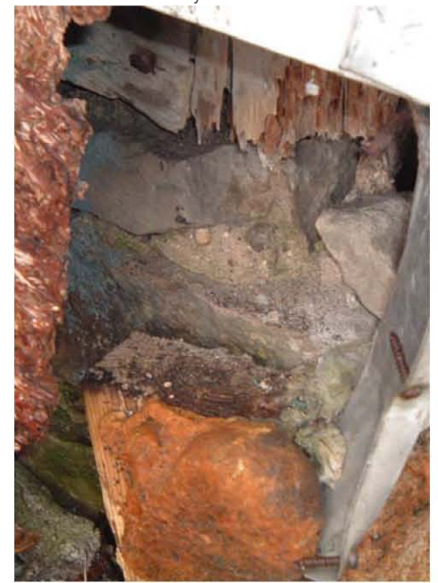
Where the aluminum cladding and chipboard materials have been pulled away in some locations around the base of the building a rubble stone masonry wall can be seen.
