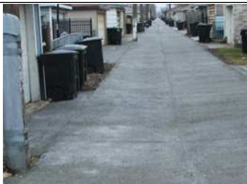
Pervious concrete applied to an alleyway in Chicago (Source: City of Chicago)
