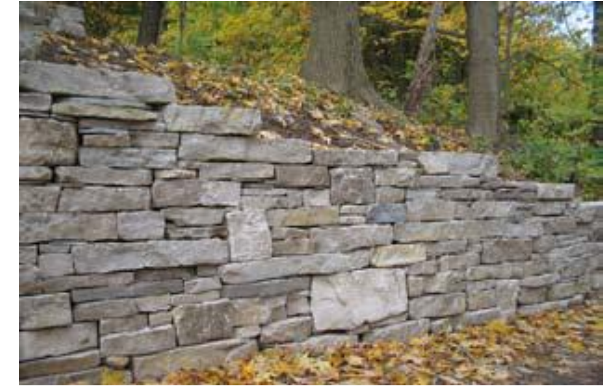
Natural stone retaining walls
