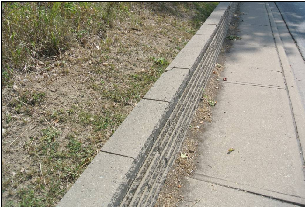
Plate 17: Detail of the concrete block slope protection.
