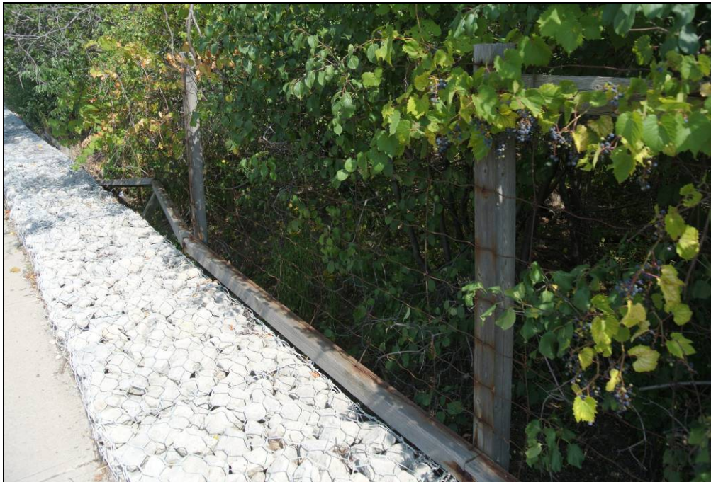
Plate 15: Detail of gabion slope protection located sporadically along the southwestern border of the study area.
