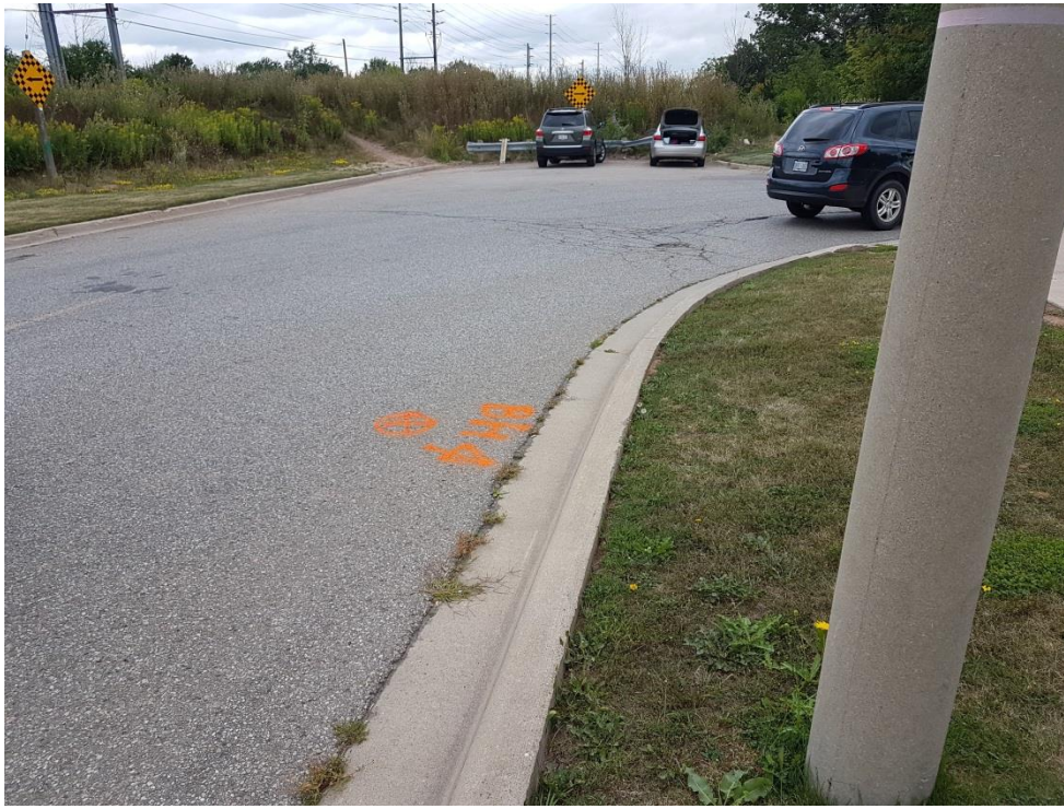
Photograph 5: Distortion from frost heaving near BH4.
