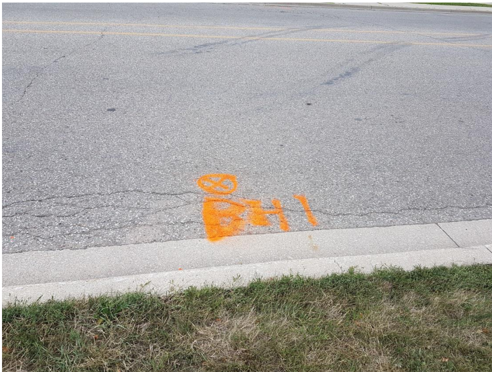
Photograph 6: Longitudinal and transverse cracks near BH1.
