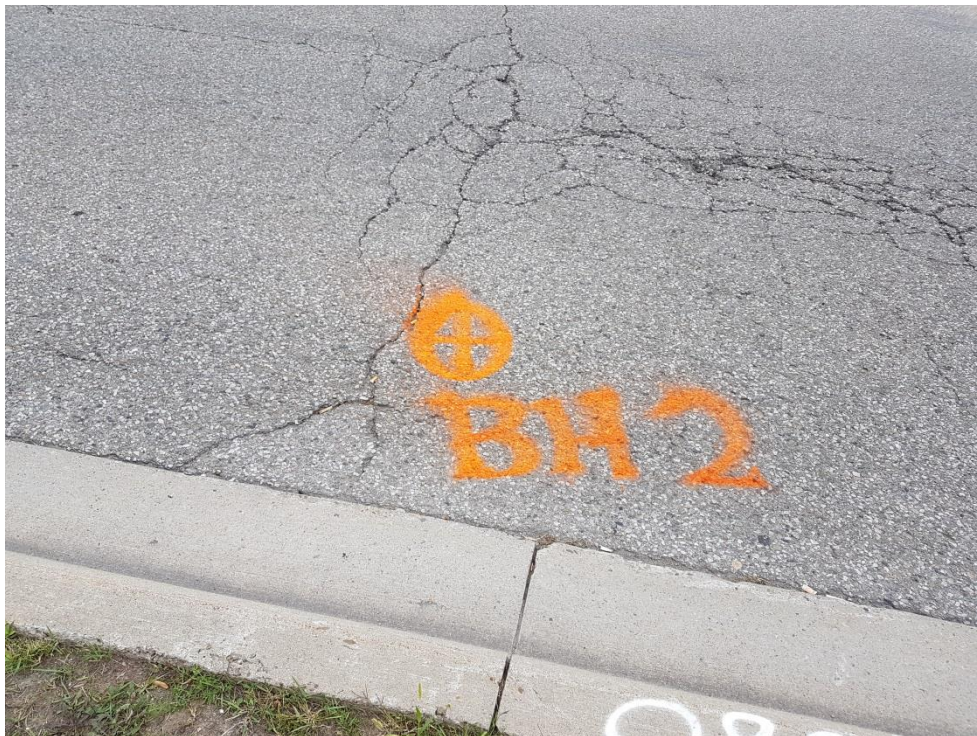
Photograph 4: Severe distortion from frost heaving near BH2.
