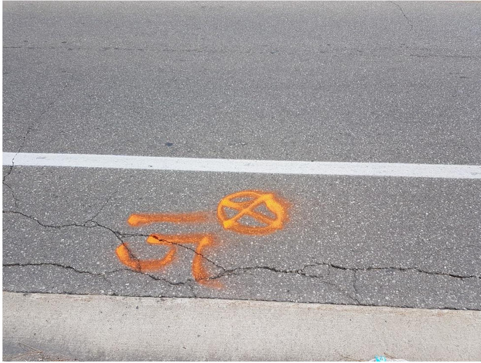
Photograph 11: Wheel track crack at north and longitudinal crack along curblin near BH15.
