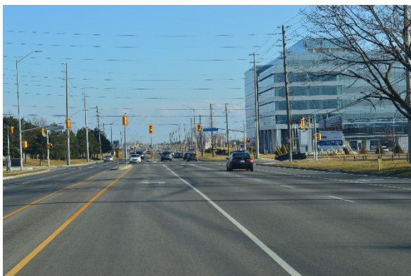
Winston Churchill Blvd is a four-lane arterial with a posted speed 60km/h. There is a gentle slope SB towards the Sheridan/ Plymouth intersection
