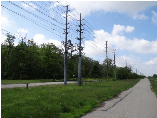
Plate 7: Termination of Sheridan Park Drive at the east portion of the study area, looking southwest.
