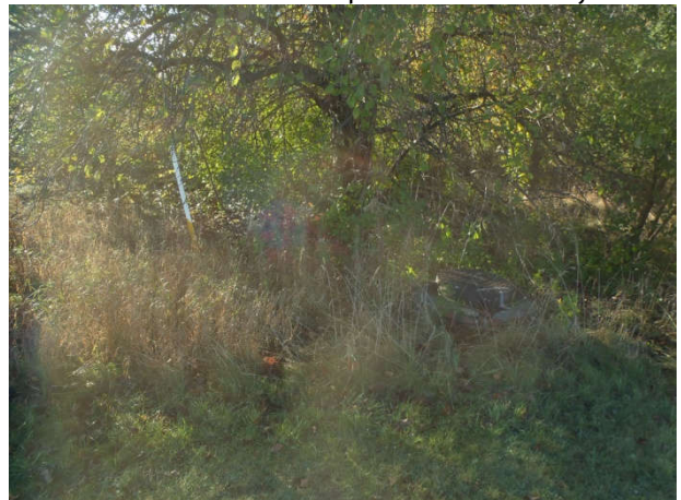
Plate 22: View S at buried gas pipeline and utility access cover at the intersection of Sheridan Park Drive and the east leg of Speakman Drive.
