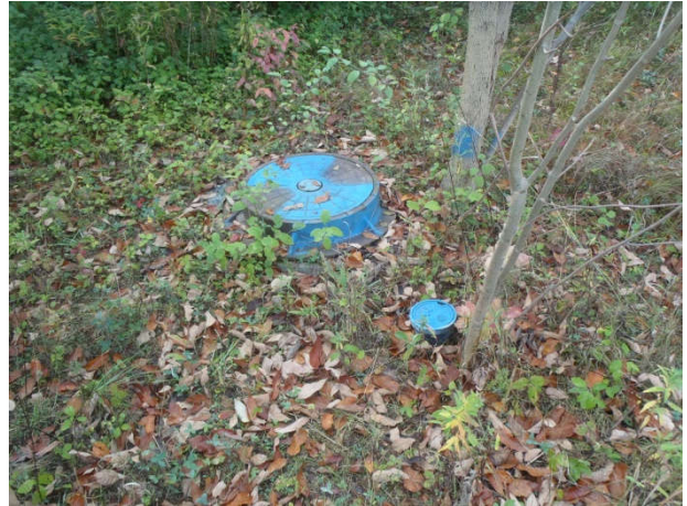
Plate 18: View SE utility access covers in the eastern portion of the study area.
