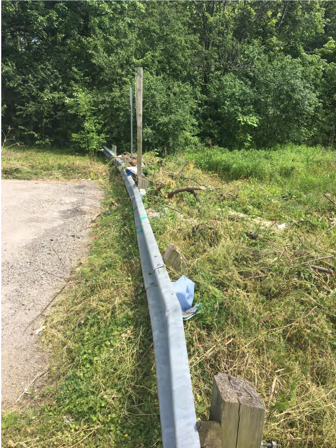
Photo 2: Road barrier at Sheridan Park Drive at east end of Site.
