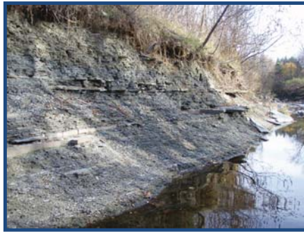
Cooksville Creek – Bank Erosion
