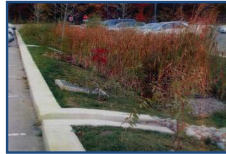
Bio-retention Facility To Treat Parking Area
