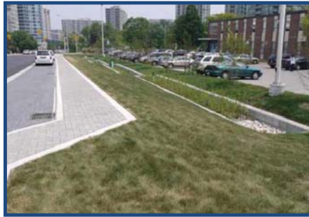
Bio-retention Facility To Treat Roadway Drainage
