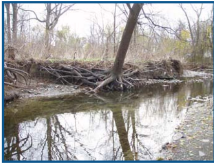
Cooksville Creek – Bank Erosion
