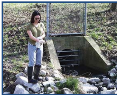
Inspection of Outfall
