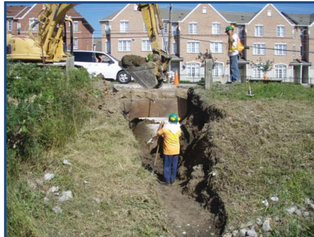
Storm Sewer Reconstruction
