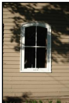
Detail of east façade window
