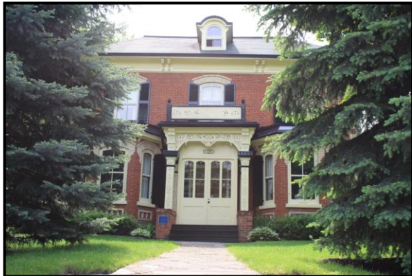
Graham-Pearson House, front, north elevation.
