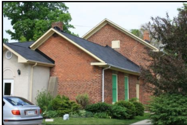
Meadowvale United Church, rear and east façades
