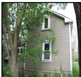
7004 Second Line West, south façade.
