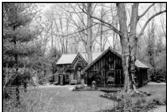
1101 Willow Lane, out buildings (photo: Heritage Mississauga)
