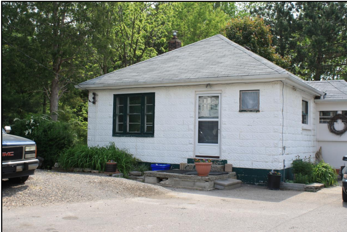
Concrete block residence at 1056 Old Derry Road
