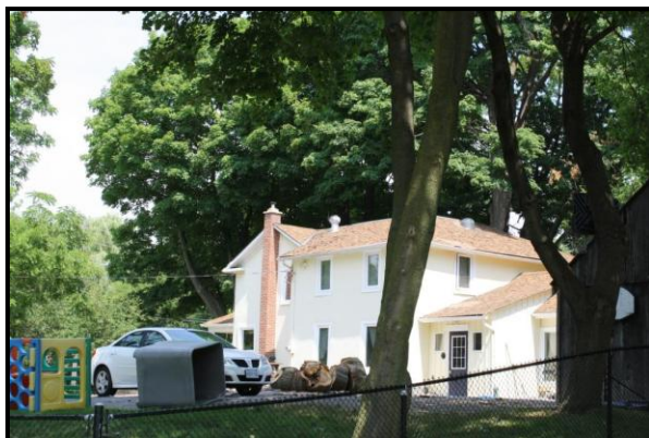
1100 Old Derry Road West, west elevation
