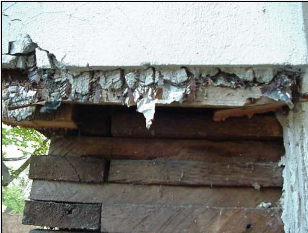
1101 Old Derry Road - Note the stacked plank construction on the lower half of the structure. The upper floor has been modified from the original structure.
