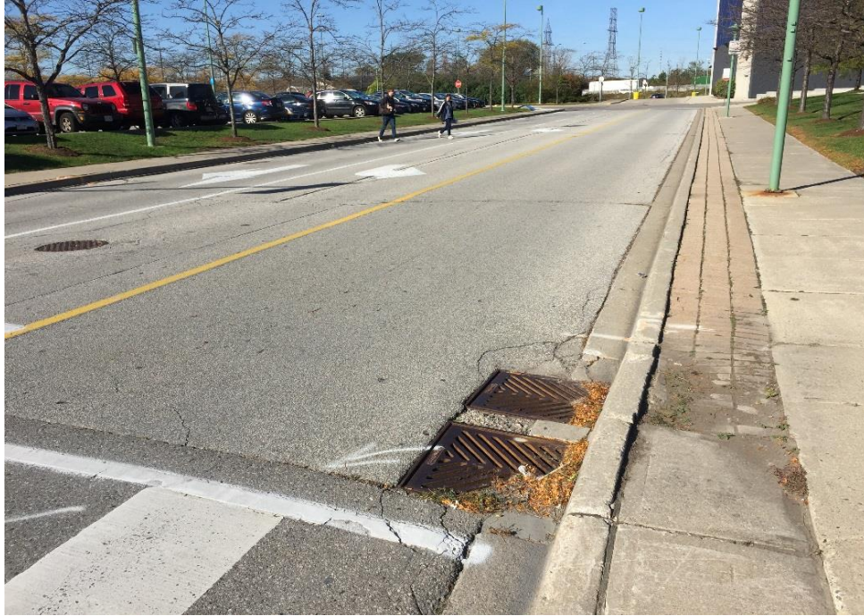
Photograph 1 – Existing Access Road/future Extension of Living Arts Drive, westbound lane, at the intersection of Rathburn Road West, looking west, showing moderate construction joint cracking, moderate longitudinal and transverse cracking. Catch basin was in fair condition with slight alligator and random cracking around it.
