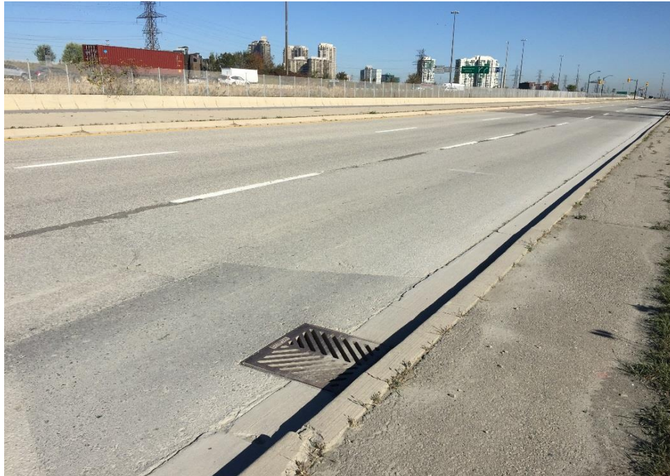
Photograph 8 – Centre View Drive, eastbound lane, at the proposed intersection with Living Arts Drive, showing slight edge cracking, slight longitudinal and transverse cracking (partially sealed) and slight cut patching. Catch basin was in fair condition.
