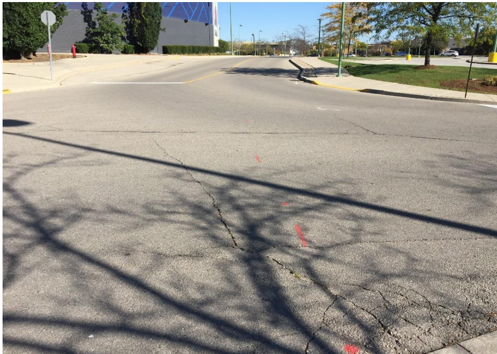
Photograph 6 – Existing Access Road/future Extension of Living Arts Drive, about 160 m west of Rathburn Road West, looking east, showing moderate longitudinal and transverse cracking associated with alligator cracking.
