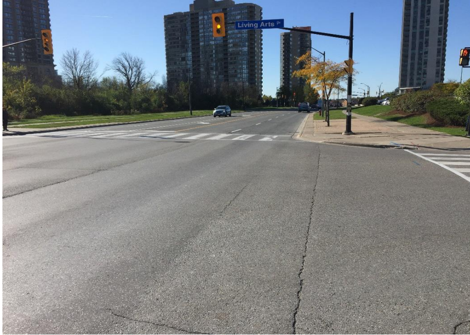
Photograph 7 – Rathbun Road West, at the intersection of Living Arts Drive, looking south, showing slight to moderate longitudinal and transverse cracking.
