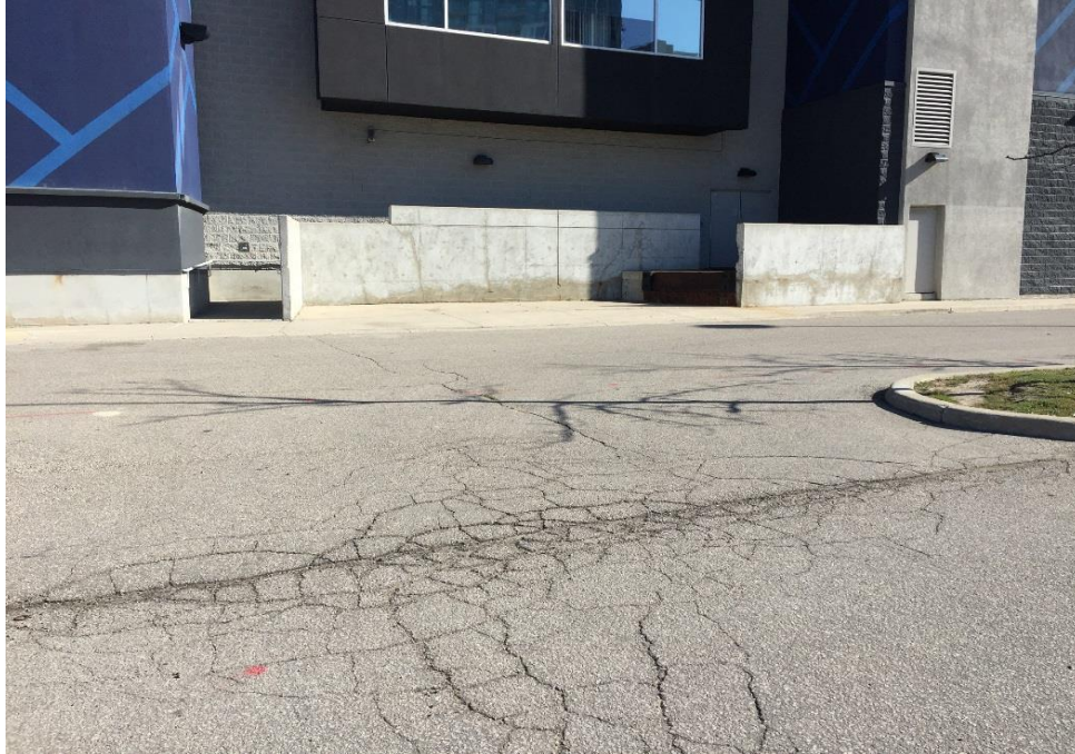
Photograph 5 – Existing Access Road/future Extension of Living Arts Drive, south of the theater, about 140 m west of Rathburn Road West, looking north, showing moderate longitudinal and transverse cracking associated with slight to moderate alligator cracking and.
