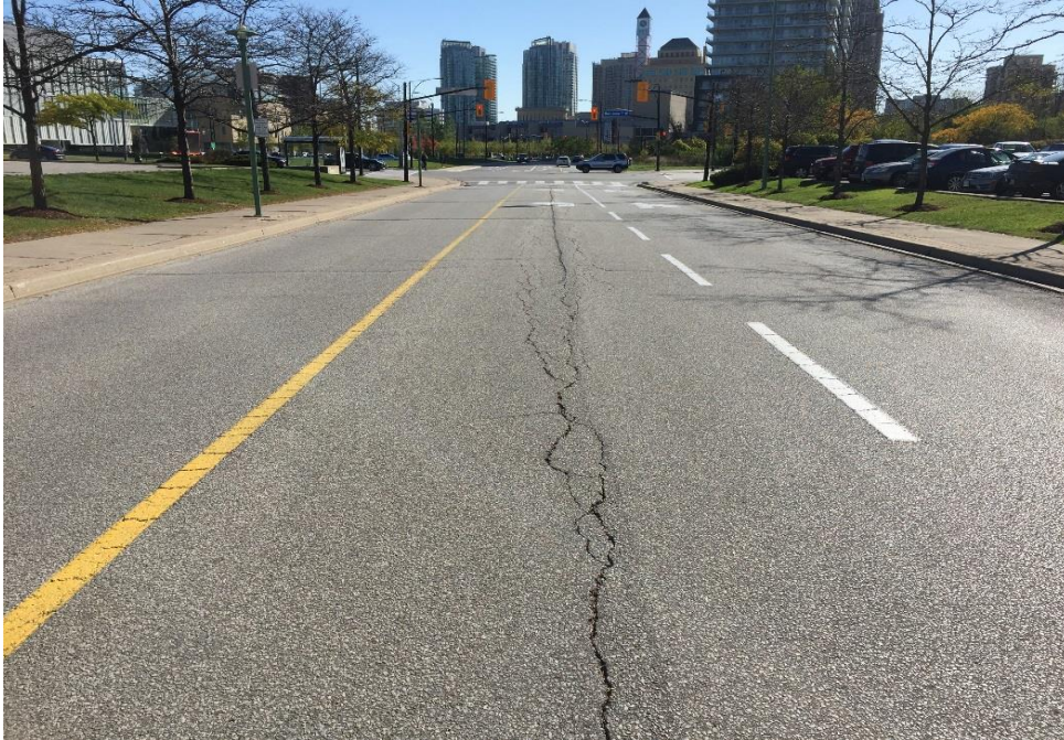
Photograph 3 – Existing Access Road/future Extension of Living Arts Drive, eastbound lane, about 50 m west of Rathburn Road West, looking east, showing moderate longitudinal cracking associated with slight to moderate alligator cracking and slight to moderate transverse cracking.
