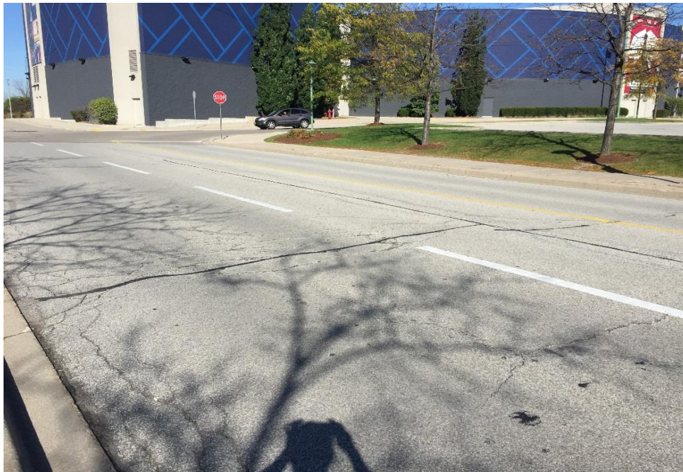
Photograph 4 – Existing Access Road/future Extension of Living Arts Drive, eastbound lane, about 45 m west of Rathburn Road West, looking west, showing moderate edge cracking associated with alligator cracking, slight to moderate longitudinal and transverse cracking (partially sealed).
