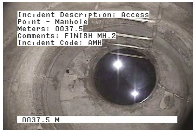
AMH - Access Point - Manhole @ 37.5 m. FINISH MH.2
