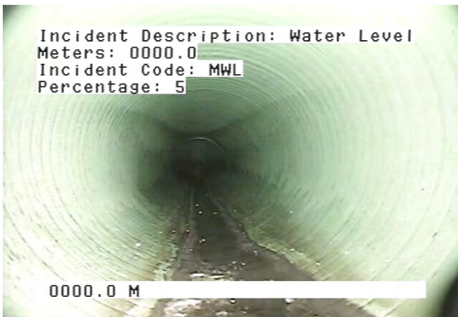
AMH - Access Point - Manhole @ 11.6 m. FINISH MH.8
