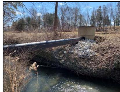
B. Slumping gabion baskets undermining and scouring around chamber structure.
