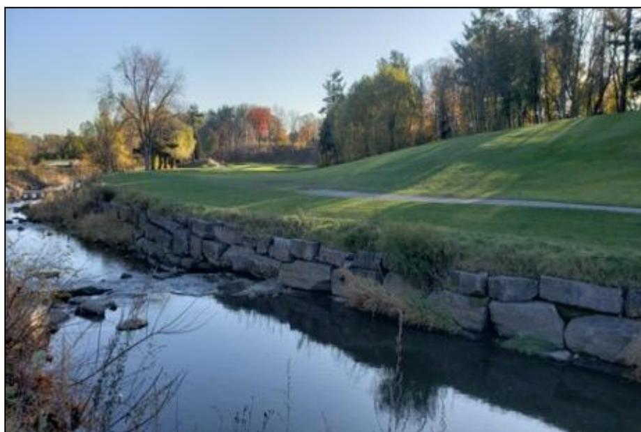
Figure 4-4. An Example of Engineered Channel Restoration with Armourstone.
