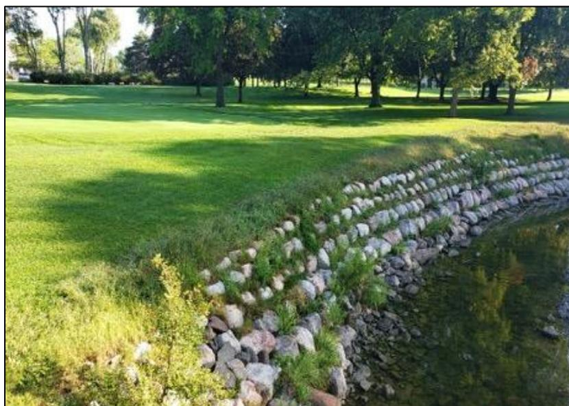
Figure 4-6. An Example of Engineered Channel Restoration with Vegetated Roundstone.
