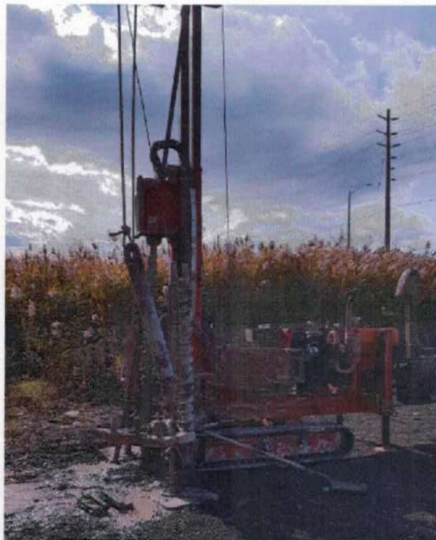
The drilling equipment
