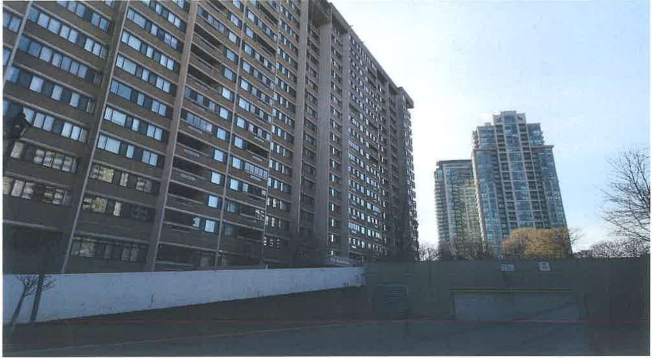
Residential building to South of subject site (looking Southwest)
