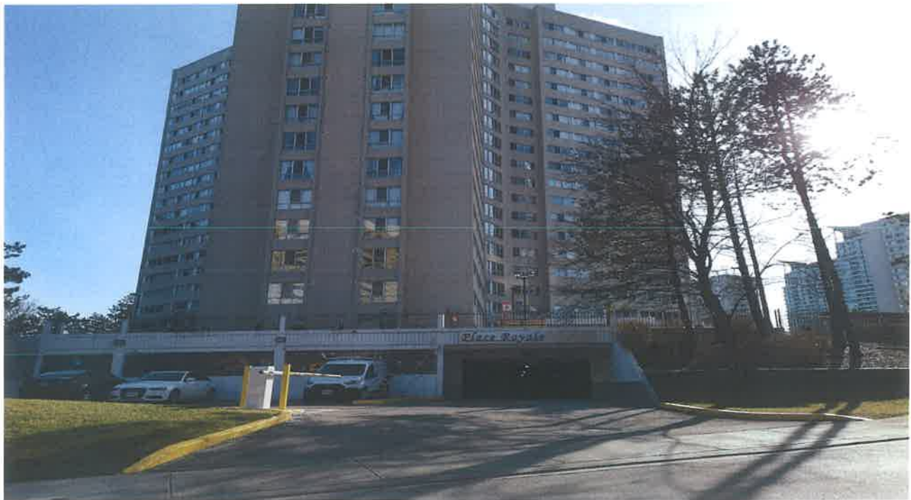
Residential building to Northwest of subject site (looking Southeast)
