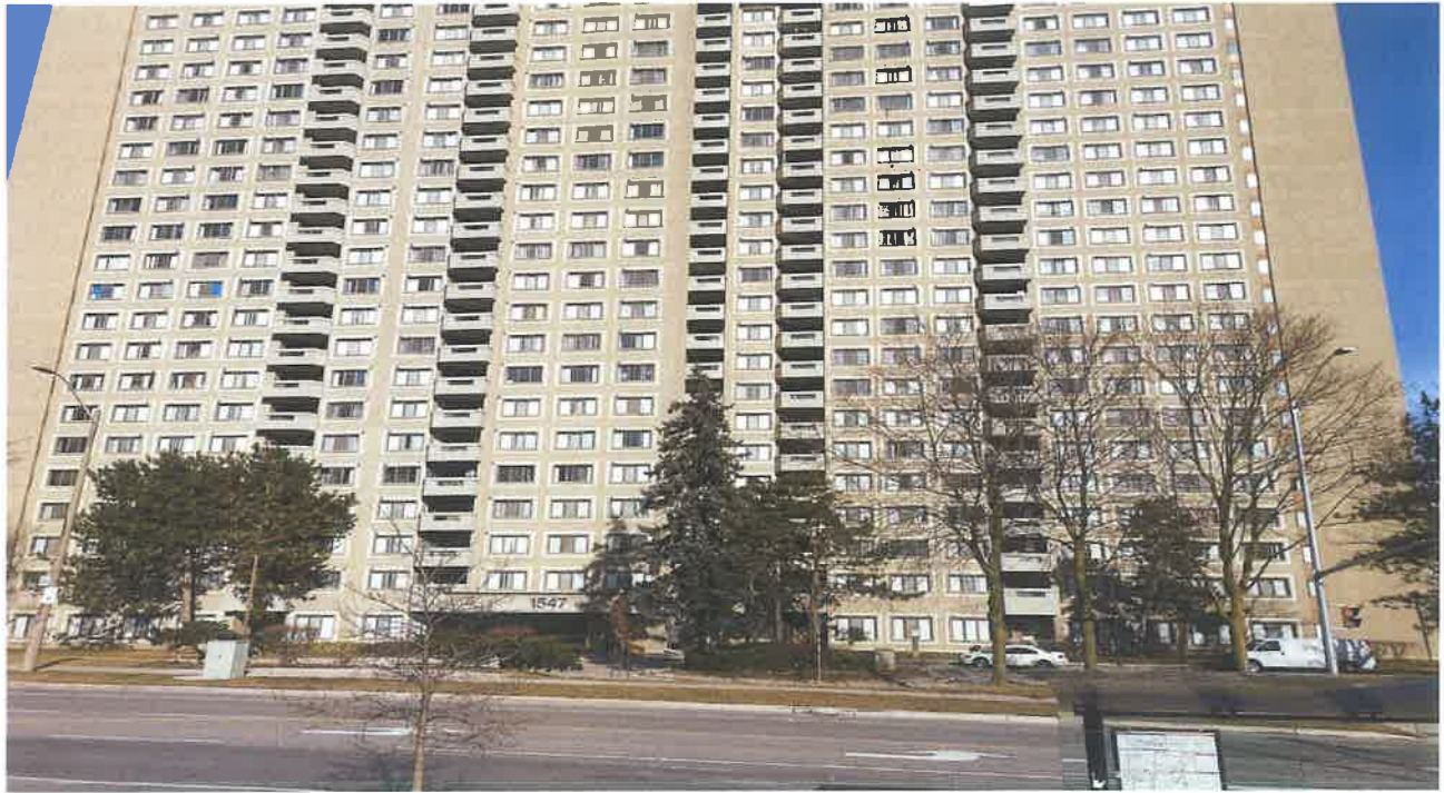
Residential building to Northeast of subject site (looking Northeast)
