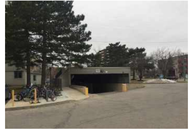
1840 Bloor Street below-grade parking ramp
