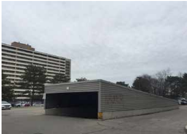
1850 Bloor Street below-grade parking ramp
