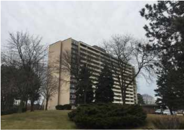
1900 Bloor Street looking south from Bloor Street
