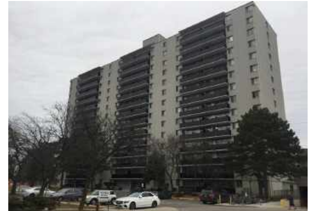
Subject site: 1840 Bloor Street West looking southwest
