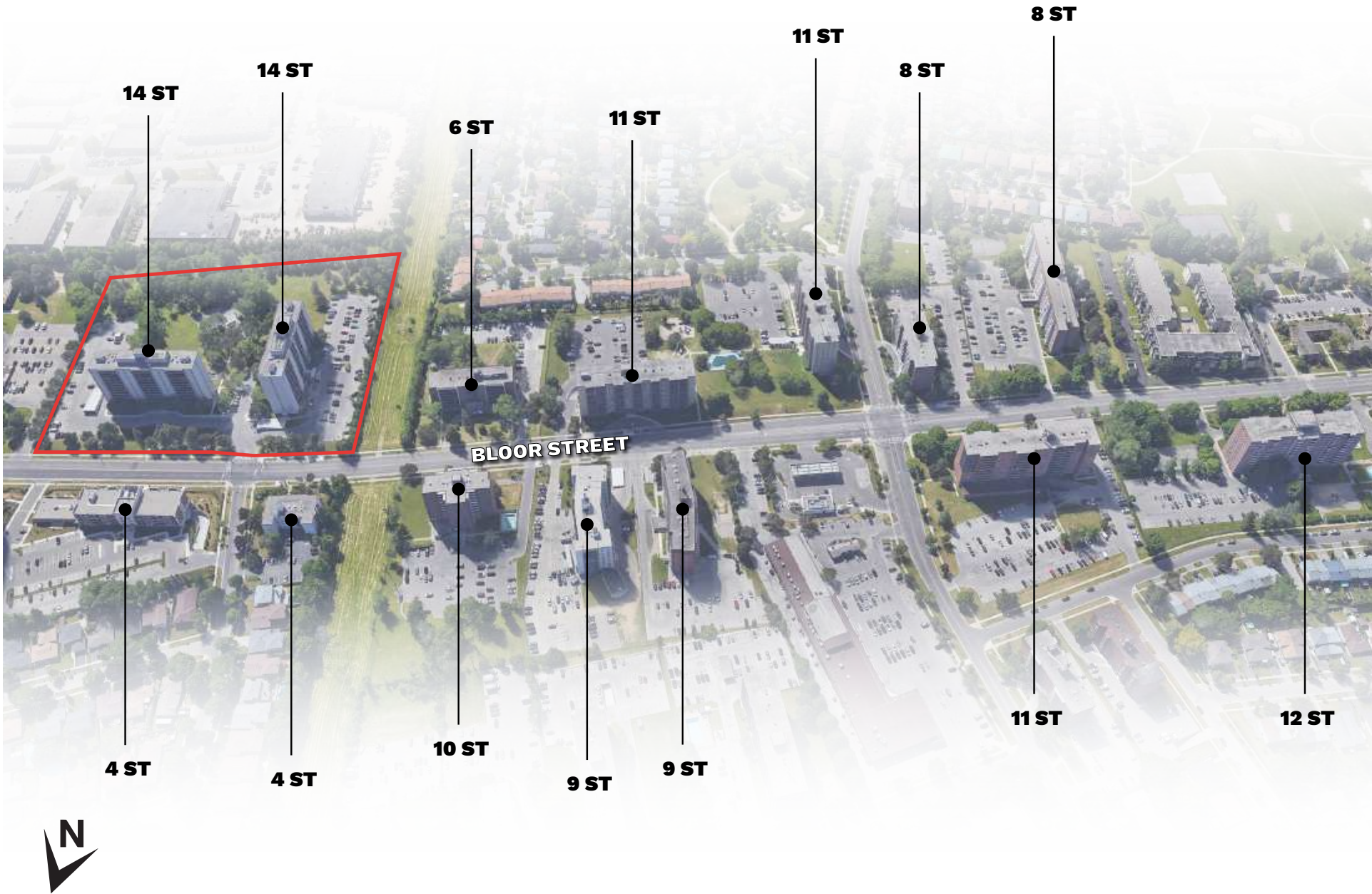
Figure 4 - Highrise Buildings in the Immediate Context West of Site
