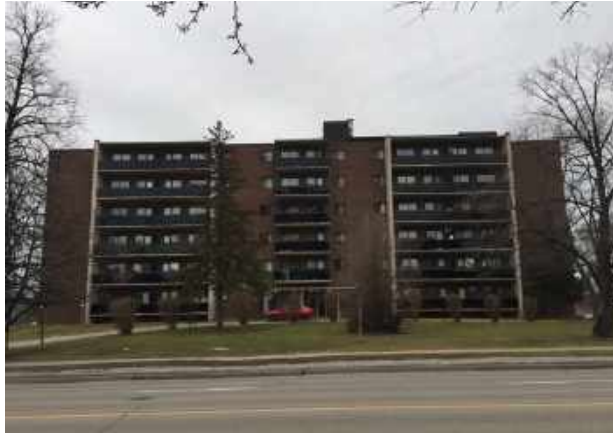
1780 Bloor Street looking south from Bloor Street
