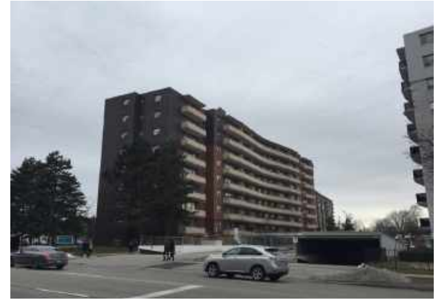
1745 Bloor Street looking north from Bloor Street
