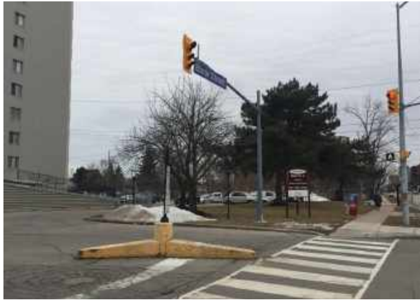
Driveway access at Bloor Street and Bridgewood Drive
