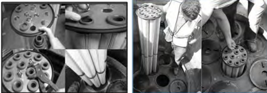
Assembly of a Jellyfish Filter cartridge (left) and installation of a filter cartridge into a cartridge receptacle in the deck (right).
