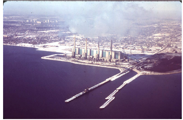
Fig. 15 Ralph Crysler, "Lakeview Generating Station, Aerial View," 1972, City of Mississauga Historic Images Gallery, Lakeview Gallery, LG_R135.jpg. The oblique aerial photograph captures the massiveness of the station with its four smokestacks already covered in soot. Note how the coal conveyor is elevated over the intake channel, which it crosses on its way to the coal yard.
