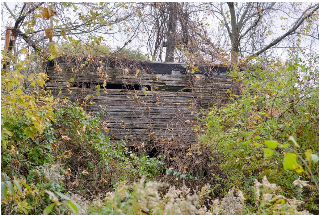
Fig. 65 A severely deteriorated baffle
