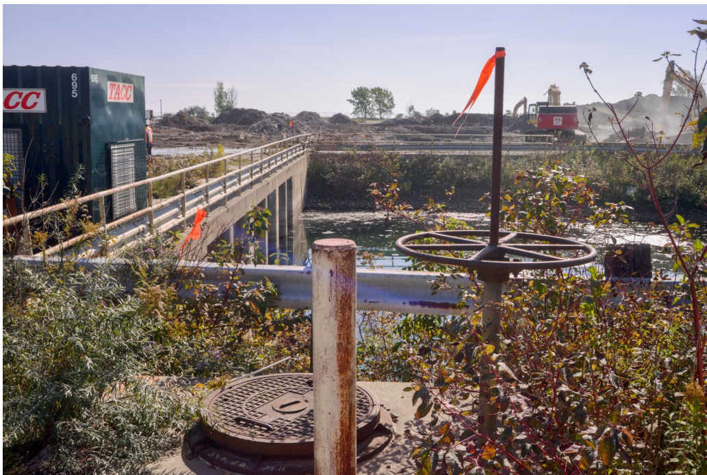
Fig. 29 View of the former station's discharge outlet, looking southward across the discharge channel to land being cleared of concrete rubble. Lake water, heated through the powerhouse, used to empty at the discharge outlet into the discharge channel.
