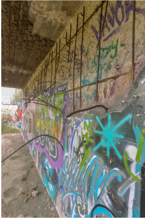
Fig. 70 Detail of spalled concrete and exposed rebar on the backstop's north wall and of damaged wood on the canopy's underside
