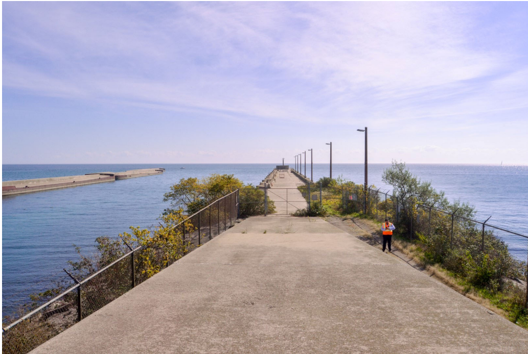
Fig. 34 View on the docking causeway near its north end, looking southward. The docking causeway ramps up steeply near its north end. To the left of the docking causeway is the north-south intake channel. In the far left is the eastern breakwater, which in this view is the part made of concrete-filled steel barges.
