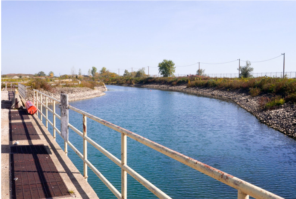
Fig. 32 Exposed intake channel and its sheltered forebay where lake water would have entered the powerhouse. The chain-link fence seen in the background marks the edge of the lake.
