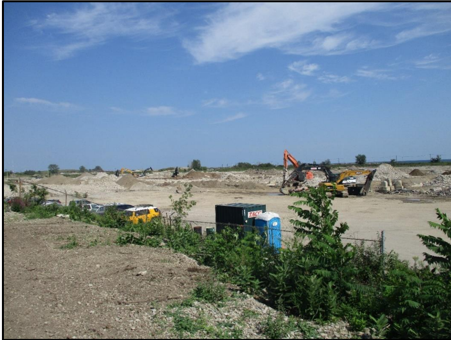
Photograph 2. Anthropogenic Areas under Construction Activity (Unit 2b)
