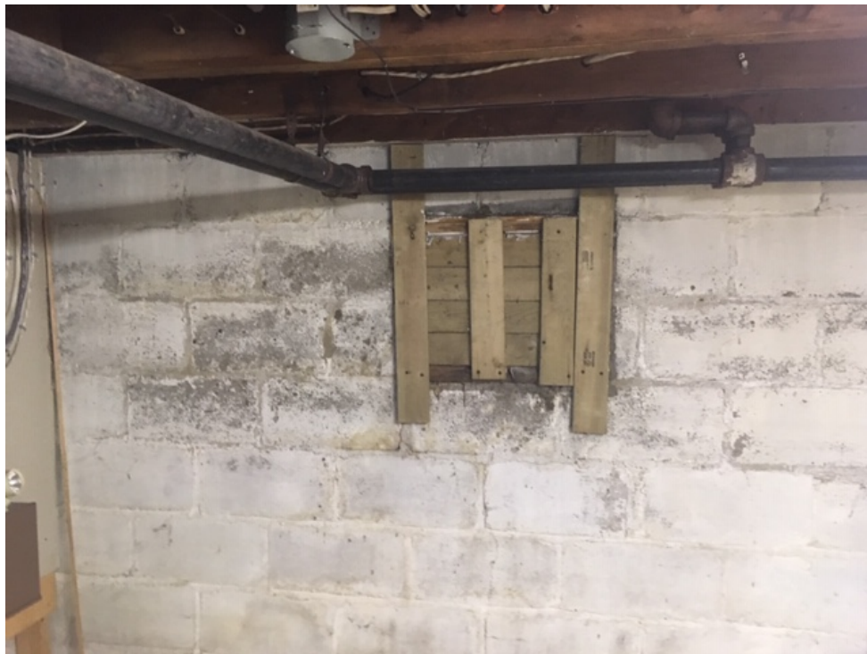
Below: Possible Coal Cellar Hatch with Wood Infill in Basement
