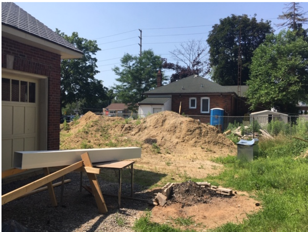
Below: View to West from New Construction
