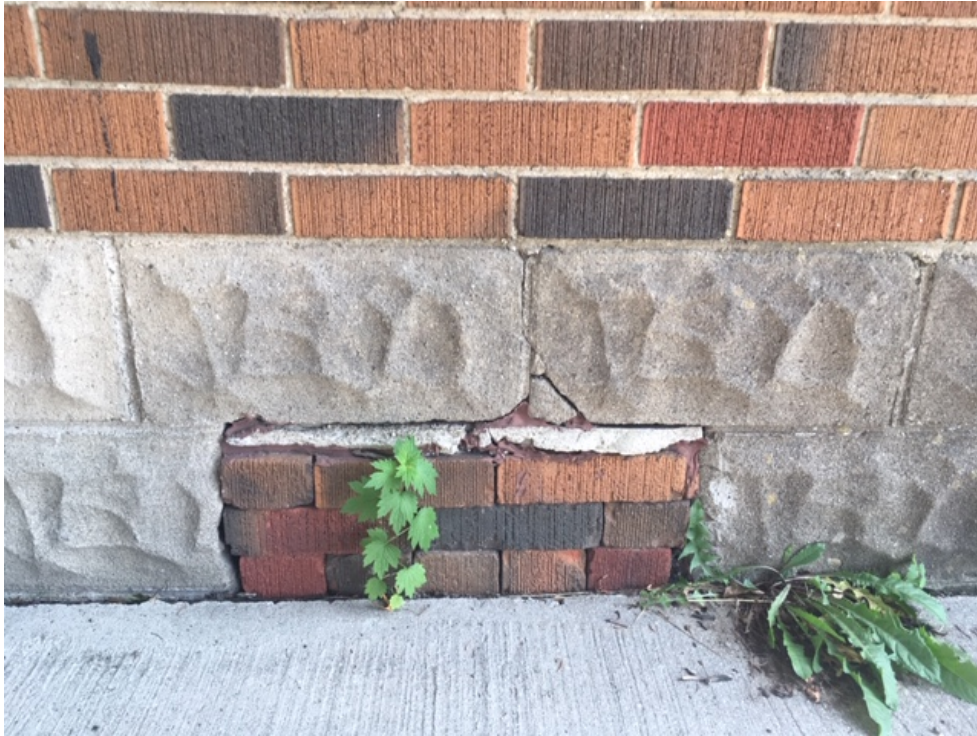
Above: Possible Former Coal Chute (?)
