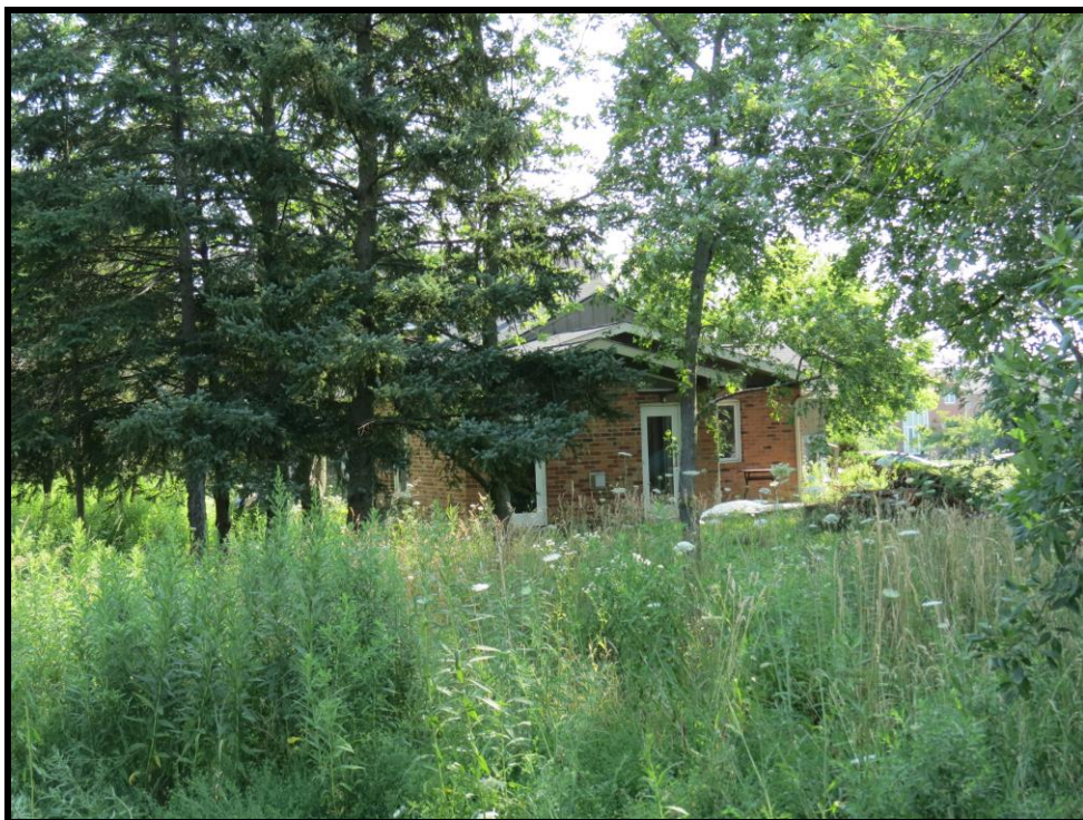
Image 26: South Elevation of 5104 Ninth Line (Photo taken on July 29, 2019; Facing North)
