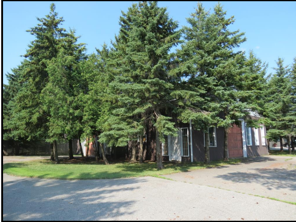
Image 9: Northeast Corner of Garage at 5150 Ninth Line (Photo taken on July 29, 2019; Facing East)
