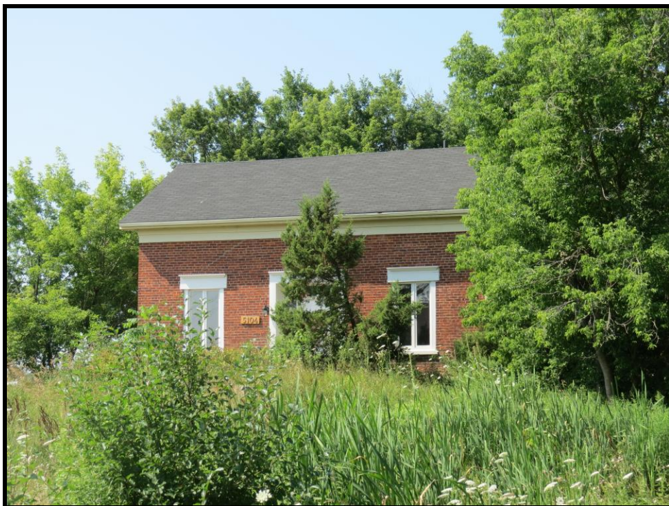
Image 30: Northwest Corner of 5104 Ninth Line (Photo taken on July 29, 2019; Facing South)
