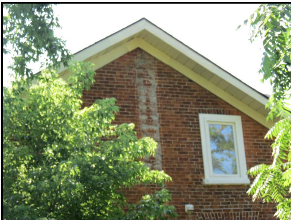
Image 28: Detail of Chimney Ghost, 5104 Ninth Line (Photo taken on July 29, 2019; Facing South)
