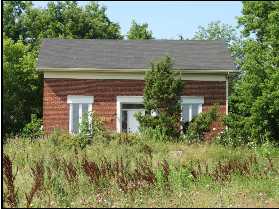
Image 23: Façade of 5104 Ninth Line (Photo taken on July 29, 2019; Facing South)
