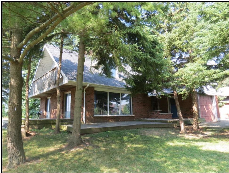
Image 4: Northeast corner of 5150 Ninth Line (Photo taken on July 29, 2019; Facing Southwest)
