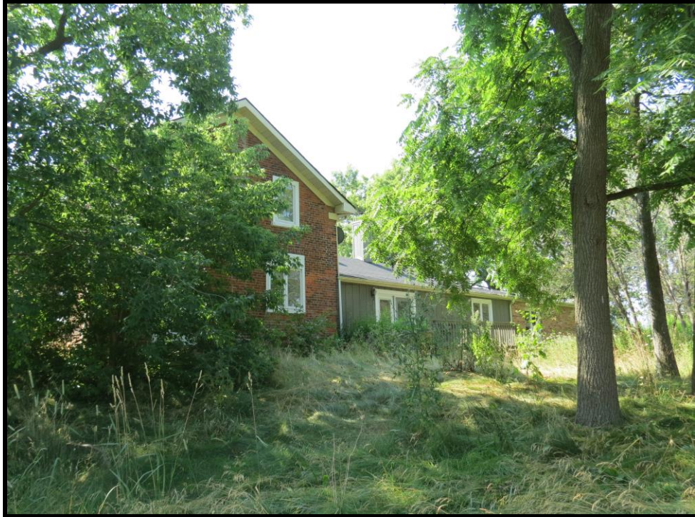
Image 27: West Elevation of 5104 Ninth Line (Photo taken on July 29, 2019; Facing South)
