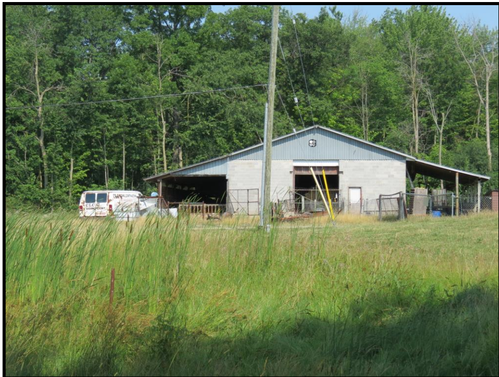
Image 12: East Elevation of Workshop at 5150 Ninth Line (Photo taken on July 29, 2019; Facing West)
