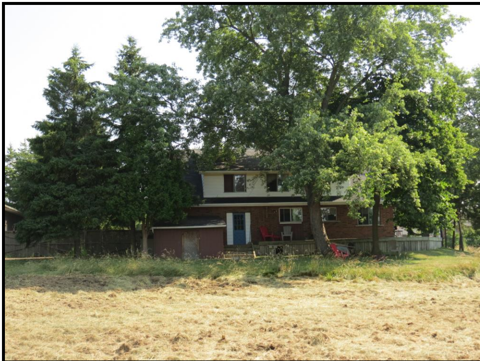
Image 6: South Elevation of 5150 Ninth Line (Photo taken on July 29, 2019; Facing North)
