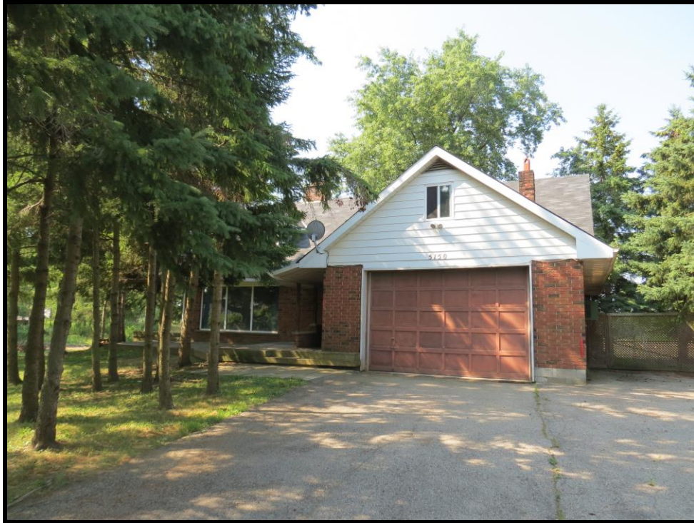
Image 3: Façade of 5150 Ninth Line (Photo taken on July 29, 2019; Facing South)
