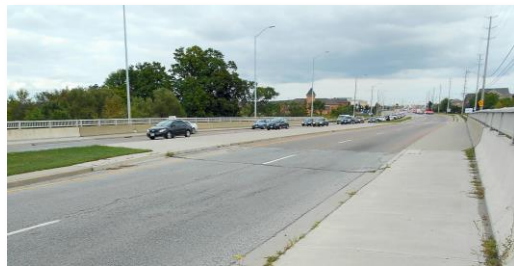
Road cross section will be modified to fit within the existing Fletcher's Creek Bridge
