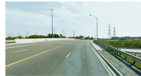
407 bridge widening will be considered to provide for the future cross section
