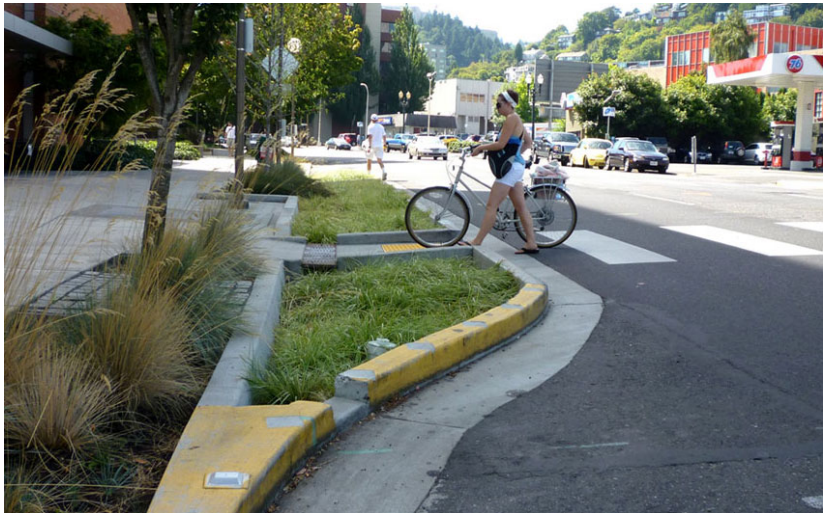
BIORETENTION BUMP-OUTS
