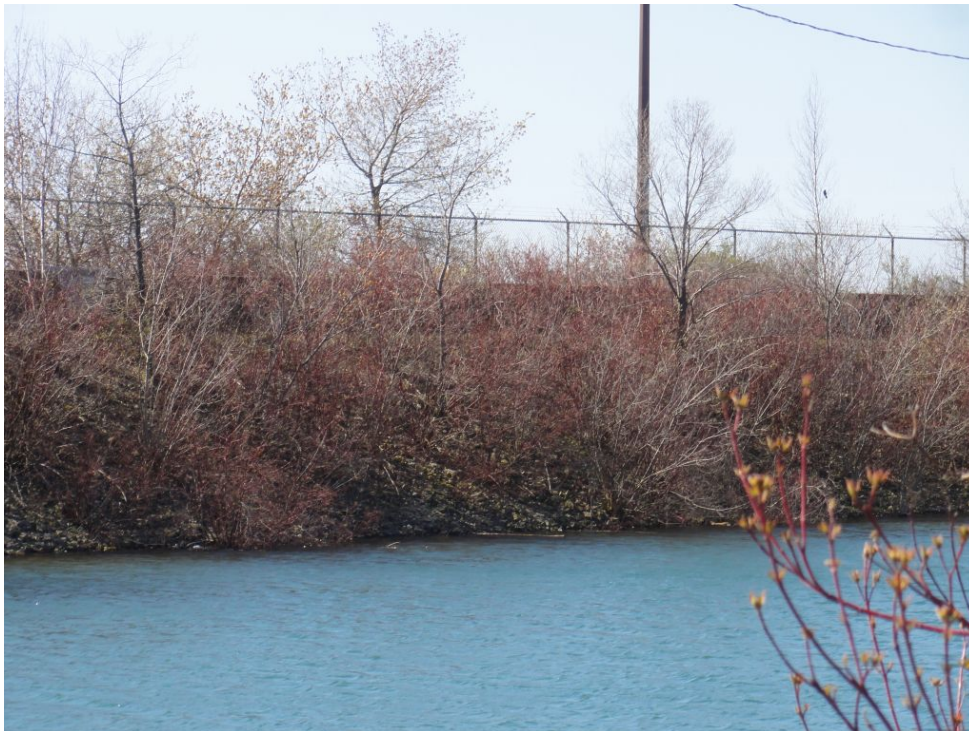
Figure 2.60: Example of riprap slope protection with extensive, established vegetation at Intake Forebay/Channel South
