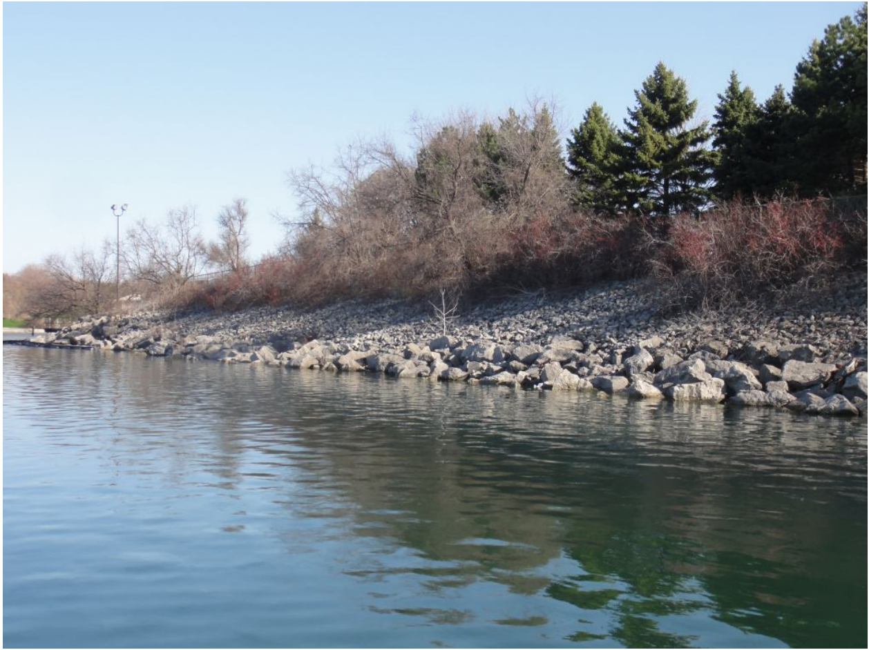
Figure 2.38: View from water of West Shoreline with armour stone at water's edge and riprap up the slope
