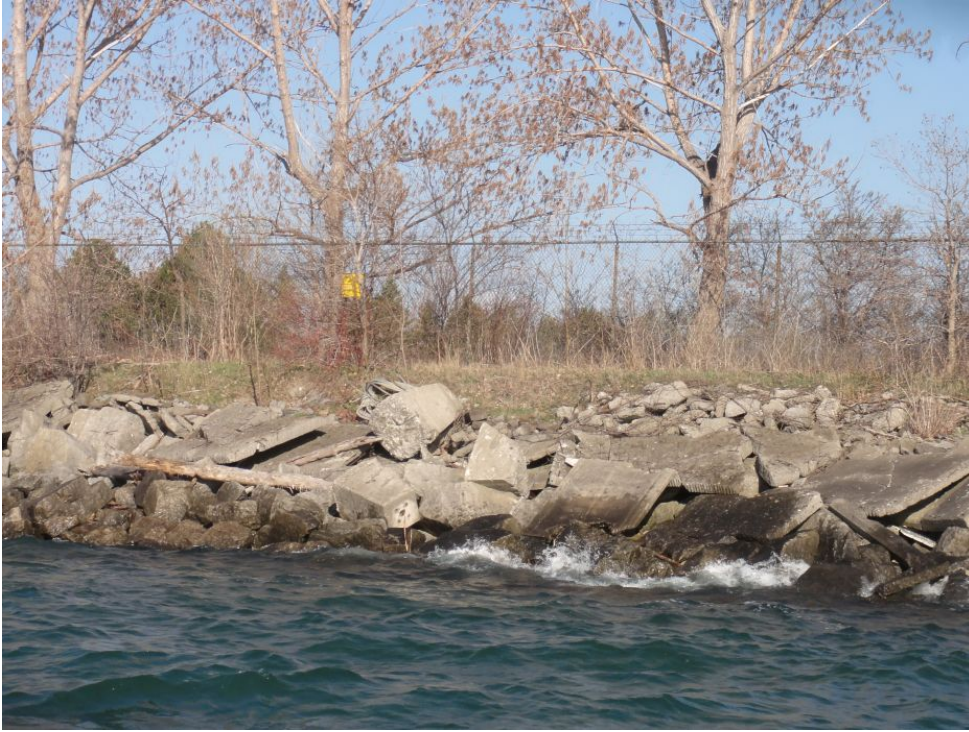
Figure 2.30: Example of concrete rubble slabs on revetment at westerly portion of Outer Shore
