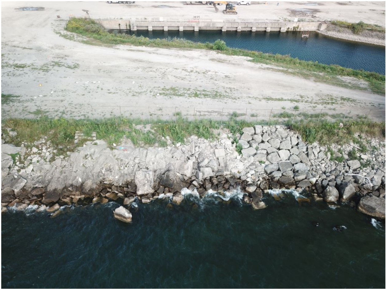
Figure 2.29: Mixture of armouring at westerly portion of Outer Shore (near OS610 to OS640)
