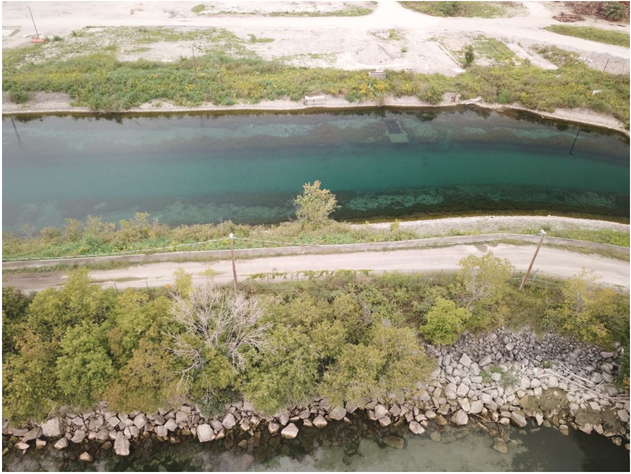
Figure 2.50: Riprap slope protection at east end of Intake Forebay/Channel North (background of photo; Outer Shore in foreground)
