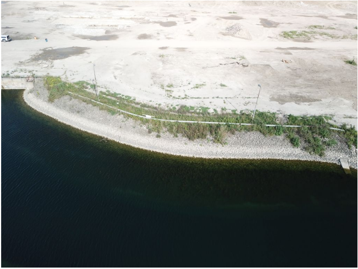
Figure 2.49: Riprap slope protection at west end of Intake Forebay/Channel North (IFN680 to IFN740)
