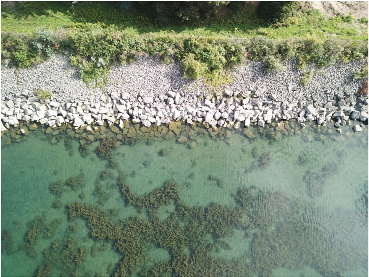
Figure 2.37: West Shoreline armour stone and riprap shore protection
