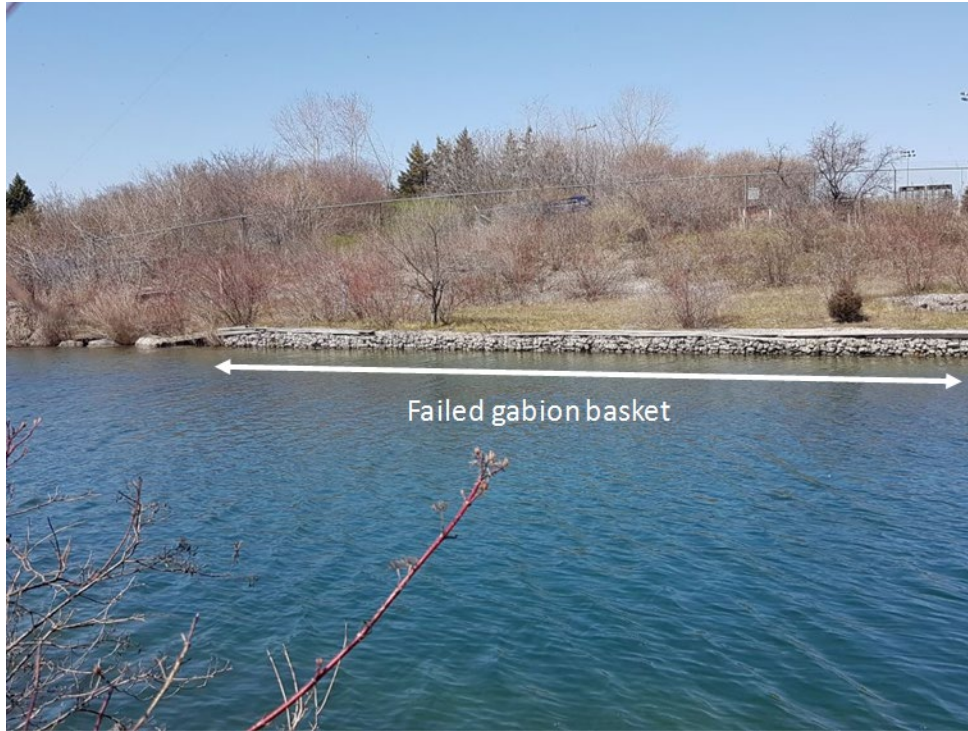
Figure 2.47: Discharge Channel West – failed gabion basket protection and gradual backshore slope
