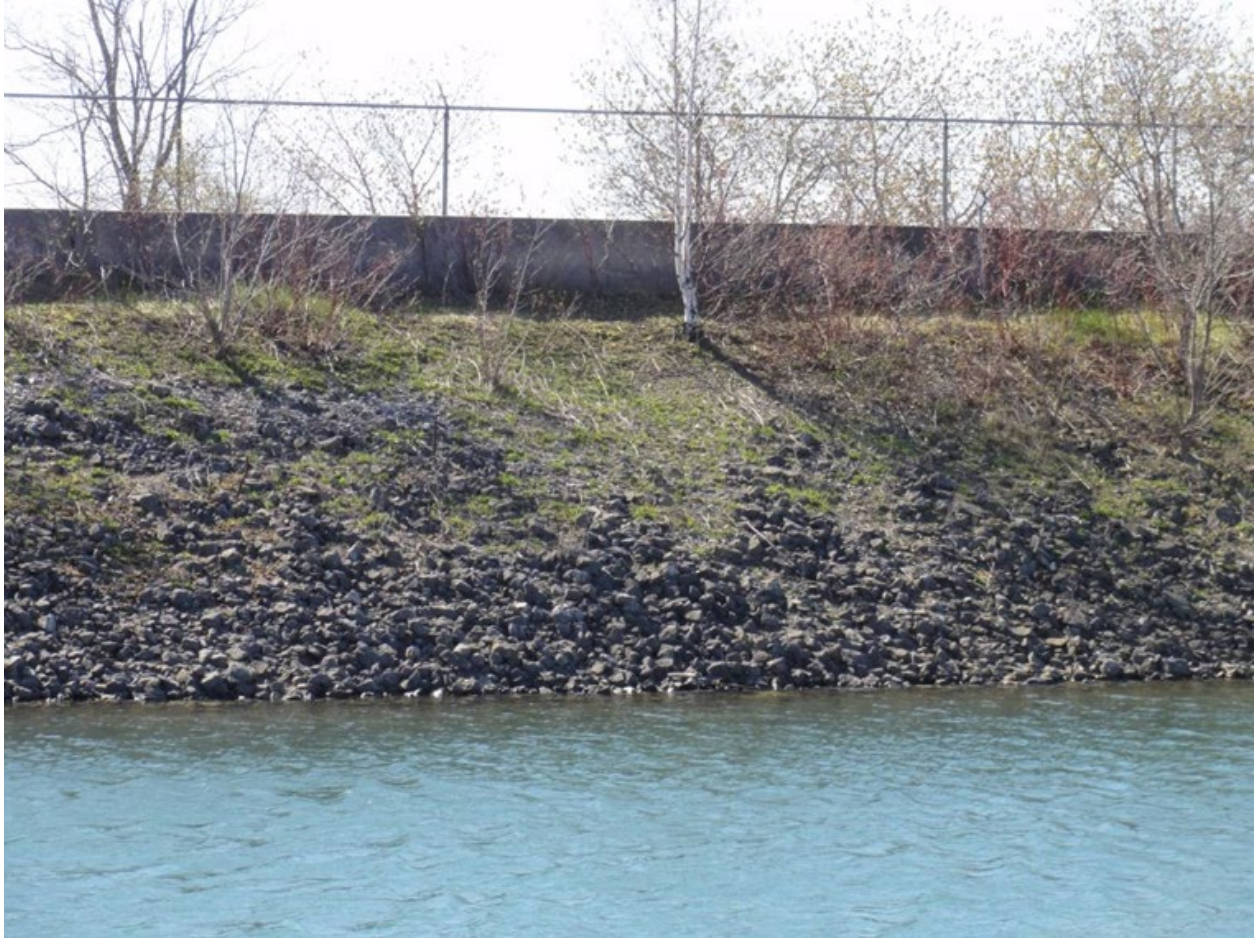
Figure 2.58: Example of riprap slope protection with some vegetation at Intake Forebay/Channel South
