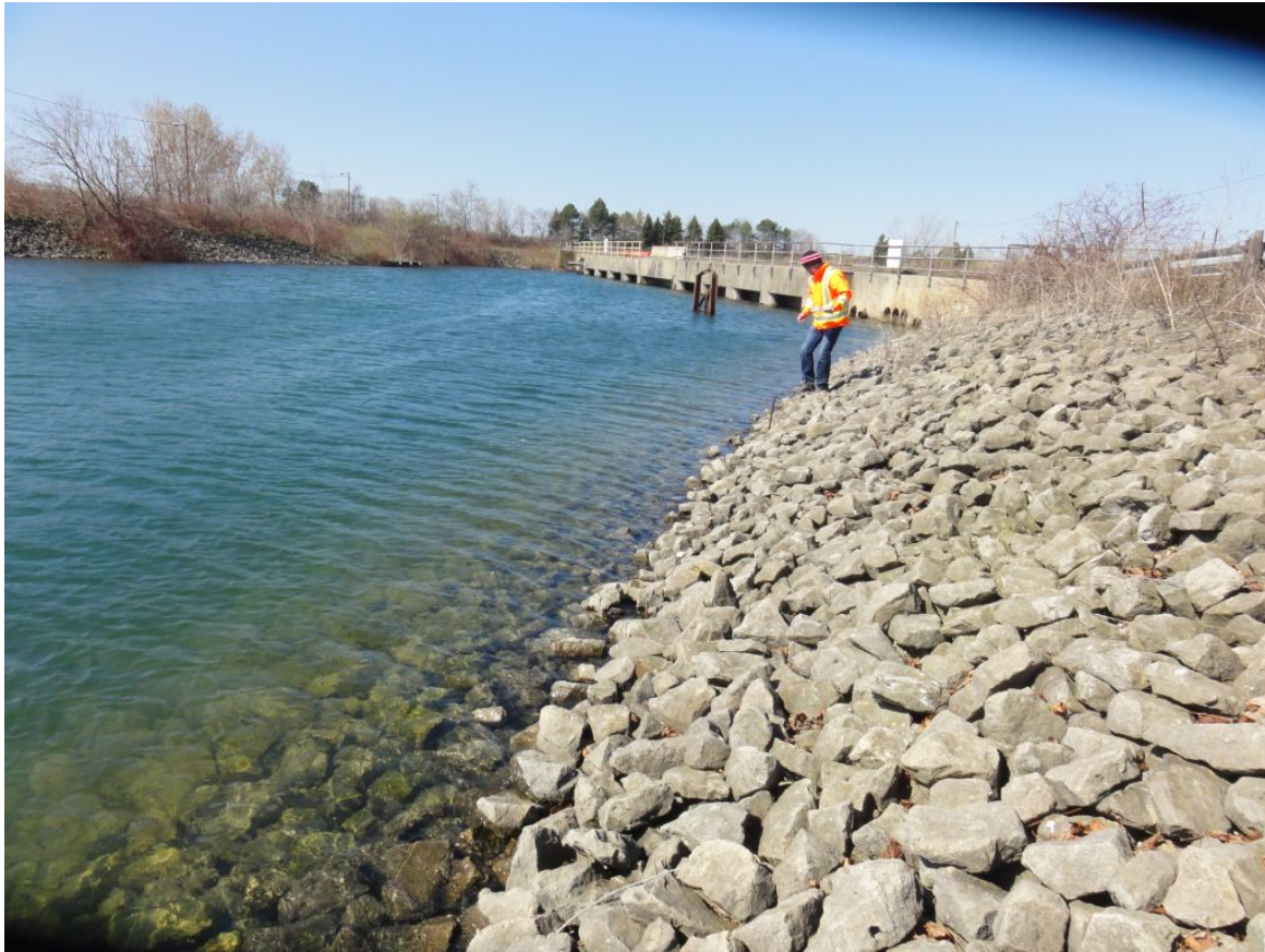
Figure 2.9: Site reconnaissance of riprap slope protection at Intake Forebay/Channel North
