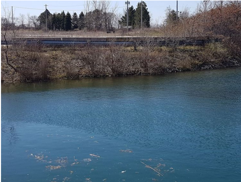
Figure 2.43: Discharge Channel East –riprap with extensive vegetation
