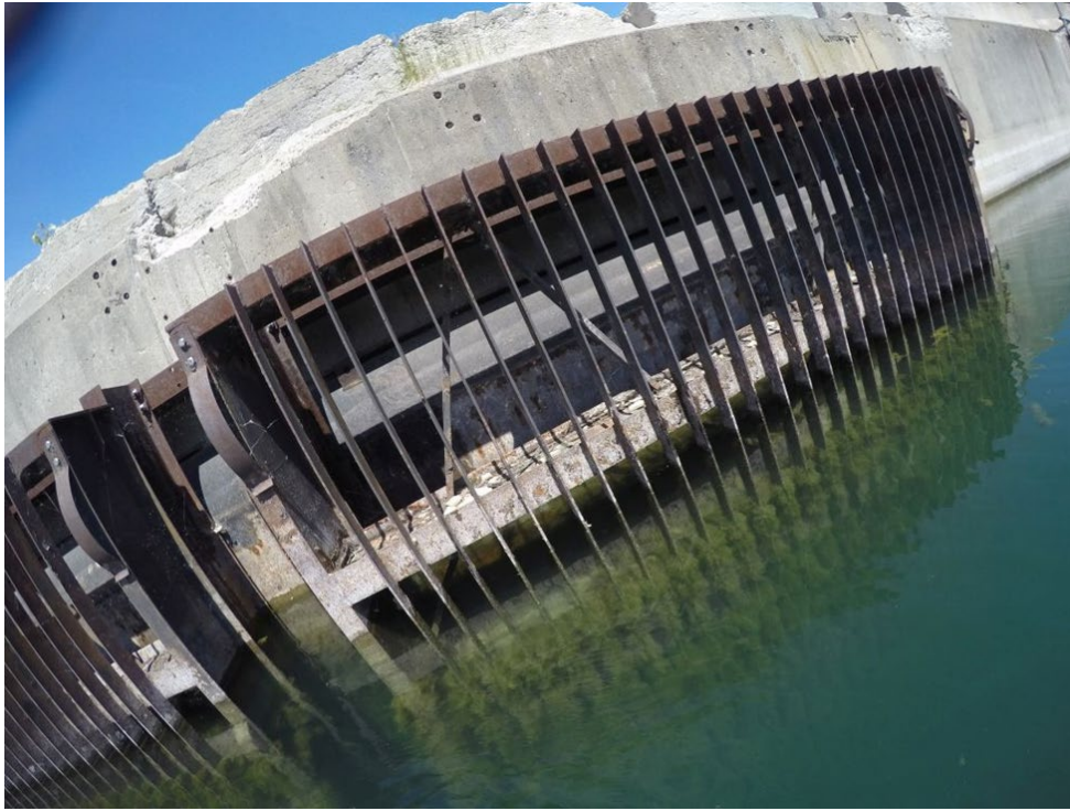
Figure 2.70: View from water of intake grate/screen at Pumphouse 1
