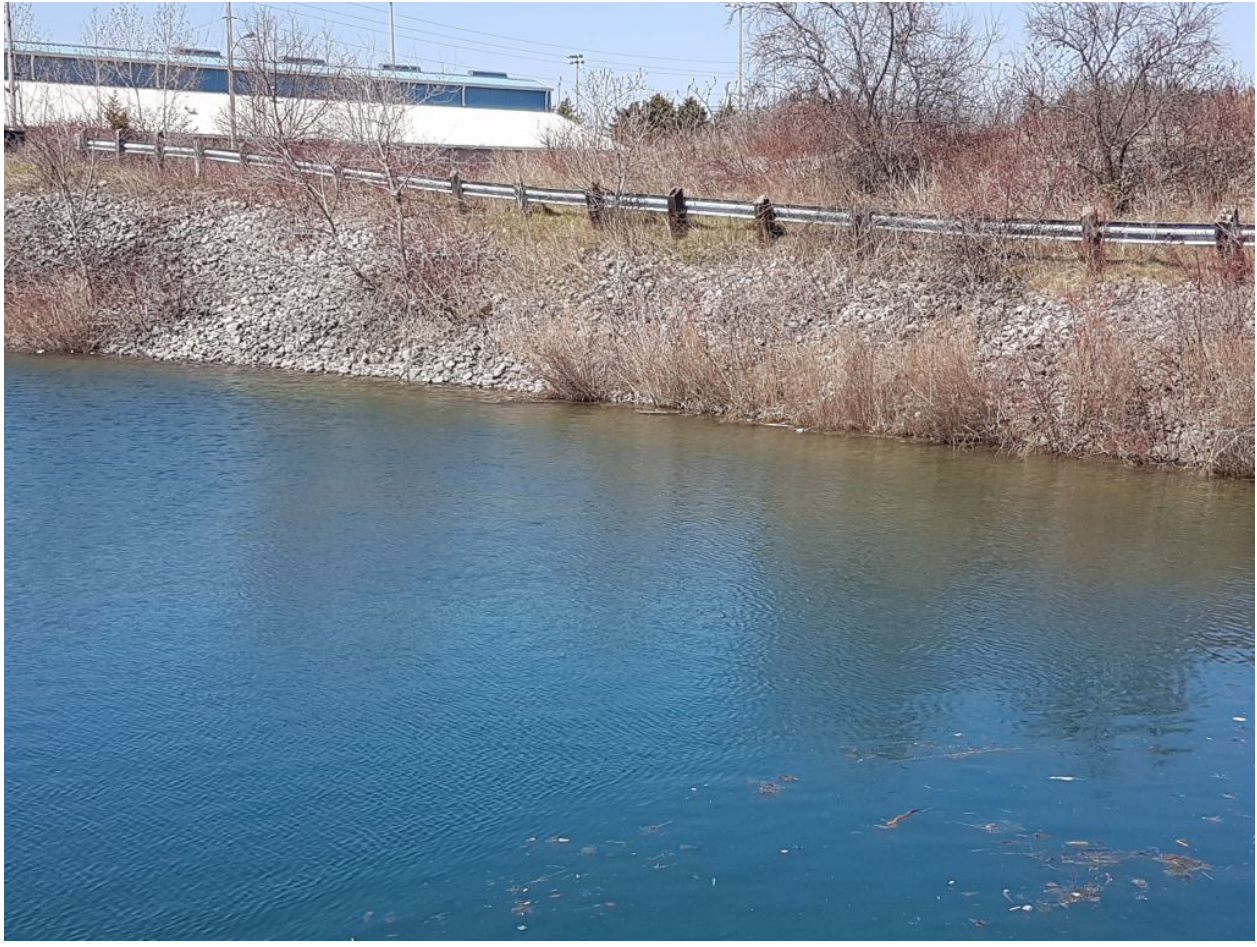
Figure 2.46: Discharge Channel West – vegetated riprap slope
