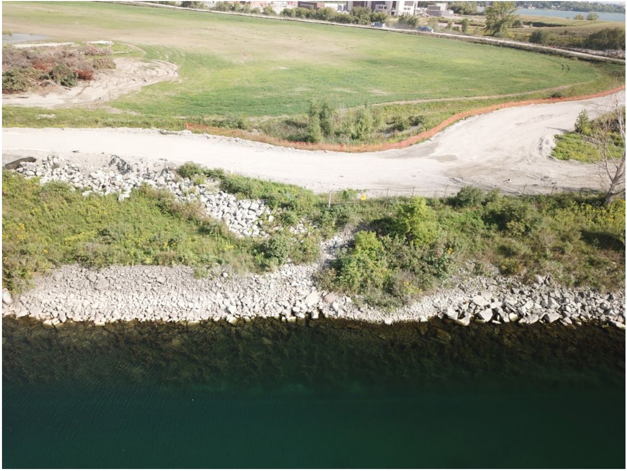
Figure 2.54: Transition of stone size at easterly end of Intake Forebay/Channel North (more sheltered from wave action to the left; less sheltered from wave action to the right)
