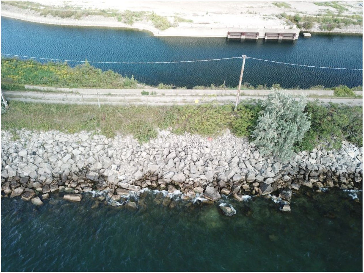
Figure 2.24: Example of stone protection at easterly portion of Outer Shore (this view around OS500)
